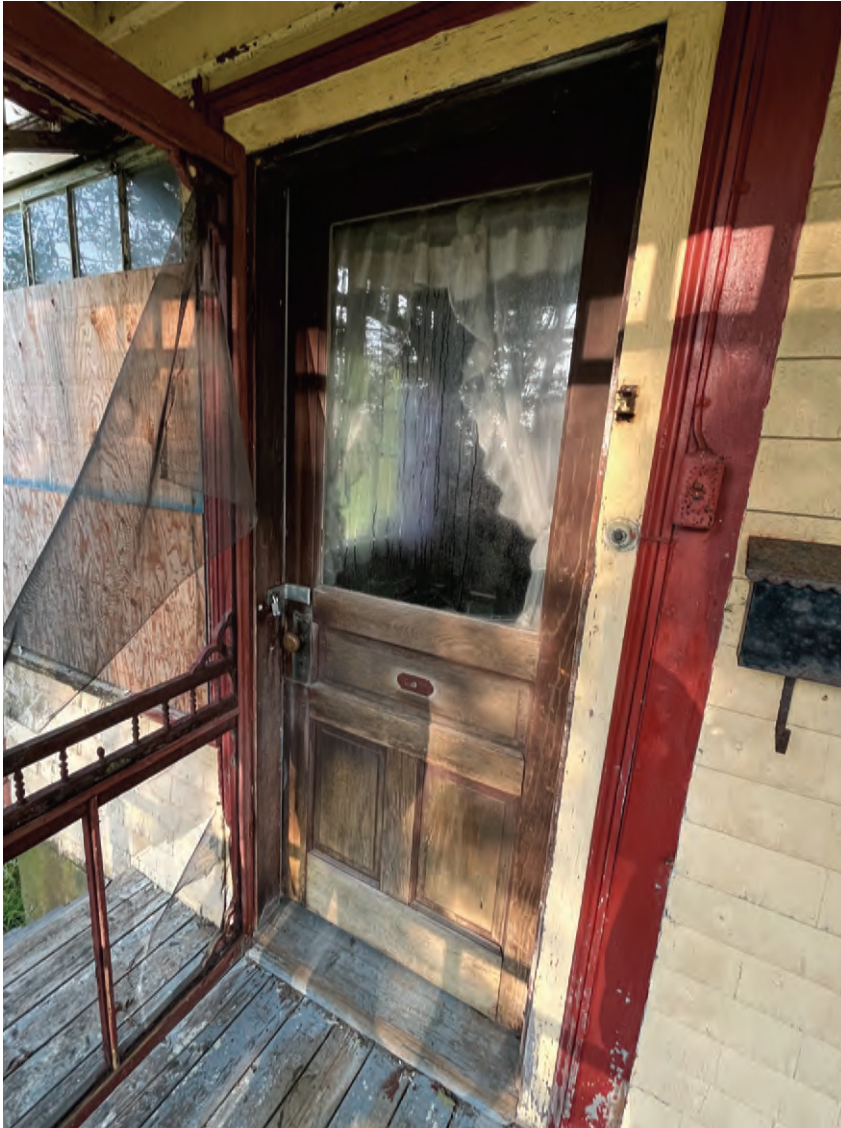
Figure 27: Original wood entry door with inset glazing, relocated to the front face as part of the 1930s alterations.
