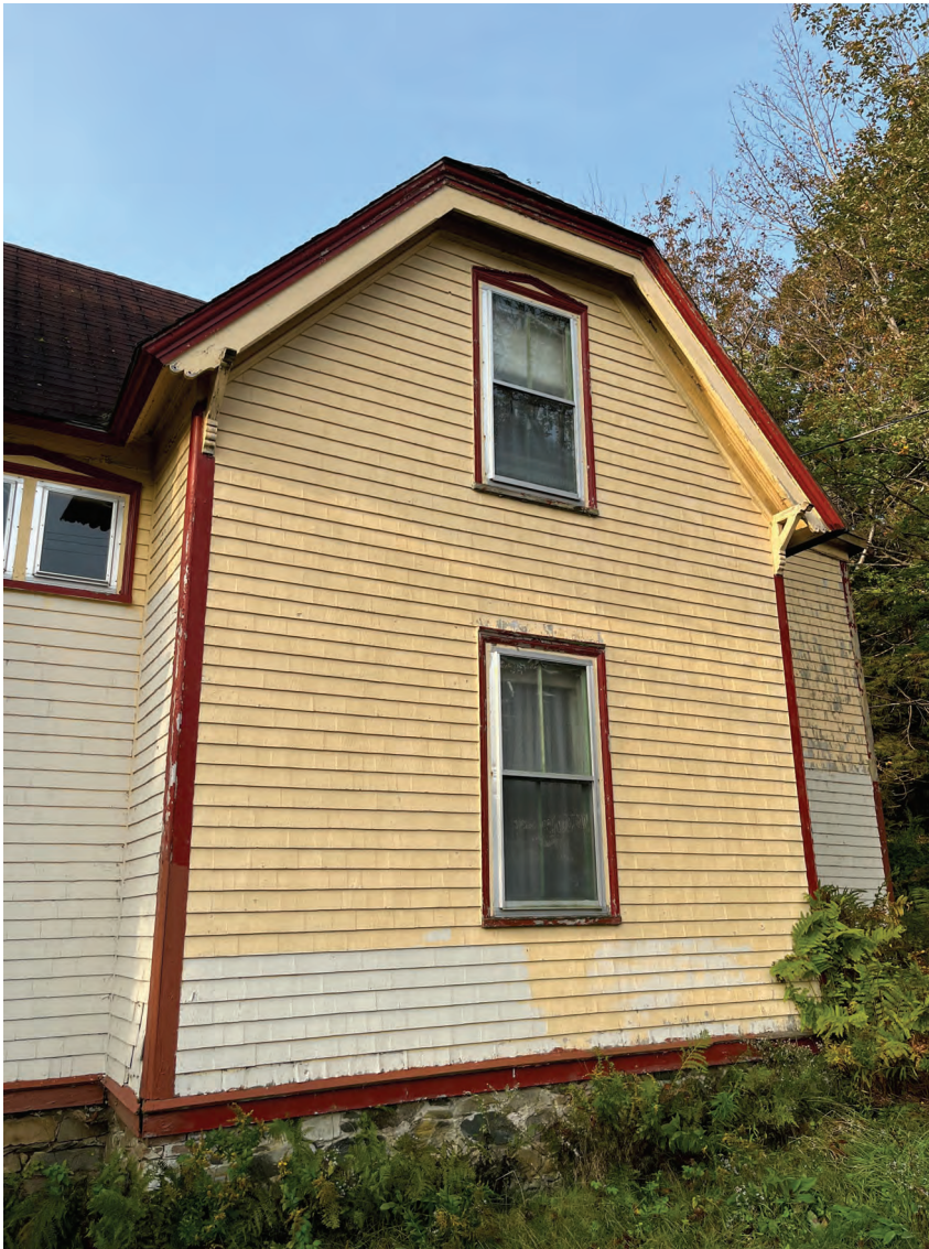
Figure 19: North side addition (1917)
