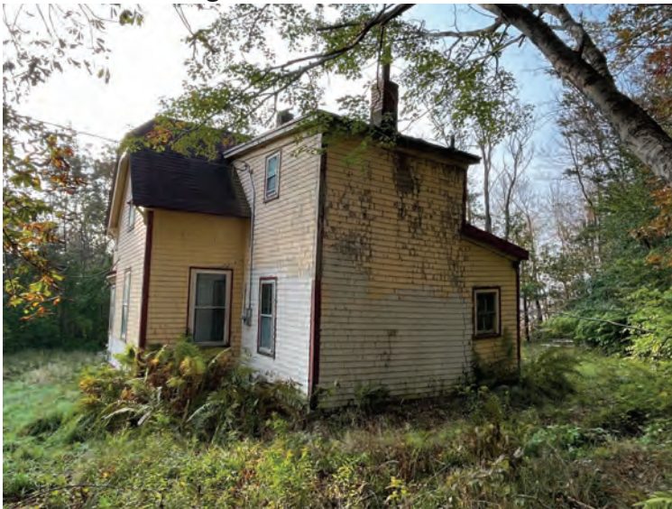
Rear addition protruding out from the 1917 addition.
