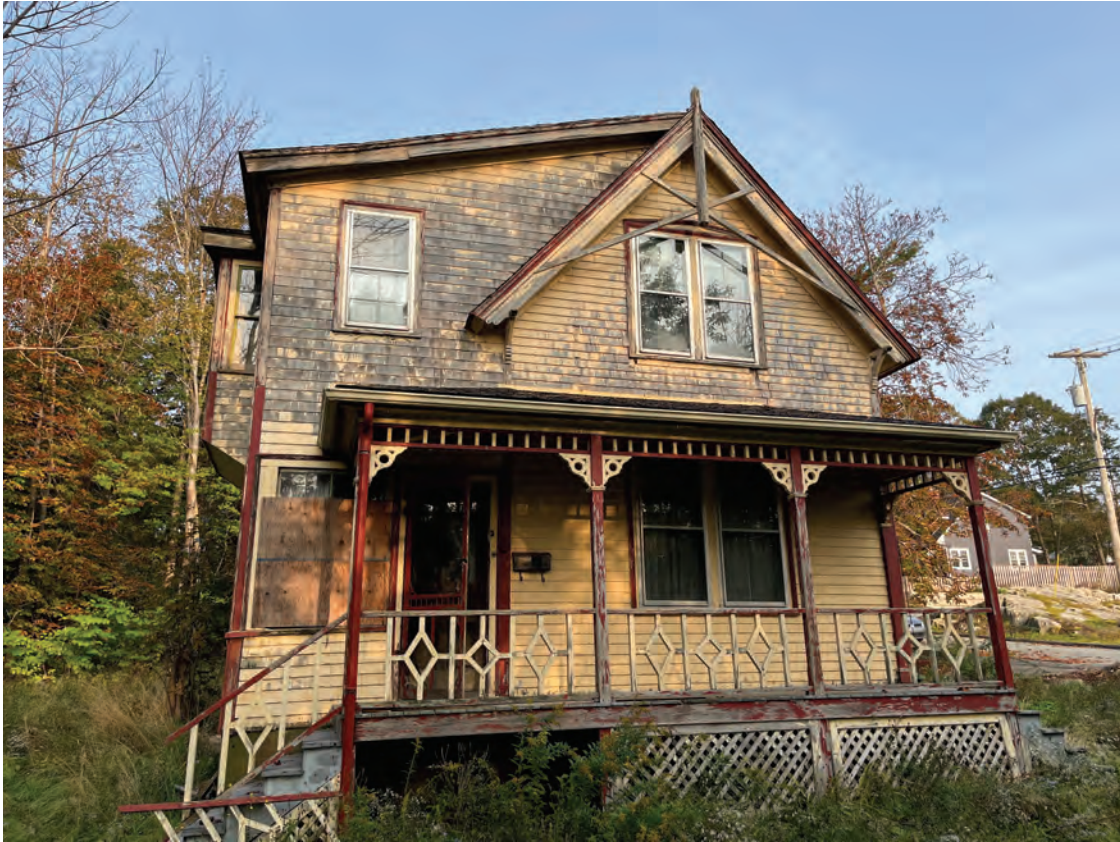
Figure 15: Front of house, east side
