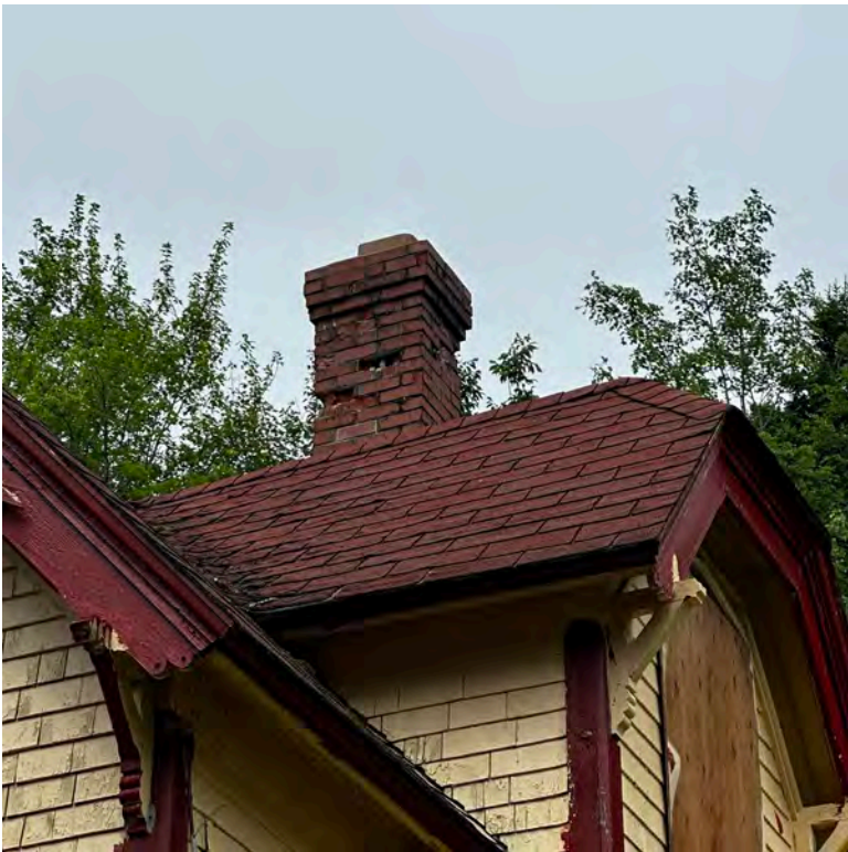
Figure 12: Brick chimney located above the gabled dormer on the north elevation (Staff photo, July 17th, 2024)
