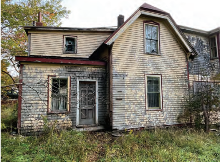
South side additions
