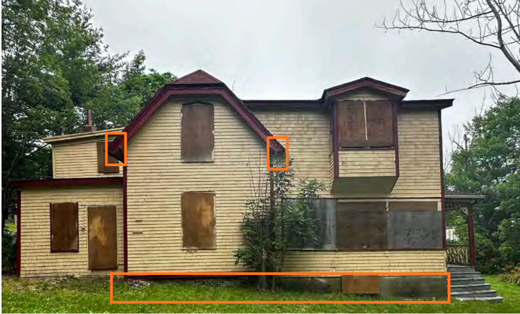
Figure 10: Red Gables from south elevation with the foundation outlined in blue and consistent brackets outlined in orange (Staff photo, July 17th, 2024)
