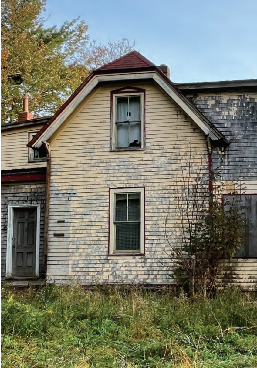
Figure 20: South side addition (1917)
