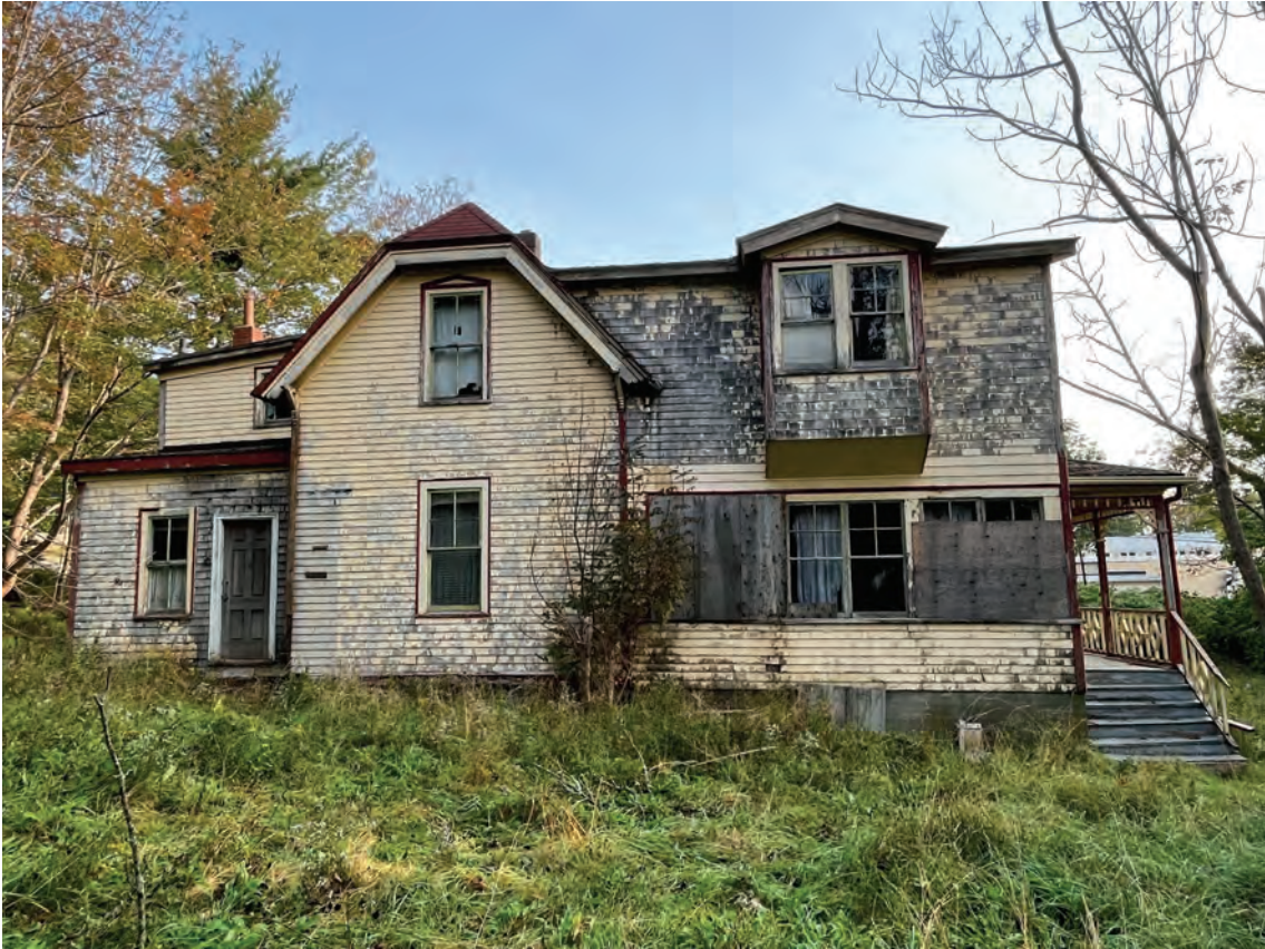
Figure 17: South side of house
