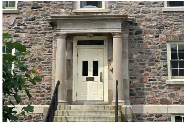
Photo 12: Secondary entrance, looking west
