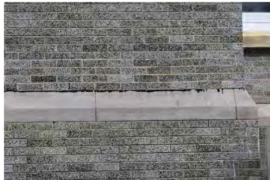
Photo 21: Belt-course, looking north
