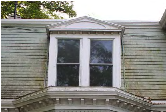
Photo 4: Gable dormer, looking south
