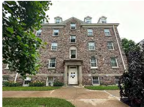
Photo 37: Representative bay, looking south (HRM 2023b)
