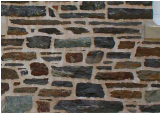
Photo 3: Stone clad exterior, looking south
