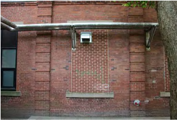
Photo 14: Bricked in window opening, looking south
