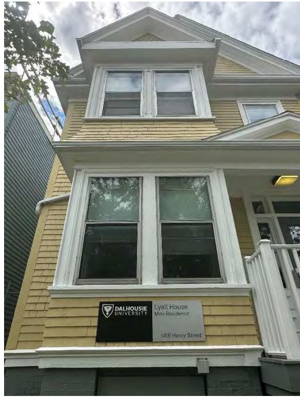
Photo 6: Projecting gable bay, looking west (HRM 2023b)
