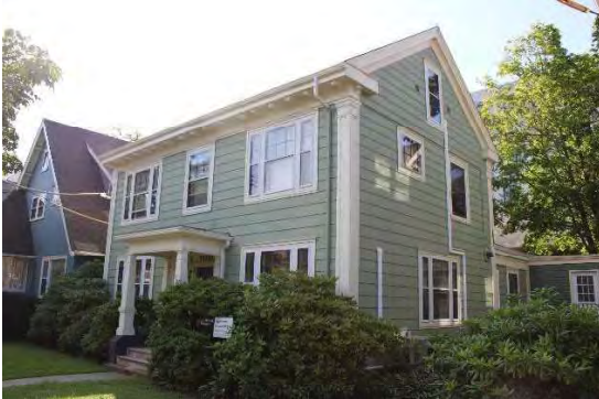
Photo 1: Two-and-one-half storey height, looking southeast
