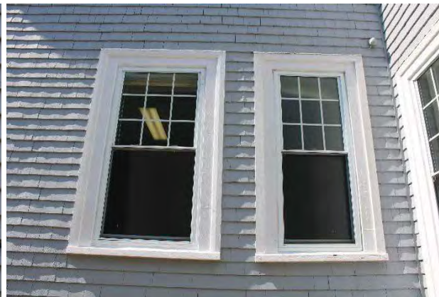
Photo 6: Replacement windows and wood surrounds
