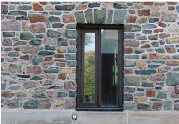
Photo 10: Representative window opening with stone voussoir, looking west
