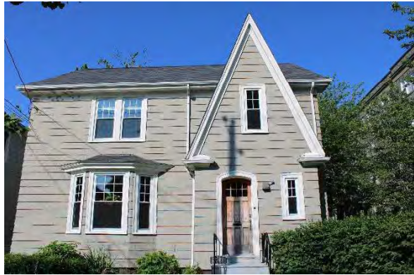
Photo 18: Asymmetrical front façade, looking west
