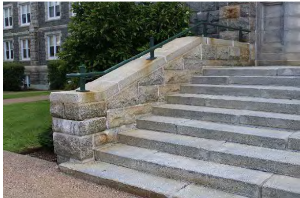
Photo 11: Stone staircase details, looking northeast
