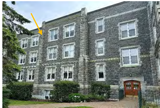
Photo 3: Representative pilaster, denoted by arrow, looking east (HRM 2023)
