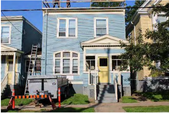
Photo 13: Front façade, looking west
