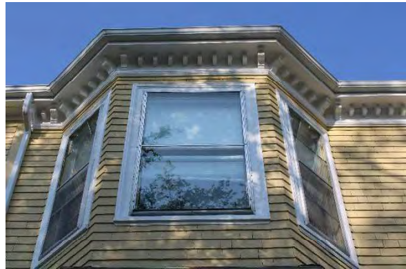
Photo 16: Wood sash windows, looking west
