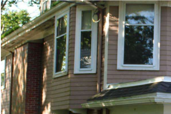
Photo 11: Bay window on second storey of east façade, looking southeast
