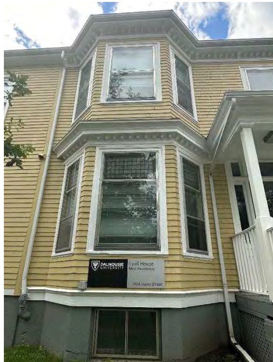
Photo 14: Projecting bay, looking west (HRM 2023b)
