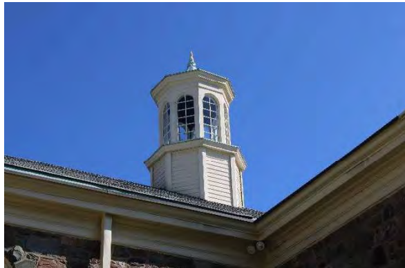
Photo 26: Cupola, looking north
