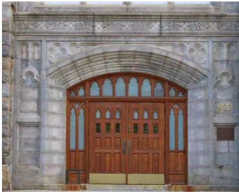
Photo 10: Main entrance, looking east
