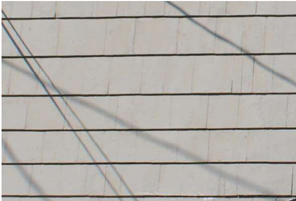
Photo 17: Wood clad exterior, looking west
