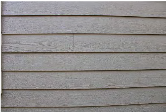
Photo 11: Wood siding, representative view
