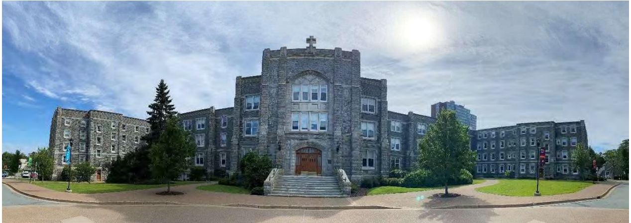
Photo 1: General view showing three storey structure and wings, looking east
