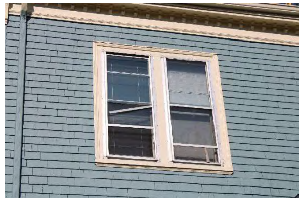
Photo 18: Representative wood sash window, looking west
