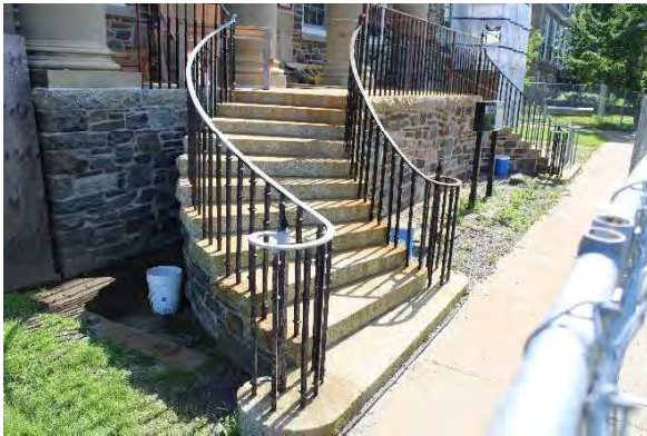
Photo 9: Curved staircase, looking southwest
