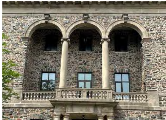
Photo 7: Balcony, looking west
