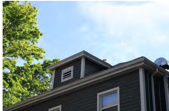
Photo 4: Hip dormer on the rear (west) façade, looking northeast
