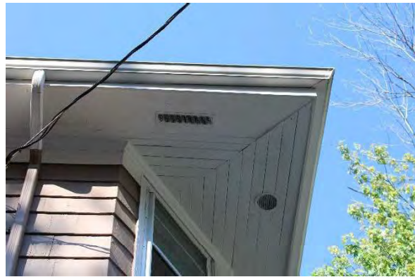
Photo 14: Wood soffits and fascia, looking west
