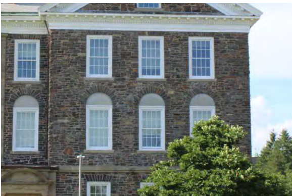
Photo 7: Representative window openings, looking north
