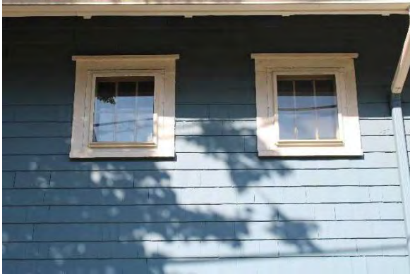
Photo 7: Representative square window openings, looking south
