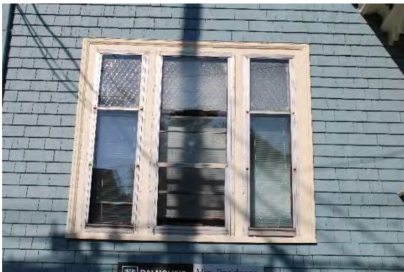
Photo 9: Representative wood sash window, looking west
