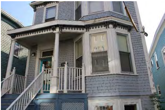
Photo 3: Two storey bay window
