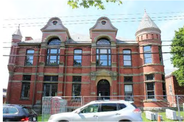
Photo 14: General view of front (northeast) façade showing asymmetrical design, looking southwest
