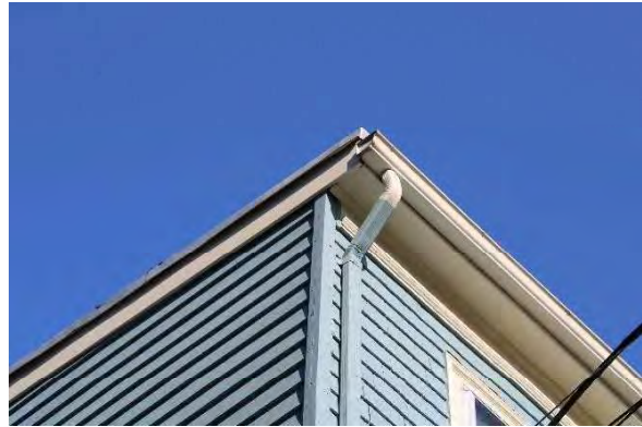
Photo 6: Fascia and soffit, looking north
