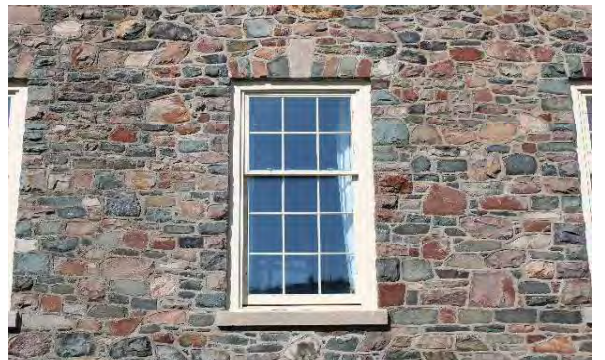
Photo 6: Representative rectangular window opening, looking west
