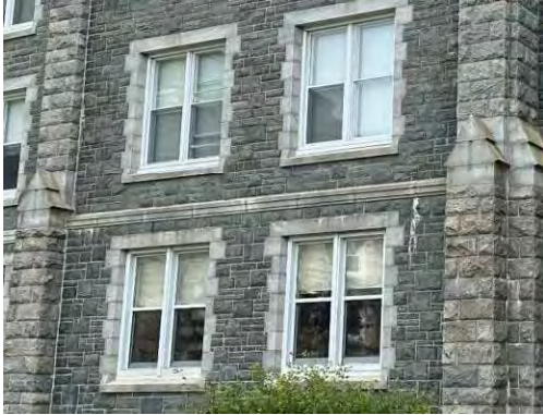
Photo 6: Square window openings, looking east (HRM 2023b)
