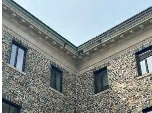
Photo 5: Frieze, brackets, and cornice, looking south
