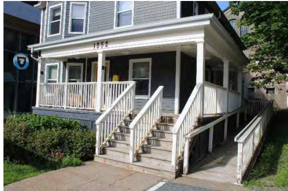
Photo 6: Wrap-around porch, looking southwest
