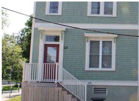
Photo 6: Front entrance pilasters
