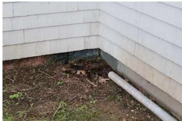
Photo 13: Wood shingle cladding and parged and poured concrete foundation, looking northeast
