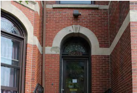
Photo 10: Stained-glass fan light above front entrance, looking north
