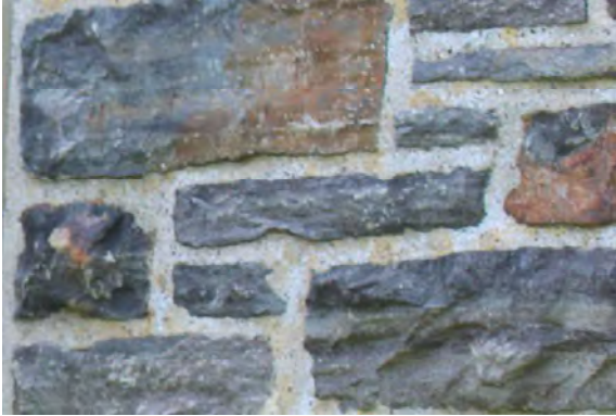
Photo 3: Stone exterior, looking north
