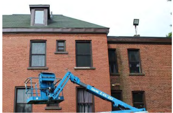
Photo 15: Brick voussoirs and stone sills on side façade, looking west
