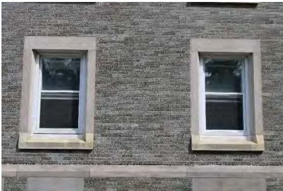
Photo 22: Rectangular window openings, looking north
