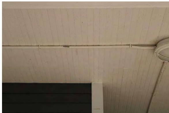
Photo 8: Wooden ceiling of porch, looking west
