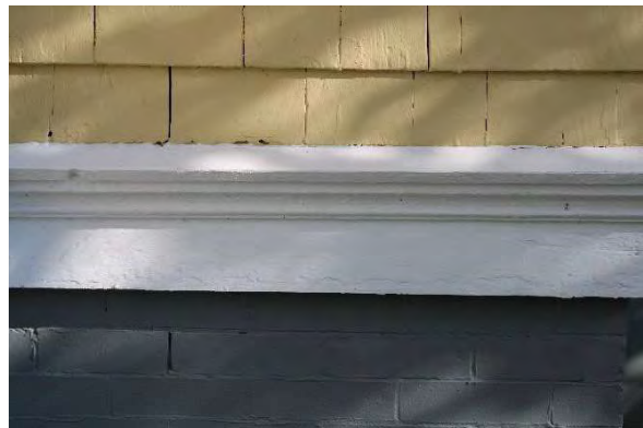
Photo 4: Shingle and belt course details, looking west
