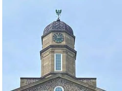
Photo 2: Cupola, looking west
