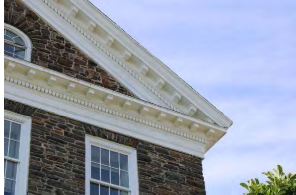
Photo 4: Representative pediment and cornice details, looking west
