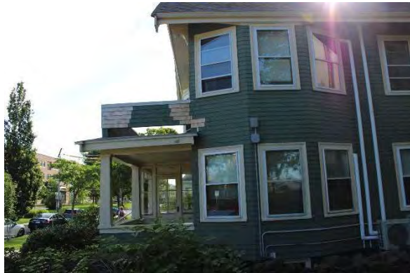
Photo 9: Full height bay, looking east
