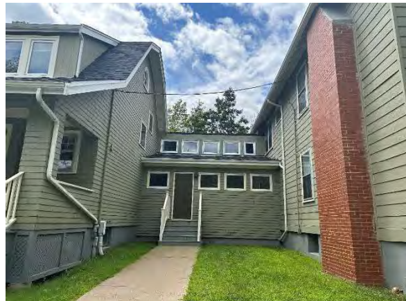
Photo 15: Connecting addition, looking west (HRM 2023b)
