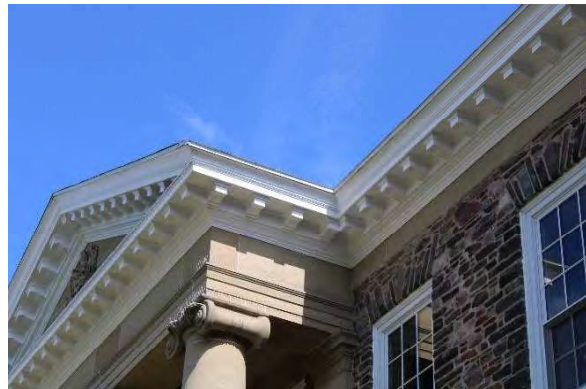
Photo 2: Representative bracketed cornice and pediment, looking southeast
