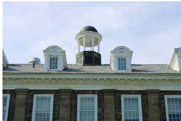
Photo 2: Representative photo of dormers and view of cupola, looking north
