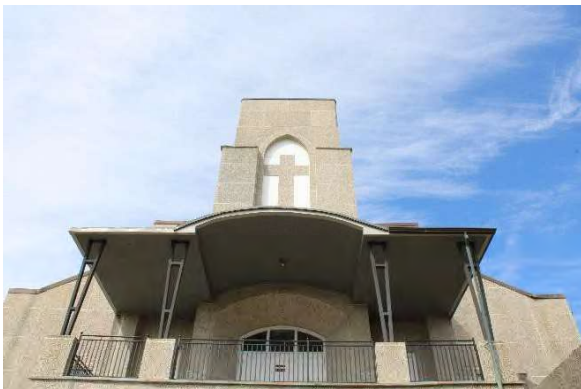
Photo 28: Balcony, looking west
