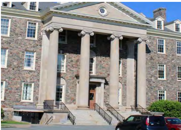
Photo 9: Columns, looking northwest
