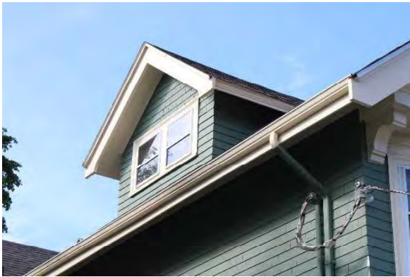
Photo 3: Representative dormer, looking west
