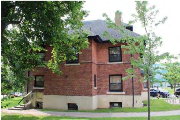
Photo 7: Projecting bay on the north façade, looking south
