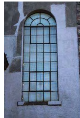
Photo 6: Representative arched window, looking west
