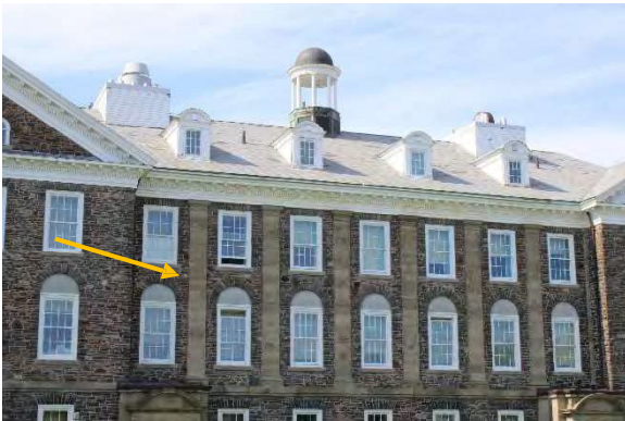
Photo 5: Stone pilasters, denoted by arrow, looking north
