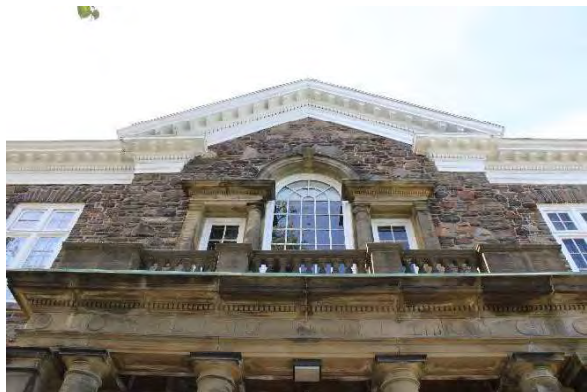
Photo 15: Second storey windows, looking north
