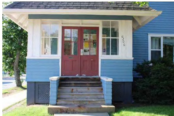
Photo 6: Partial width enclosed front porch, looking south
