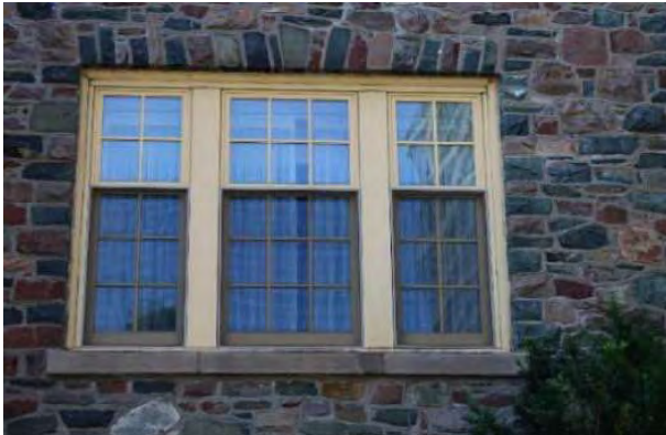
Photo 21: Representative window opening, looking south
