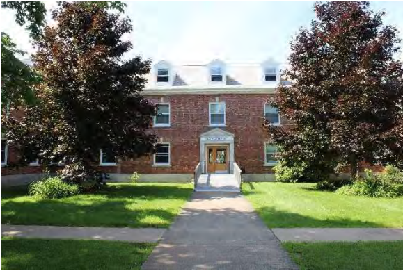
Photo 2: General view of the front (northeast) façade showing the two and one half storey massing and gable roof dormers, looking southwest
