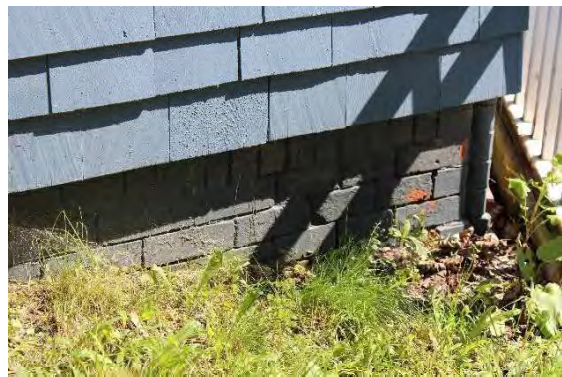
Photo 12: Brickwork under shingles
