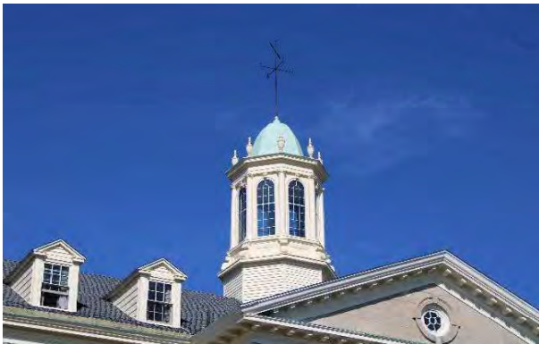
Photo 3: Cupola, looking west
