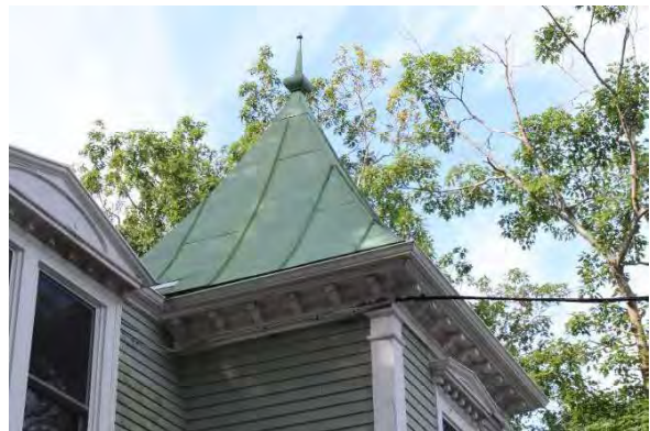
Photo 5: Copper roof, finial, and brackets on projecting central frontispiece, looking southwest
