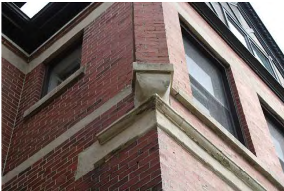
Photo 6: Stone corbel and belt courses, looking northeast
