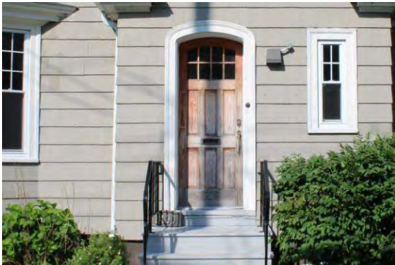
Photo 19: Main entrance, looking west
