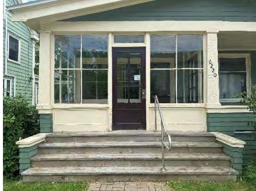
Photo 7: Enclosed part of front porch, looking south (HRM 2023b)
