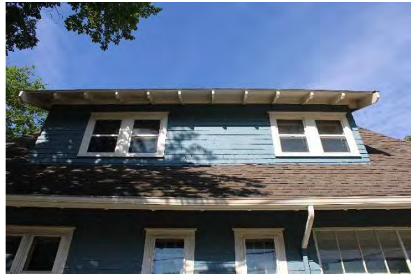
Photo 4: Representative dormer details, looking west
