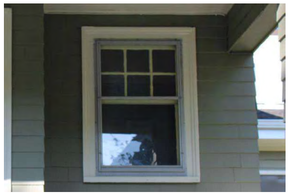
Photo 5: Wood sash window, looking west
