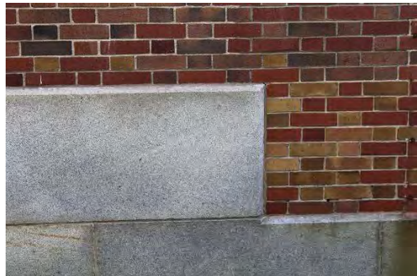
Photo 13: Cut stone or stone clad foundation, looking southeast
