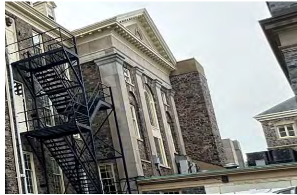
Photo 14: Rear façade pediment, looking south (HRM 2023b)
