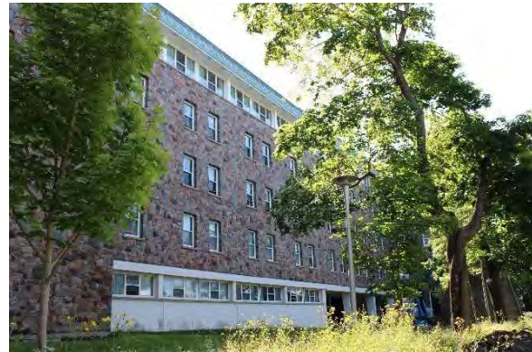
Photo 2: Shirreff Hall five storey section, built 1967, looking east
