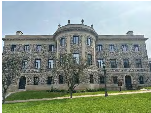
Photo 11: Rear façade showing apse and arched secondary entrances, looking east
