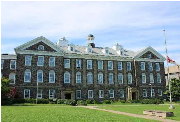
Photo 1: Science Building showing general plan, looking north
