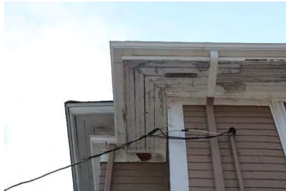
Photo 2: Wood fascia and soffits, looking east
