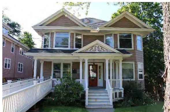
Photo 18: Front façade, looking south
