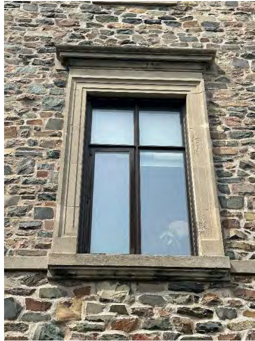
Photo 9: Representative window opening with stone surround, looking west
