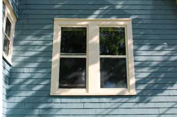
Photo 8: Representative rectangular window openings, looking south
