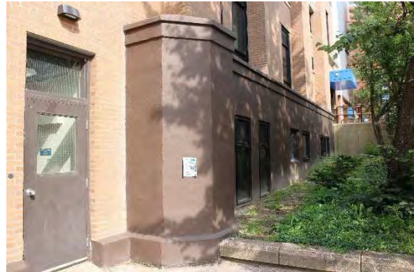
Photo 8: Concrete foundation on the east façade, looking northeast
