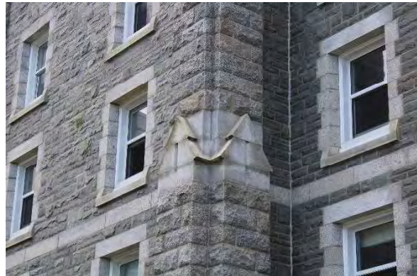
Photo 15: Representative pilaster and belt-course details, looking south
