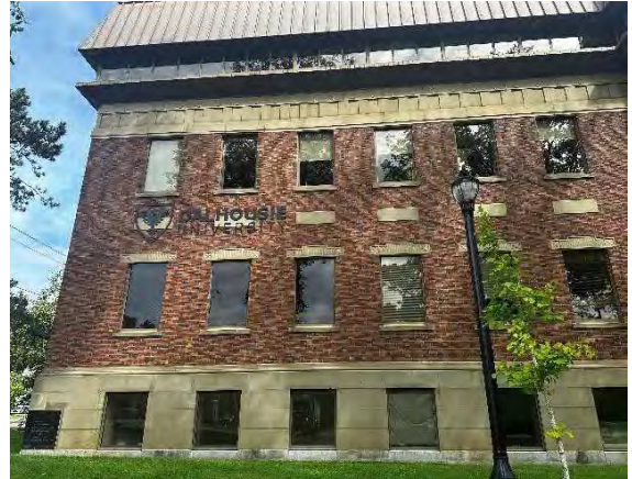
Photo 6: Window openings, looking north
