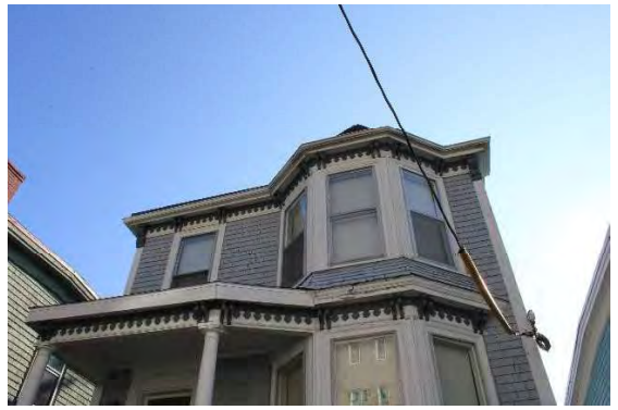
Photo 4: Two storey bay window
