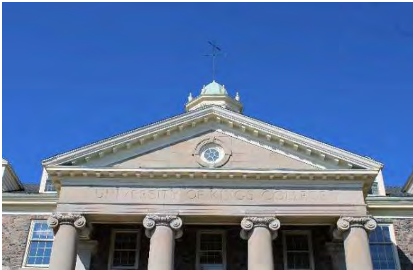
Photo 7: Pediment, looking west
