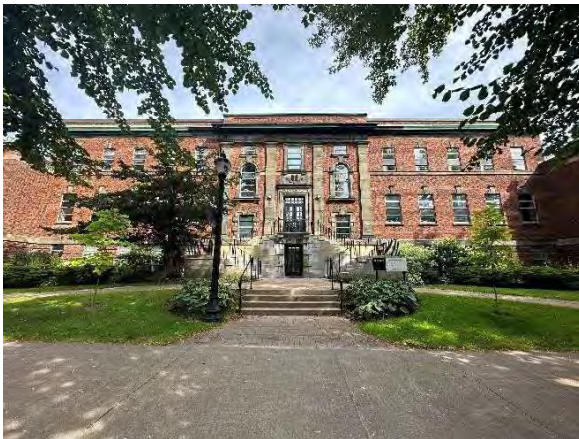
Photo 1: Public Health Clinic, looking north
