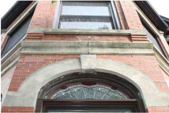
Photo 8: Stone belt courses, window heads and keystones, looking north
