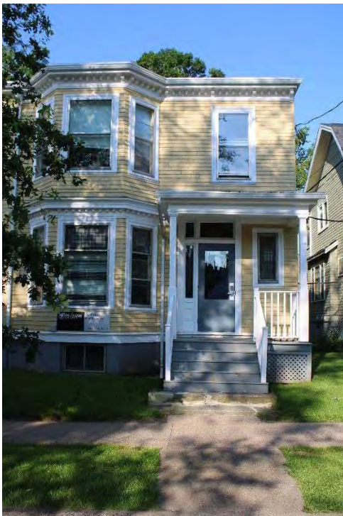
Photo 13: Front façade, looking west
