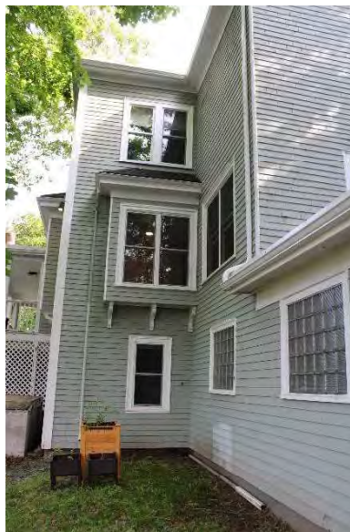
Photo 1: Glass block windows and poured concrete foundation in the Stairs House rear addition
