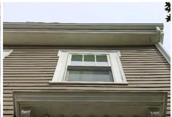
Photo 7: Classically inspired window details including wooden surrounds on upper storey windows and wide eaves with wooden soffits, looking north
