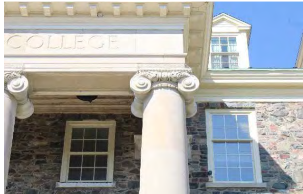
Photo 8: Representative column details, looking west (HRM 2023b)
