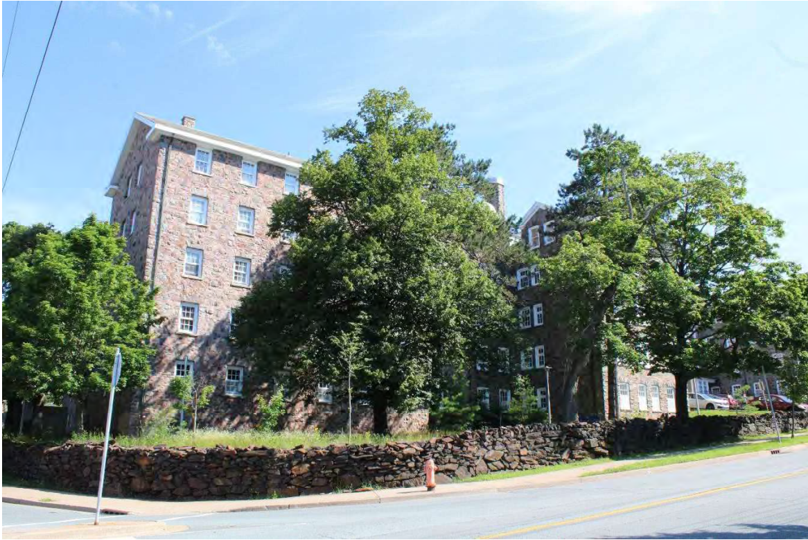
Photo 14: Dry stack stone wall and Shirreff Hall, looking north
