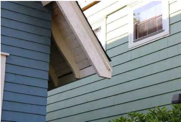
Photo 3: Fascia, soffit, and rafter detailing, looking west
