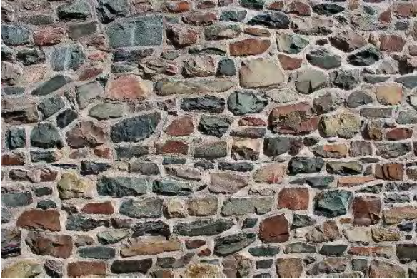
Photo 4: Stone cladding, looking west
