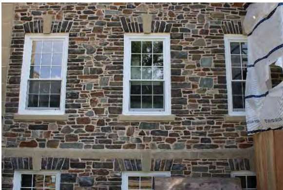
Photo 7: Representative window openings, looking south
