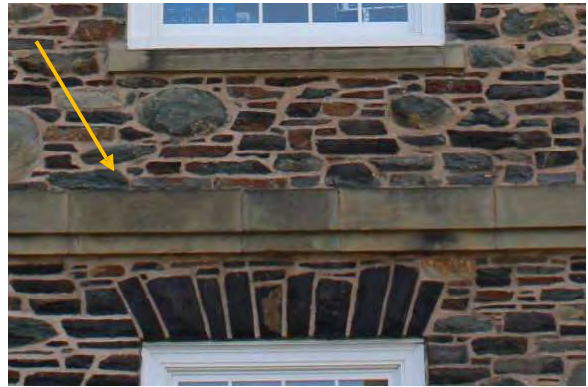
Photo 6: Belt course, denoted by arrow, looking west
