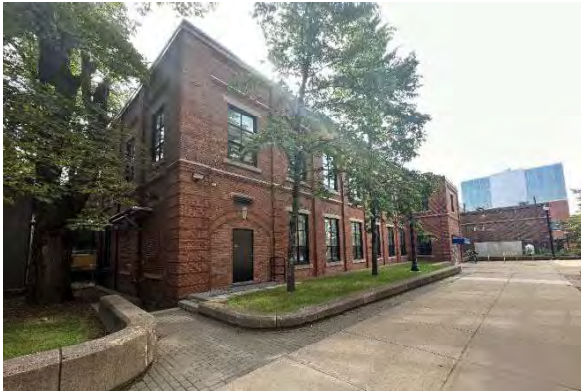
Photo 5: 5273 Dacosta Row, looking southeast
