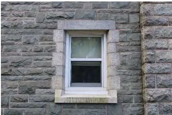
Photo 16: Representative window opening, looking south
