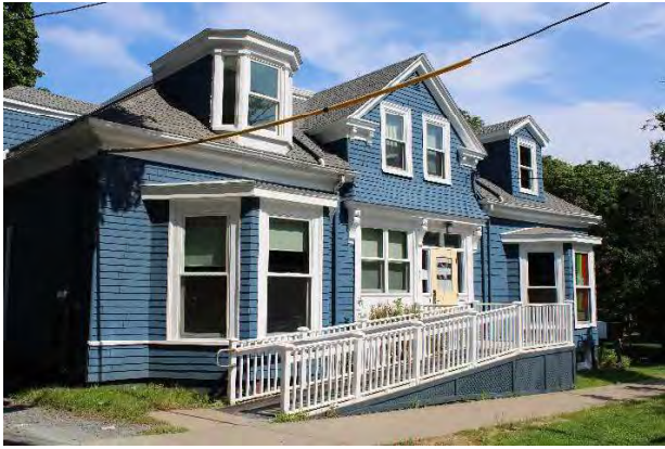
Photo 1: 1321 Edward Street looking east, with Scottish dormer
