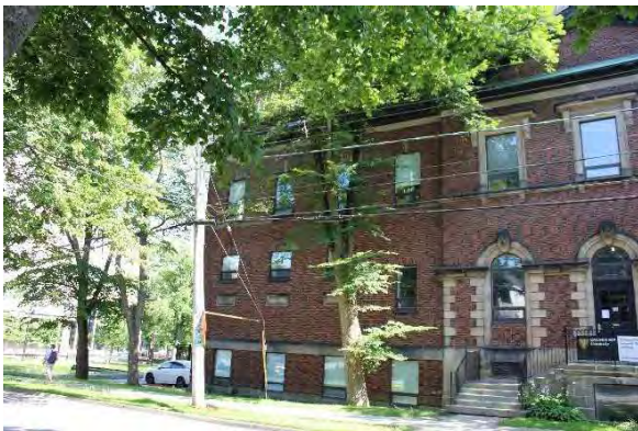
Photo 12: East half of building, looking south
