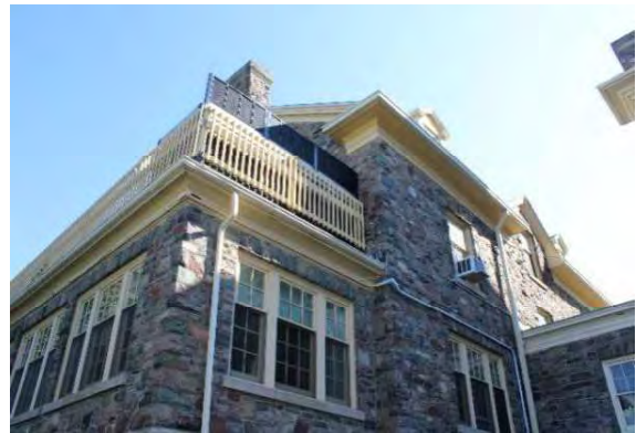
Photo 24: Balcony, looking north
