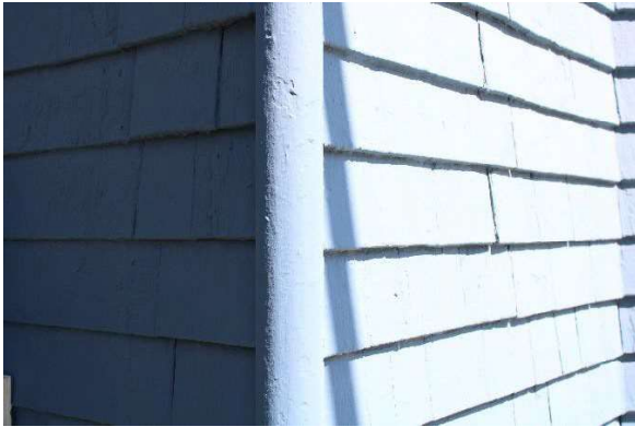
Photo 7: Painted shingle exterior
