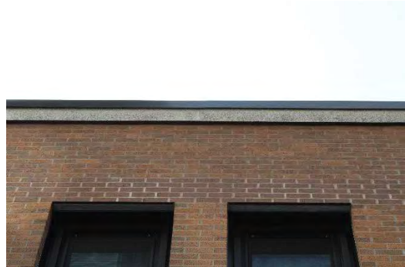
Photo 2: Flat roof and pebble dash cornice, looking south
