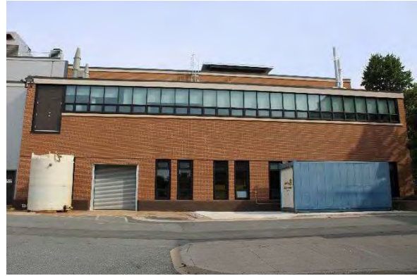
Photo 6: Ribbon window on the south façade, looking north
