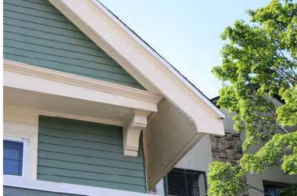
Photo 2: Soffit and fascia details, looking south
