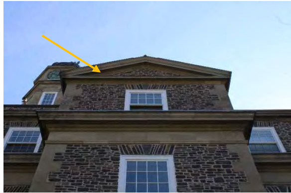
Photo 4: Representative cornice, denoted by arrow
