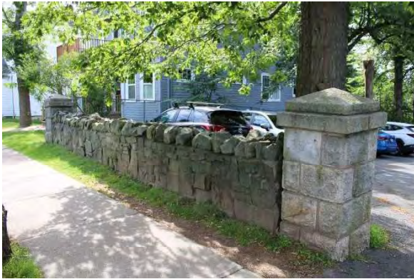
Photo 18: Stone fence and pillar along front of property, looking southeast
