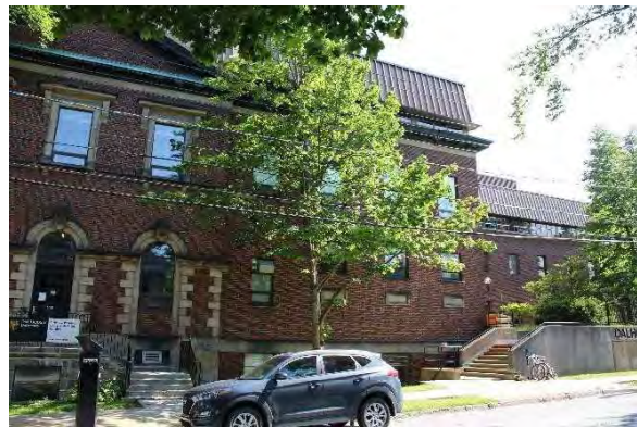
Photo 13: West half of building, looking south
