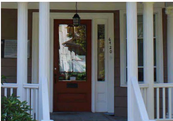
Photo 22: Main entrance, looking south
