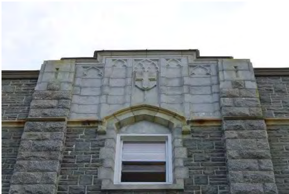
Photo 14: Stone cross and tracery, looking east
