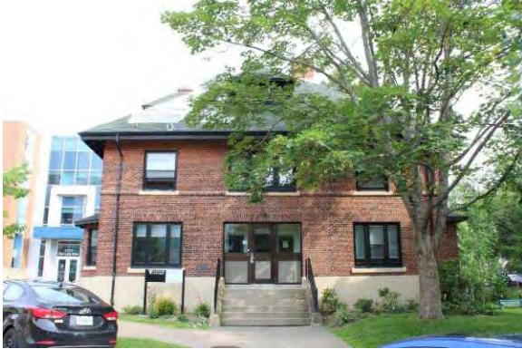
Photo 1: Sexton House showing two- and one-half storey structure, looking north
