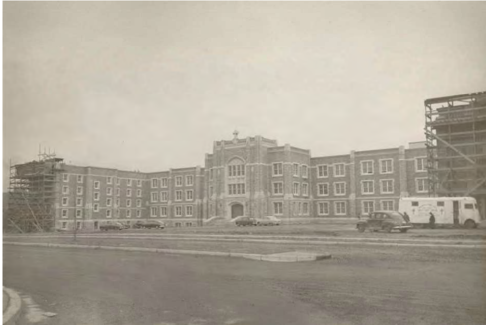
Plate 3: Construction nearly completed in 1951 (SMU Archives 1951)
