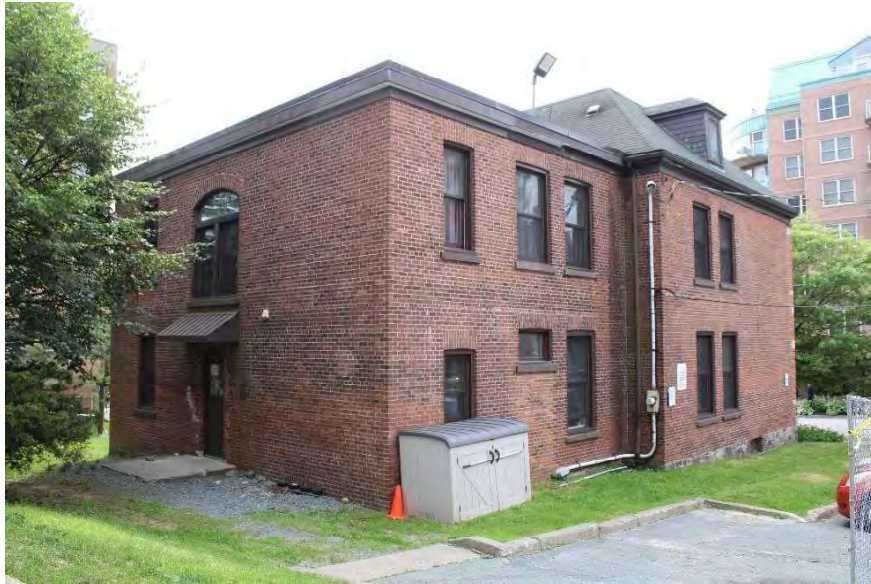
Photo 3: Rear wing and west façade with common bond brick pattern and stone foundation, looking southeast
