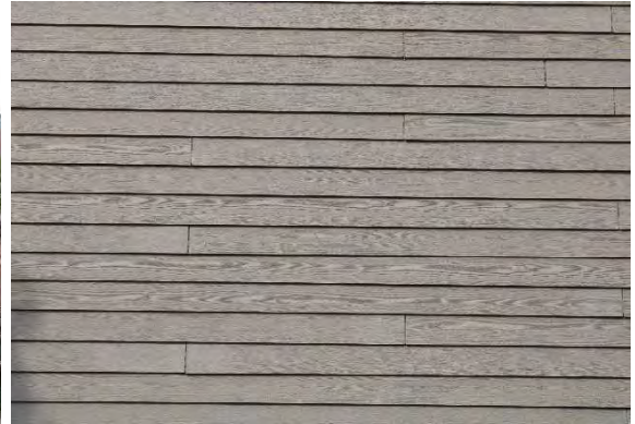
Photo 9: Wood siding, looking west
