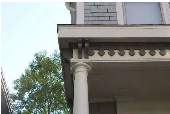
Photo 5: Wooden detailing on porch roofline
