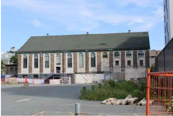
Photo 1: Showing roof and height, looking north
