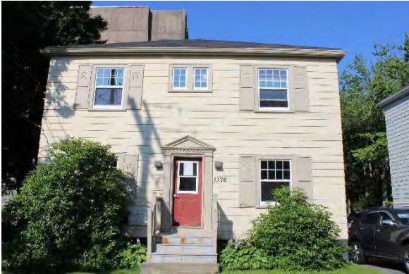
Photo 3: Symmetrical front façade, looking west
