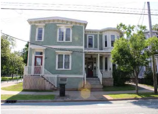
Photo 10: Two storey structure, looking east
