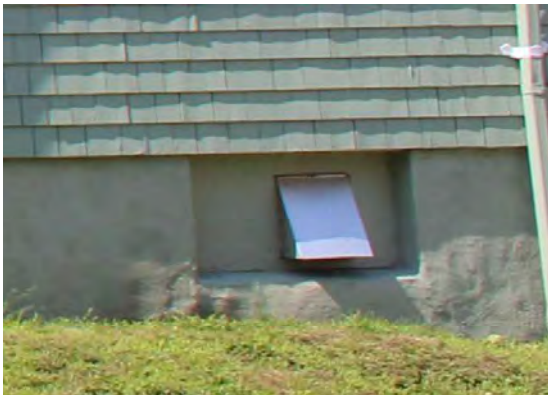
Photo 14: Parged concrete foundation
