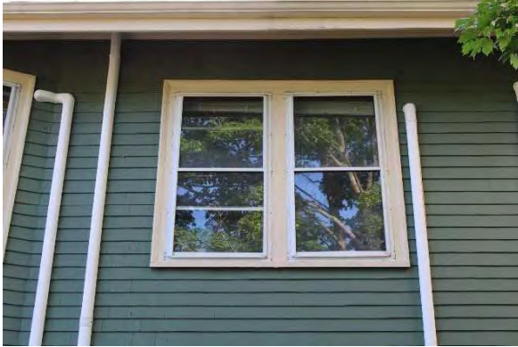
Photo 6: Representative window opening, looking east
