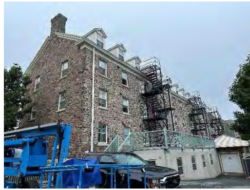
Photo 35: Cornice, return eaves, and dormers, looking east (HRM 2023b)
