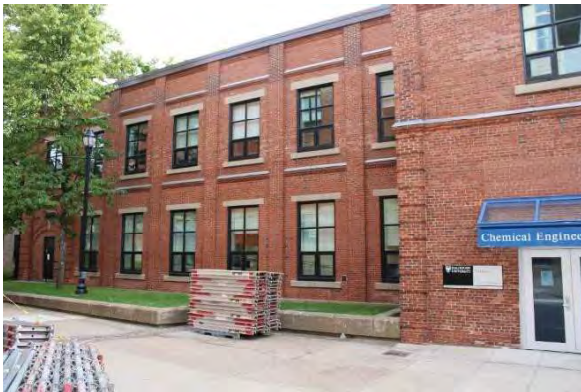
Photo 11: Concrete lintels and sills, looking northeast
