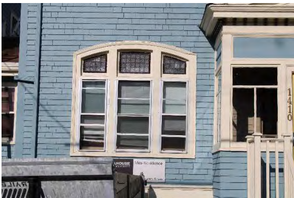
Photo 17: Segmental arch opening wood sash window, looking west
