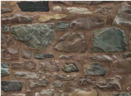
Photo 36: Stone cladding, looking east (HRM 2023b)
