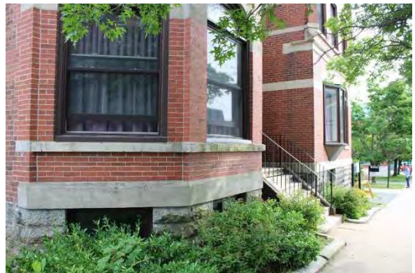
Photo 13: Rusticated stone foundation on front façade, looking northeast
