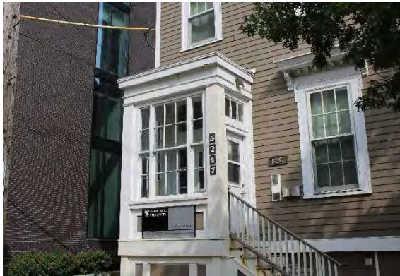
Photo 4: Off-centre front entrance and enclosed porch, looking northwest
