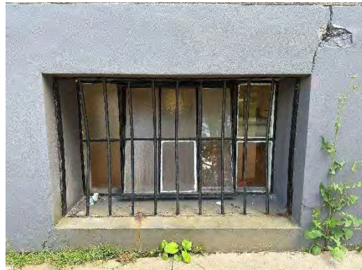
Photo 10: Representative foundation and basement window section, looking south
