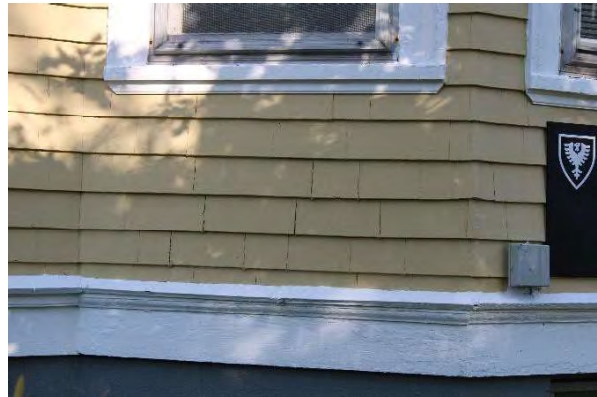
Photo 12: Wood shingle exterior and belt course, looking west
