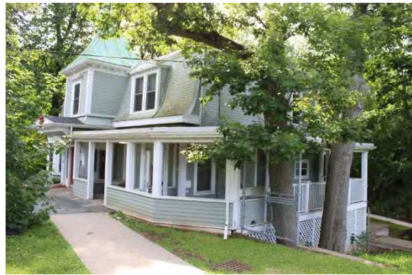
Photo 15: Wraparound verandah, looking southeast
