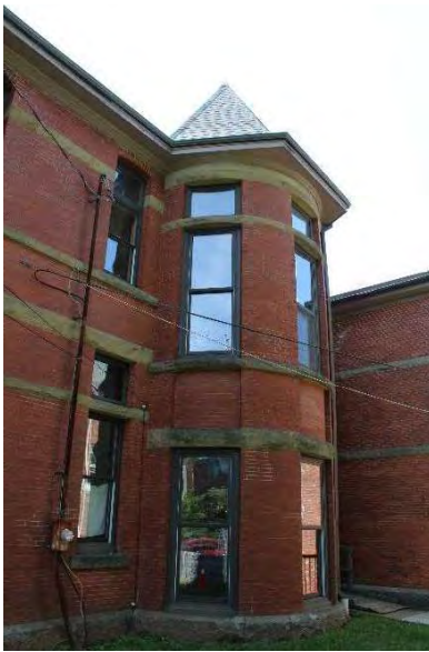
Photo 19: Tower with hexagonal roof on northwest façade, looking southwest
