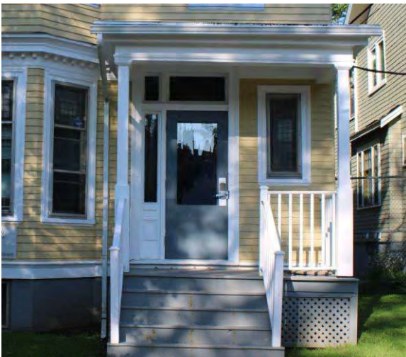
Photo 17: Partial-width porch and main entrance, looking west
