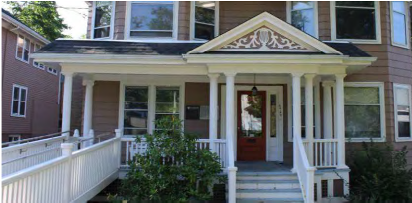
Photo 21: Porch, looking south
