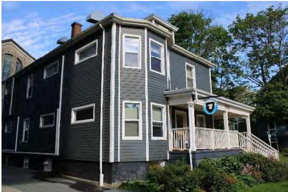
Photo 5: Two storey bay window, looking northwest
