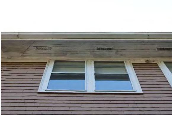
Photo 5: Representative window openings, looking east
