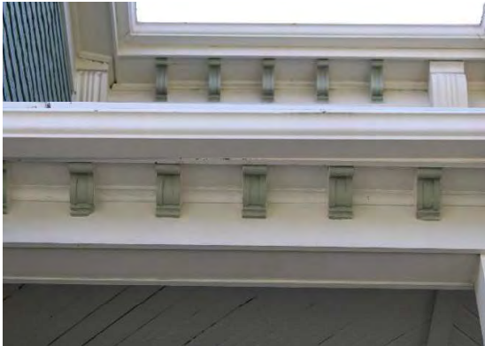
Photo 12: Italianate brackets on roofline
