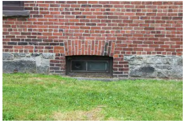
Photo 17: Stone foundation on west façade, looking east
