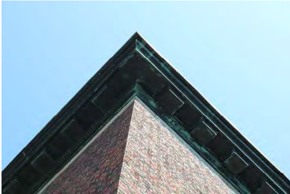
Photo 14: Copper cornice and brackets, looking west
