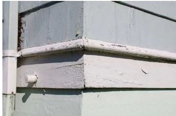
Photo 12: Wood band, looking northwest
