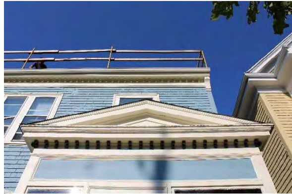
Photo 4: Cornice and bracket, looking west
