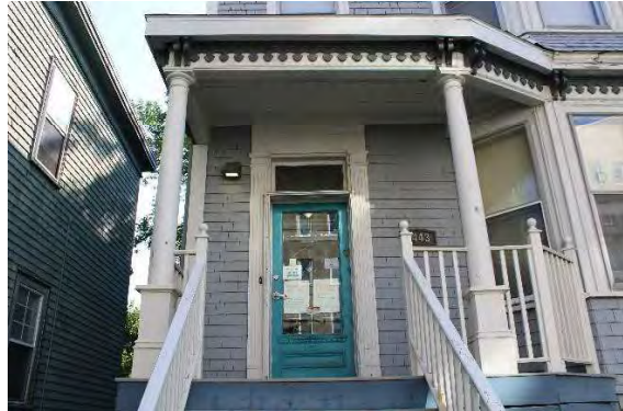
Photo 2: Partial width porch with pilasters on west main entrance, looking east
