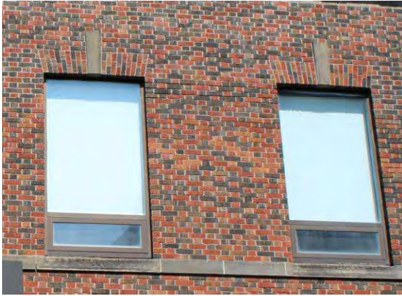
Photo 23: Representative window opening with voussoir and keystone, looking east
