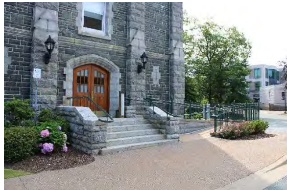
Photo 23: Secondary entrance, looking east
