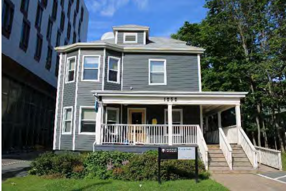
Photo 1: General view of 1252 LeMarchant Street showing simple, box-shaped, two-and-one-half storey, 3-bay design with a lack of decoration and asymmetrical front, looking west
