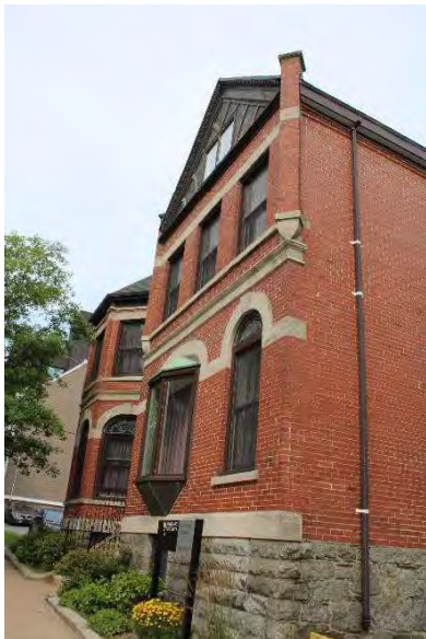
Photo 1: Front (south) façade with stretcher bond brick pattern and rusticated block foundation, looking northwest
