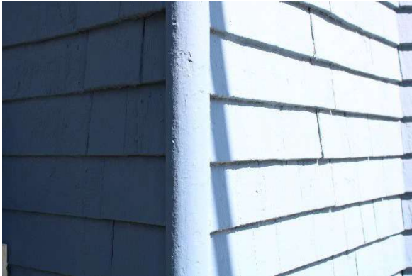
Photo 3: Painted shingle exterior
