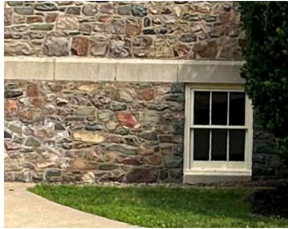
Photo 32: Belt course and representative basement window opening, looking north
