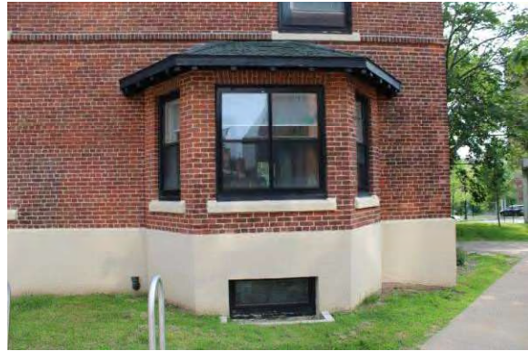
Photo 8: Bay window on the west façade, looking east
