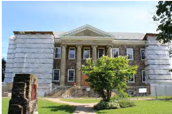
Photo 4: Front façade, looking south
