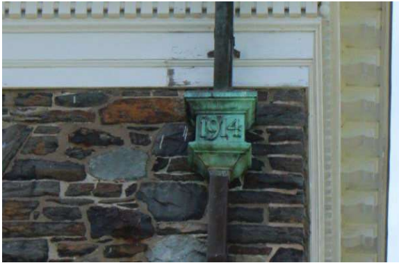
Photo 18: Copper downspout, looking north
