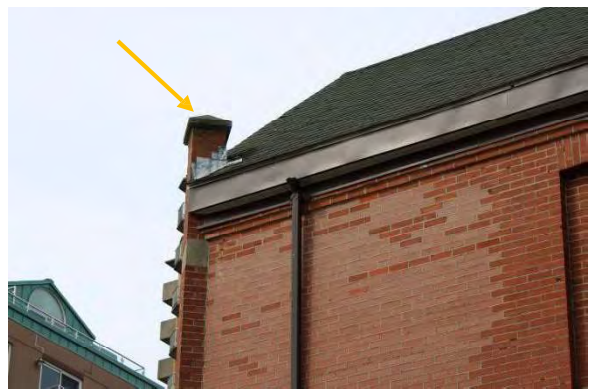
Photo 7: Cap stone, looking southwest
