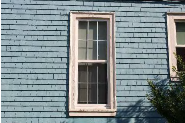
Photo 7: Wooden rectangular window openings
