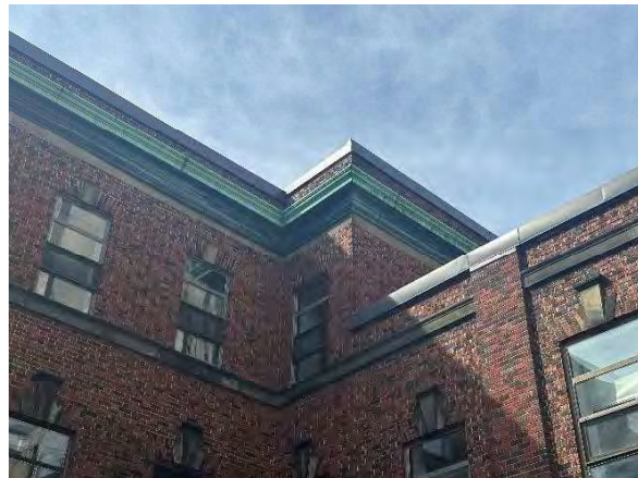
Photo 2: Copper cornice, looking north
