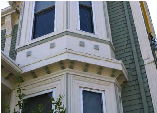
Photo 18: Detailing on bay window
