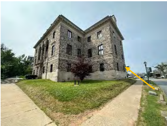
Photo 6: Beltcourses (denoted by arrow), looking southwest
