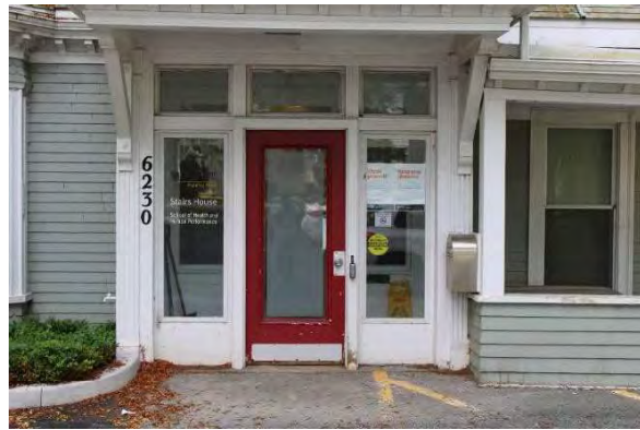
Photo 7: Rectangular transom windows and sidelights with wooden door, looking south
