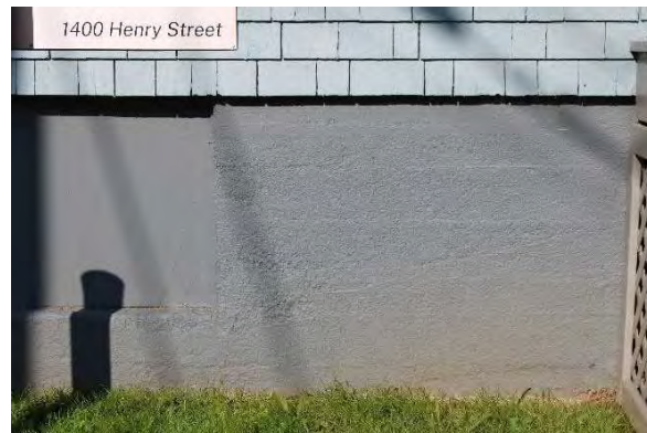
Photo 12: Concrete foundation, looking north
