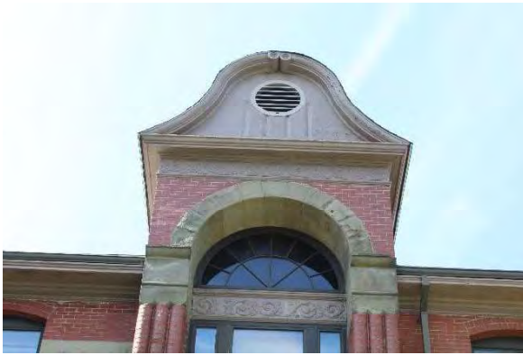
Photo 15: Eyebrow wall dormer on the front façade, looking southwest
