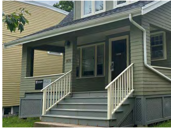
Photo 7: Full-width porch, looking southwest (HRM 2023b)
