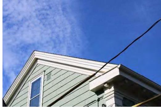
Photo 2: Roof pitch, cornice, and return eaves, looking northwest
