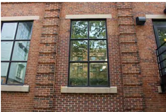
Photo 9: Pilasters, looking east
