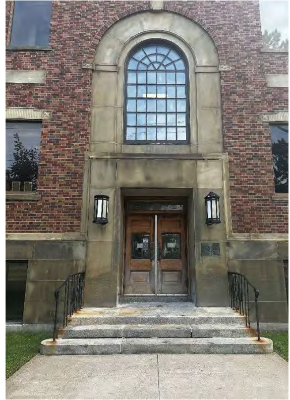
Photo 10: Secondary entrance, looking east
