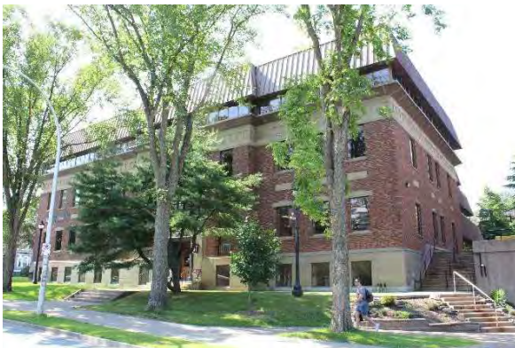
Photo 1: Dentistry Building, looking north
