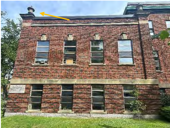
Photo 10: One storey section, representative photo, urn denoted by arrow, looking north
