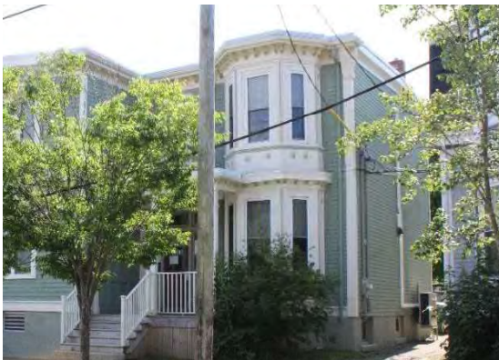
Photo 20: Two storey bay window
