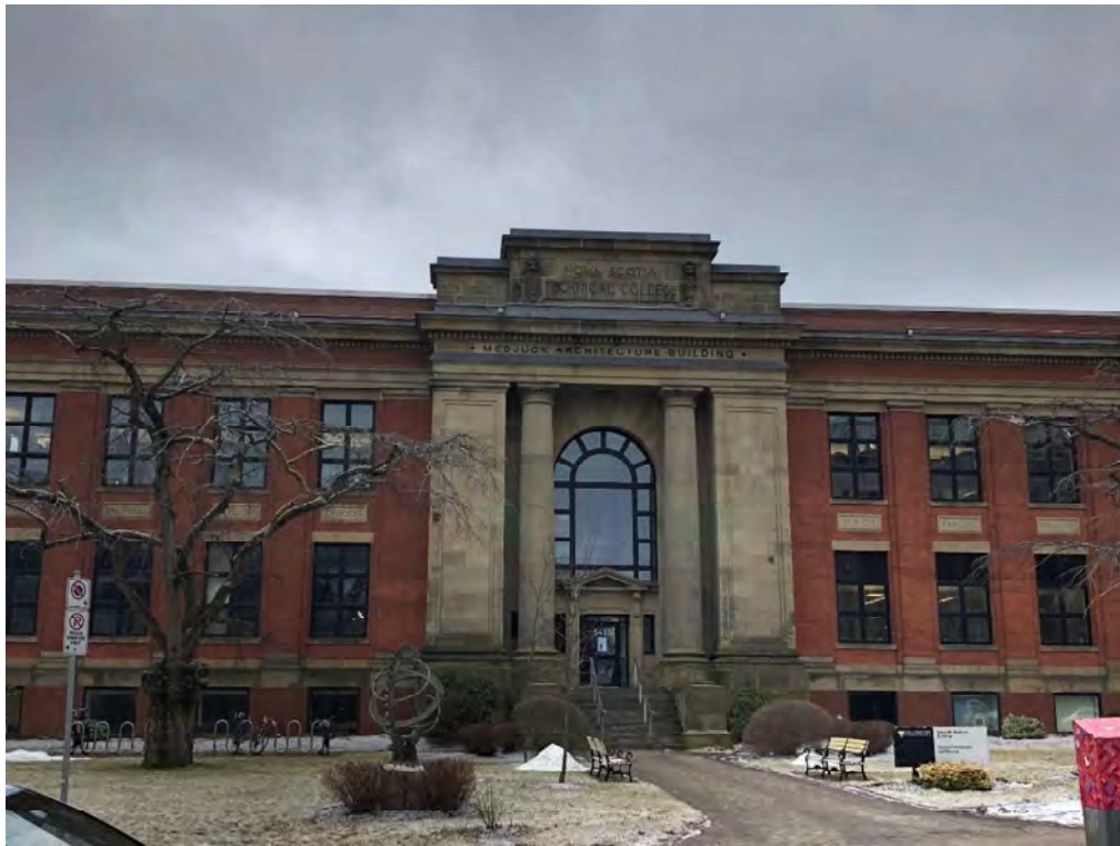
Figure 8: Main entrance of 5410 Spring Garden Road (January 2020)
