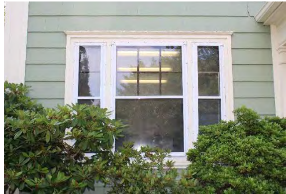
Photo 6: Representative wood sash window, looking south
