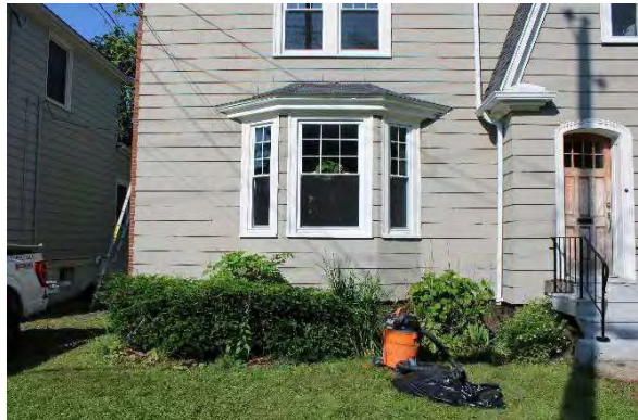
Photo 20: Bay window, looking west
