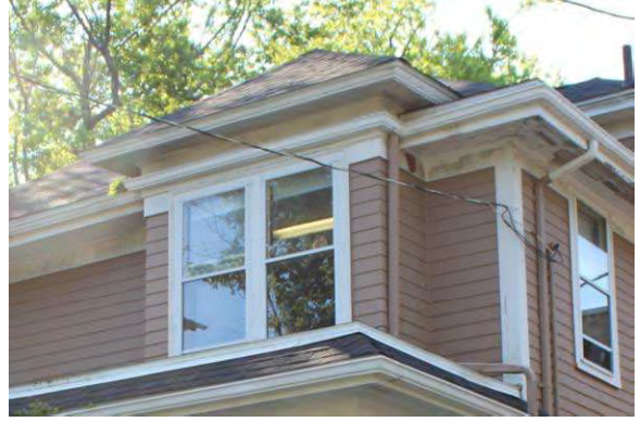
Photo 8: Second storey hip bay, looking south
