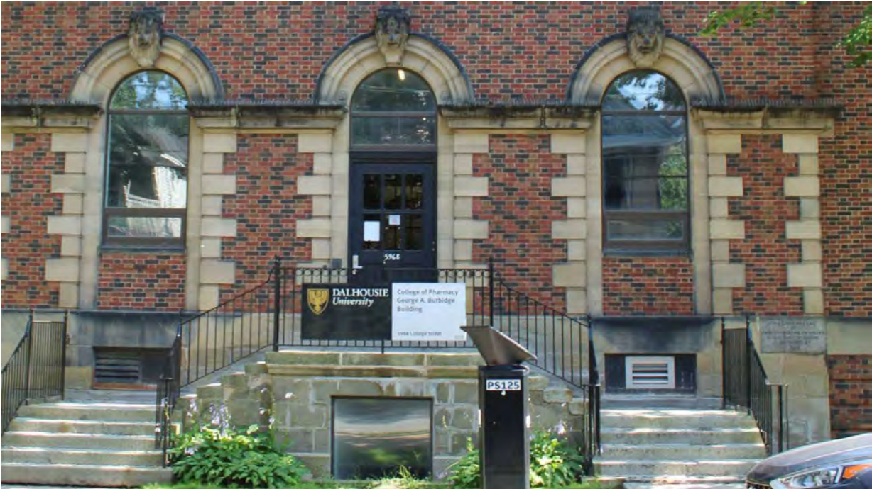
Photo 22: Arched window openings flanking frontispiece, looking south
