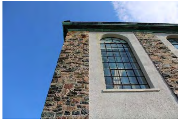
Photo 4: Representative exterior details, looking east
