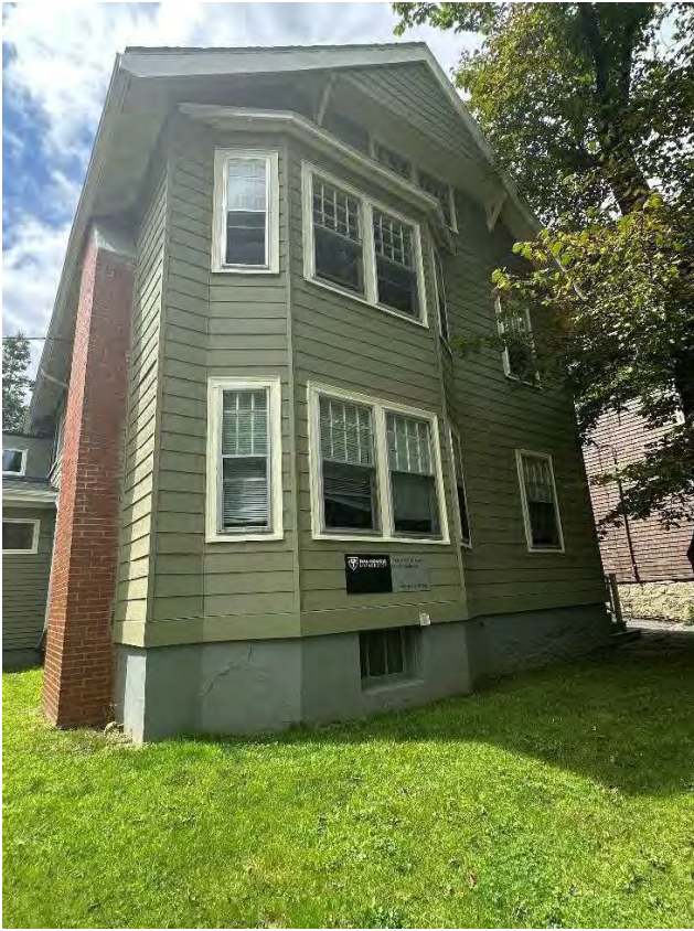
Photo 13: Asymmetrical front façade and capped chimney, looking west (HRM 2023b)
