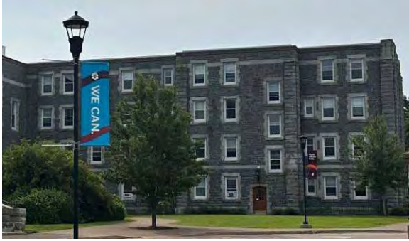
Photo 18: Stone clad section of south wing, looking south (HRM 2023b)
