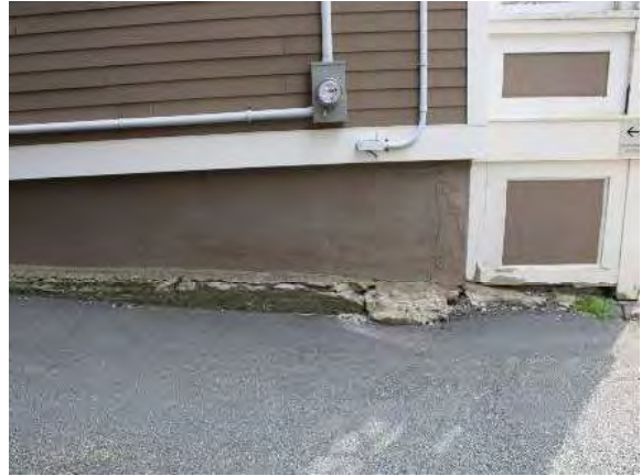
Photo 14: Parged foundation on the west façade, looking east
