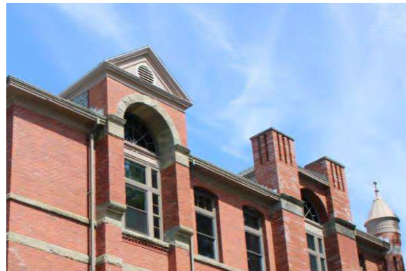
Photo 16: Gable and hip wall dormers on the southeast façade, looking north
