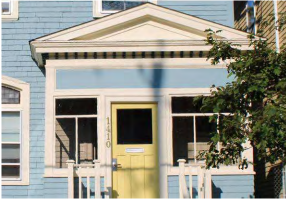
Photo 19: Enclosed porch, looking west
