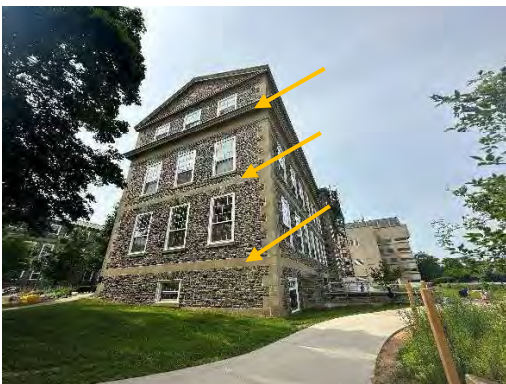
Photo 5: Belt courses, denoted by arrows, looking north
