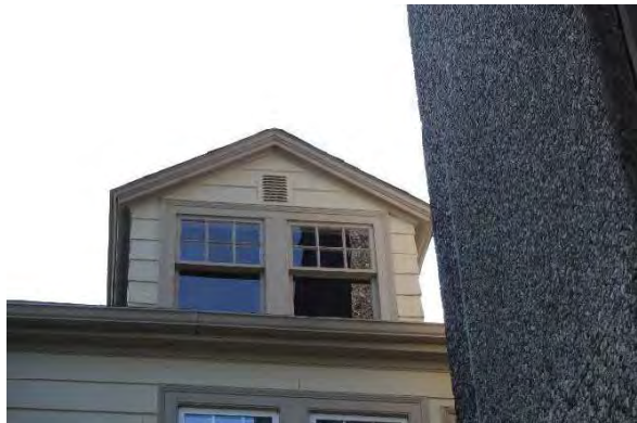
Photo 6: Rear façade dormer, looking east
