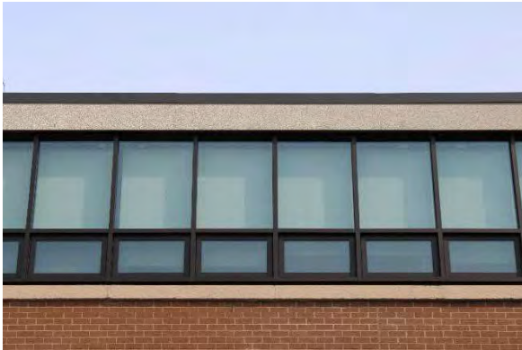
Photo 7: Ribbon window on the south façade, looking north
