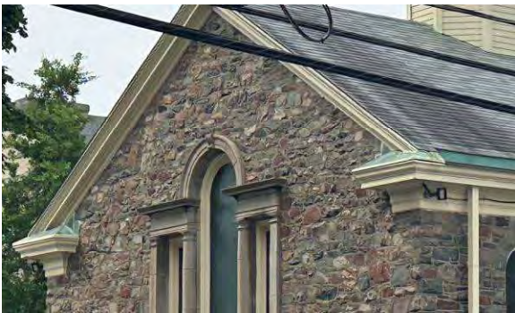
Photo 27: Cornice and return eaves, looking southwest (HRM 2023b)
