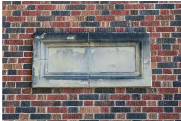
Photo 17: Stone panel, looking south
