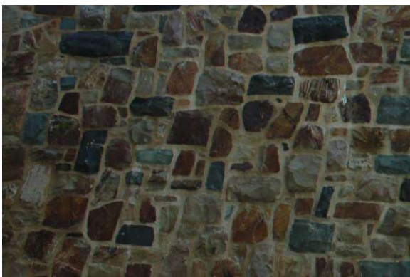
Photo 7: Stone clad exterior, looking east
