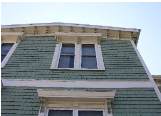
Photo 5: Italianate brackets along roofline
