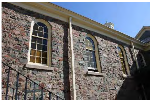
Photo 30: Representative window openings, looking north
