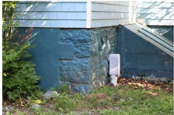
Photo 10: Cut stone foundation with concrete block reinforcements
