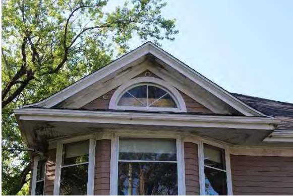
Photo 7: Pediment window within gable, looking south
