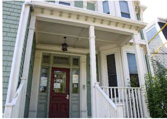
Photo 13: Pilasters, sidelights and transom on main entrance
