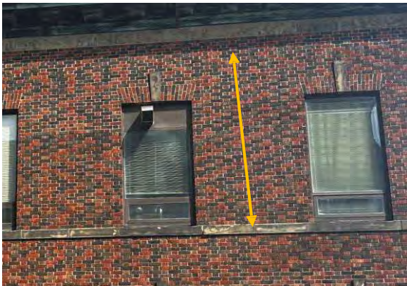
Photo 16: Representative belt course sections, denoted by arrow, looking south
