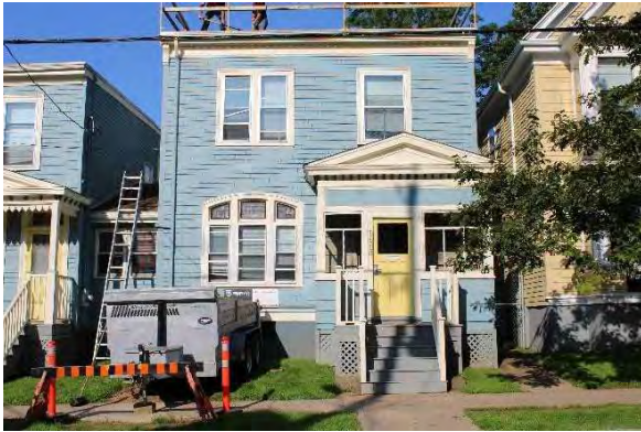
Photo 3: 1410 Henry Street, looking west
