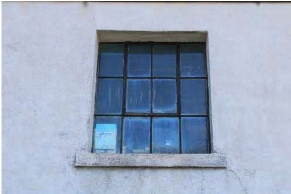
Photo 7: Representative square opening metal sash window, looking east
