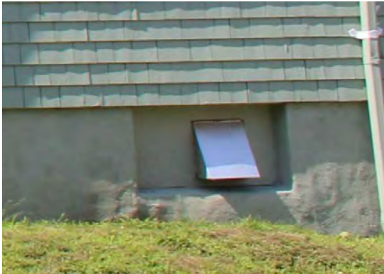
Photo 7: Parged concrete foundation
