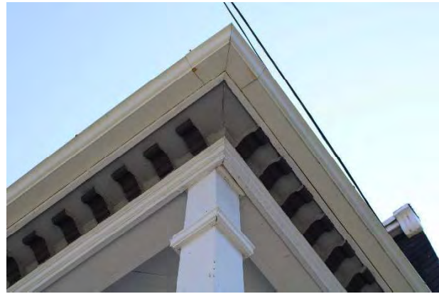
Photo 4: Dentil detailing under porch roofline
