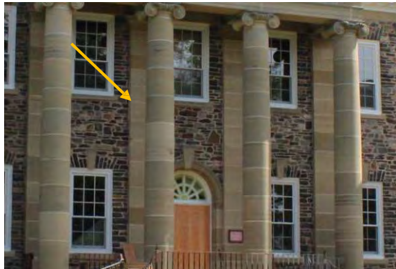
Photo 6: Pilasters (denoted by arrow), looking south
