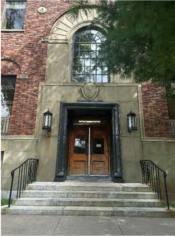
Photo 9: Principal entrance, looking north
