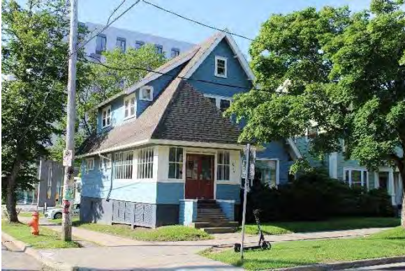
Photo 1: General view showing height, looking south
