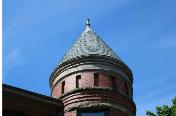
Photo 18: Conical roof of tower on north corner, looking northwest
