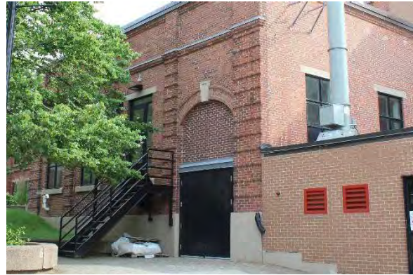
Photo 15: Bricked in arch, looking northeast
