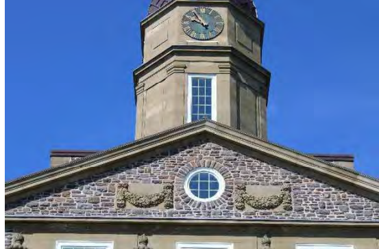
Photo 8: Circular window flanked by swag, looking west
