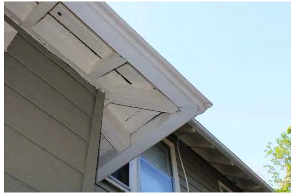
Photo 10: Wood fascia and soffits, looking south
