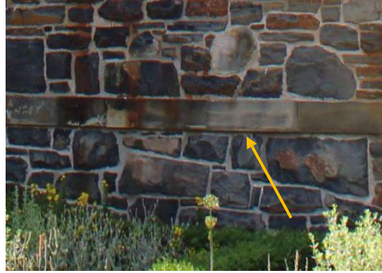
Photo 17: Belt course (denoted by arrow), looking north
