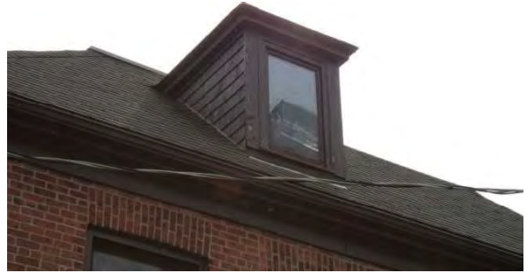
Photo 9: Wood shingles on roof dormer, looking southeast
