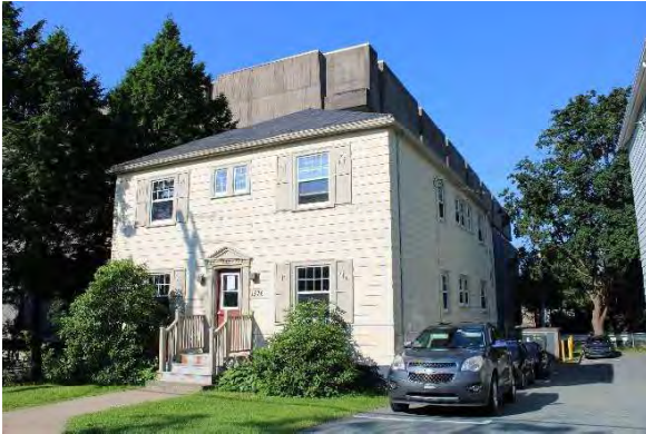
Photo 1: General view of residence showing hip roof, looking west
