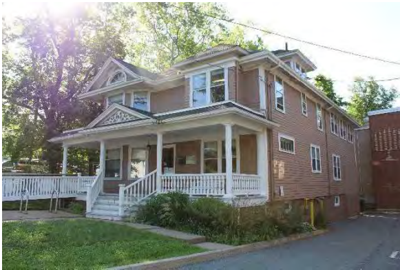
Photo 1: General view, showing height, looking south
