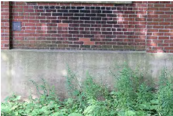
Photo 3: Close up showing common bond construction and parged foundation, looking west
