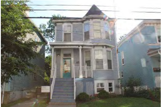
Photo 1: 1443 Seymour Street, looking east
