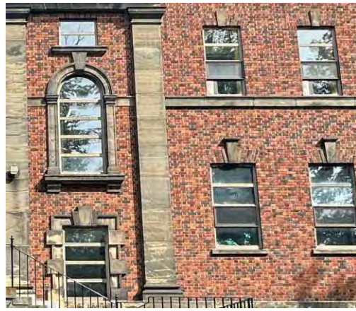
Photo 7: Representative window openings, looking north
