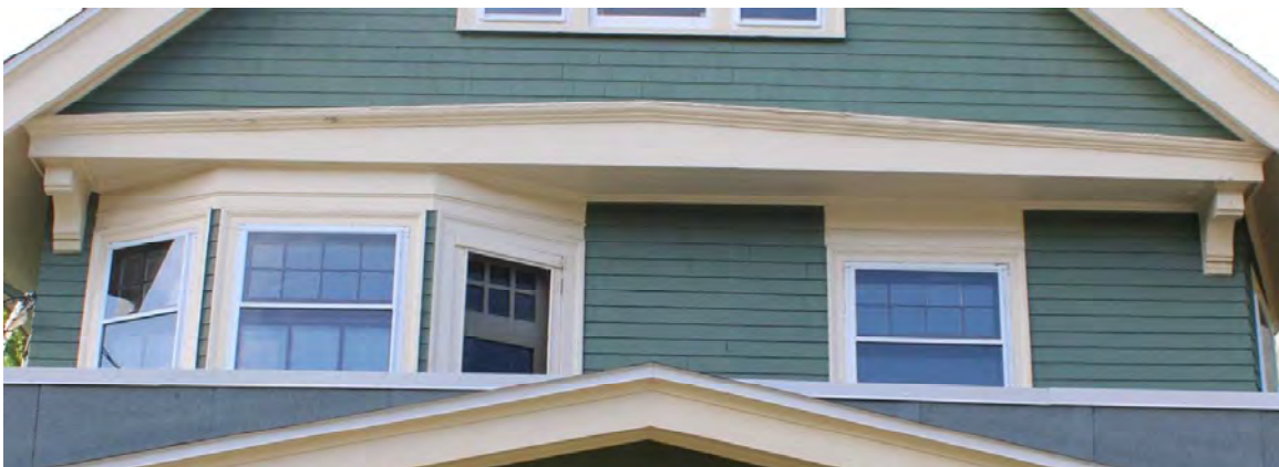
Photo 5: Bay window and low-pitched pediment with brackets, looking south
