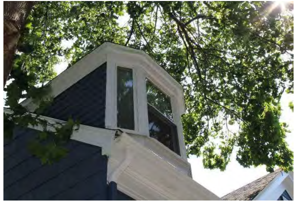
Photo 2: North façade Scottish dormers
