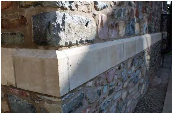
Photo 13: Belt course, looking north
