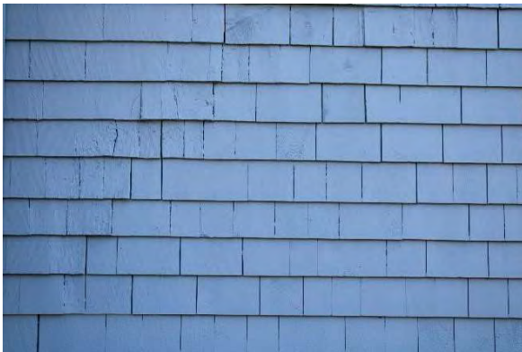
Photo 7: Shingle exterior, looking north
