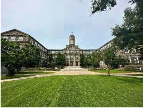
Photo 1: Front façade, showing height and U-shape, looking west
