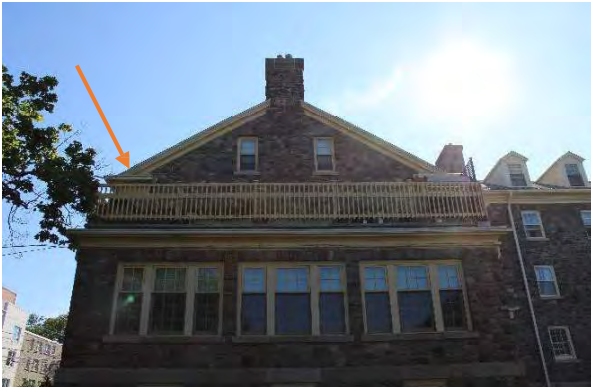
Photo 17: Cornice and return eaves, denoted by arrow, looking east
