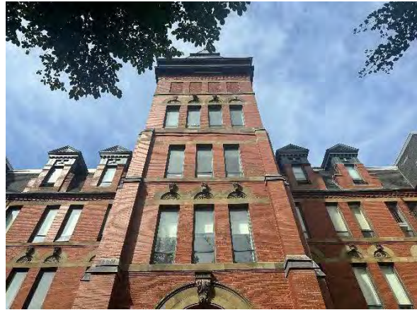
Photo 2: Tower, looking west
