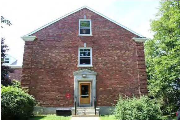
Photo 6: Red brick quoin, looking southwest
