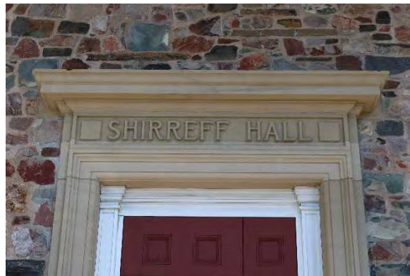
Photo 12: Main entrance door showing inscription, looking north
