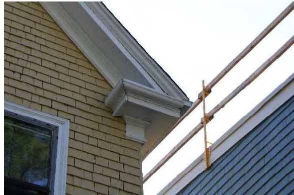
Photo 2: Return eave at southwest corner of rear façade, looking east
