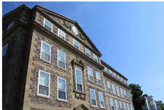
Photo 12: Secondary entrance bay, looking north
