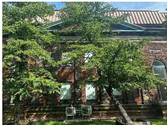
Photo 19: Projecting bay of south façade, looking north
