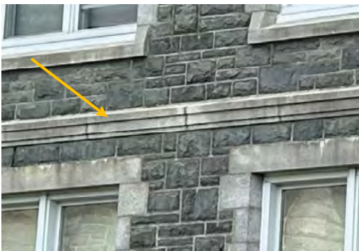
Photo 4: Representative belt course, denoted by arrow, looking east (HRM 2023b)
