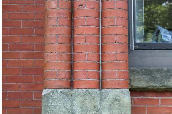
Photo 22: Close up view of brick columns, looking southwest
