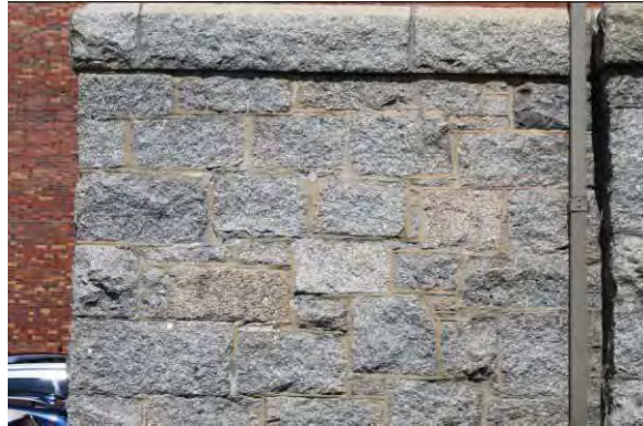
Photo 30: Cut stone foundation from the original structure, looking northwest
