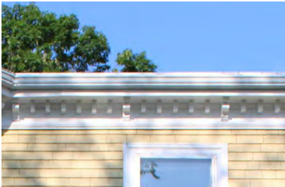
Photo 11: Wood cornice, looking west
