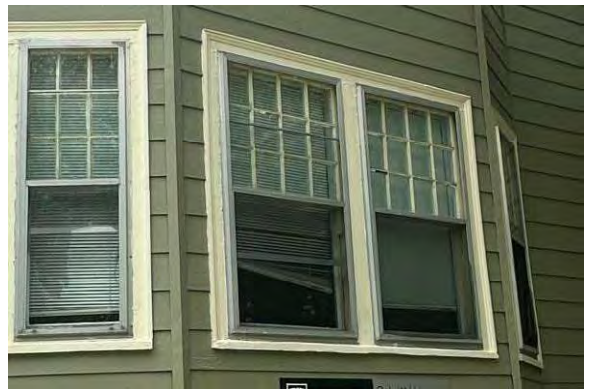
Photo 12: Wood sash windows, looking west (HRM 2023b)
