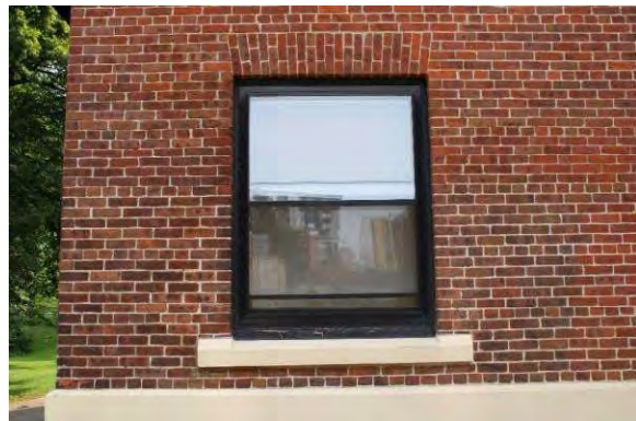
Photo 6: Representative example of window opening, looking east
