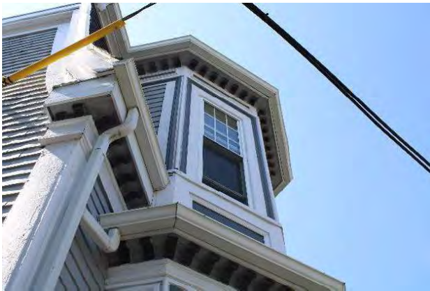
Photo 9: Second storey bay window
