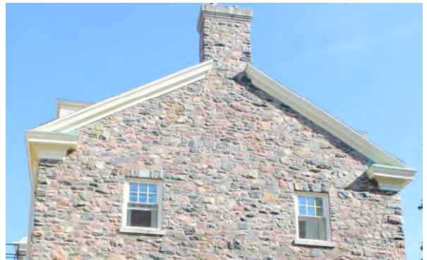
Photo 4: Cornice and return eaves, looking north (HRM 2023b)
