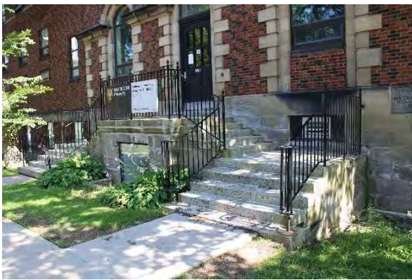
Photo 25: Staircase, looking south
