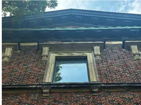
Photo 24: Representative window with stone surround, looking south
