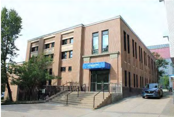
Photo 1: General view showing height and box-like shape, looking southwest
