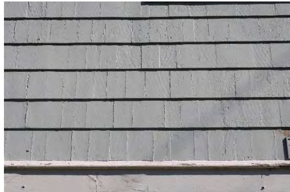
Photo 8: Wood clad exterior, looking east
