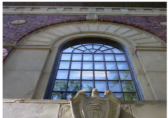
Photo 8: Stone surround and arched window, looking north
