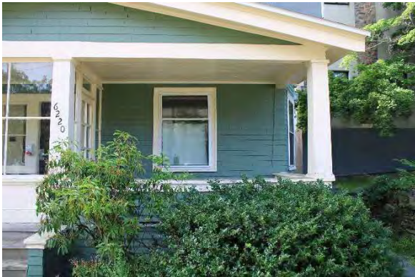
Photo 8: Open part of front porch, looking south
