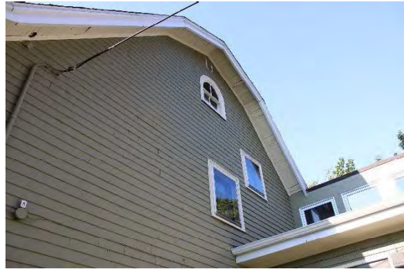
Photo 2: Roof and soffit details, looking south
