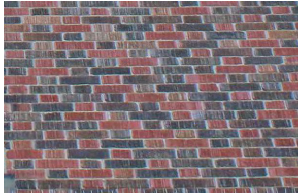
Photo 15: Red brick exterior, looking south
