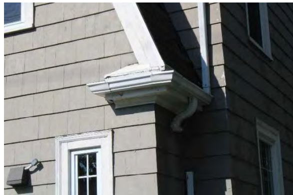
Photo 16: Representative return eave details, looking west
