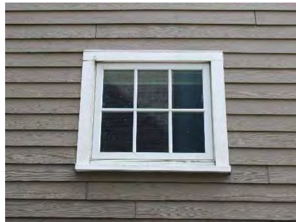
Photo 12: Vinyl sash window with mullions from side (west) façade, looking east
