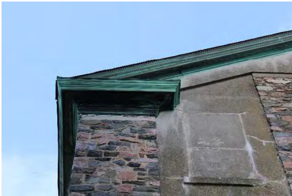
Photo 3: Representative copper eaves, soffits, and fascia, looking east
