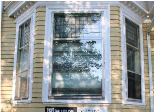
Photo 15: Leaded glass windows, looking west
