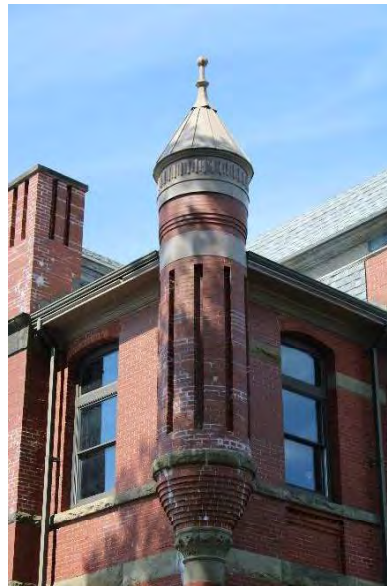
Photo 20: Cantilevered extension on the east corner, looking west
