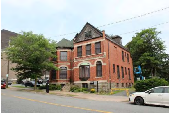
Photo 4: Front façade, looking northwest
