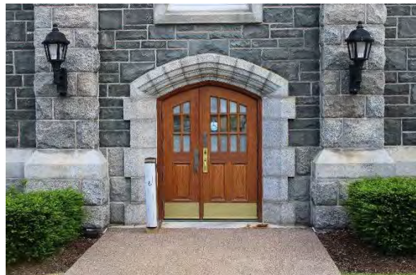
Photo 17: Secondary entrance, looking east
