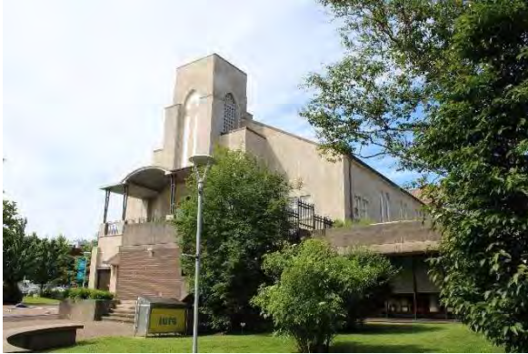
Photo 24: General view showing roof pitch and tower, looking southwest
