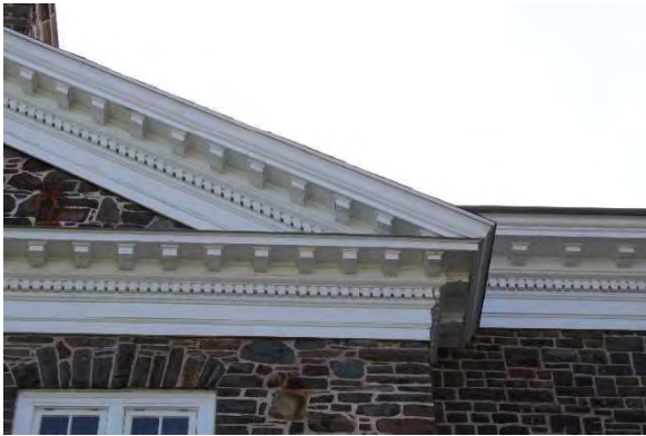
Photo 12: Cornice and pediment details, looking north
