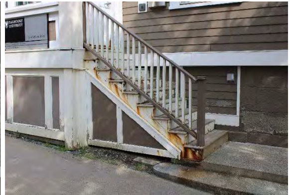
Photo 5: Short flight of stairs leading to front entrance, looking northwest
