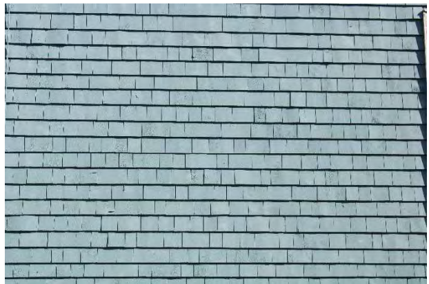
Photo 6: Painted shingle exterior
