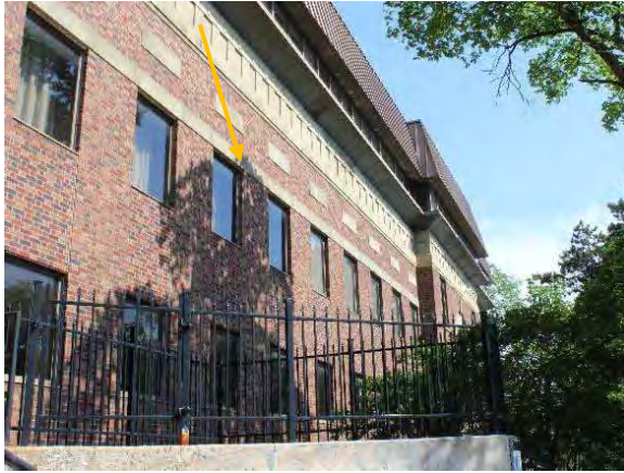
Photo 5: Beltcourse, denoted by arrow, looking south
