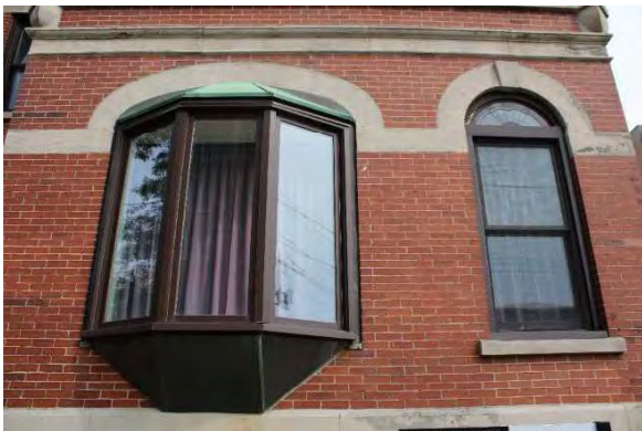
Photo 12: Bay window, looking north
