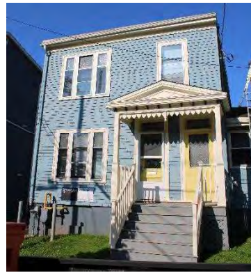
Photo 8: Front façade, looking west
