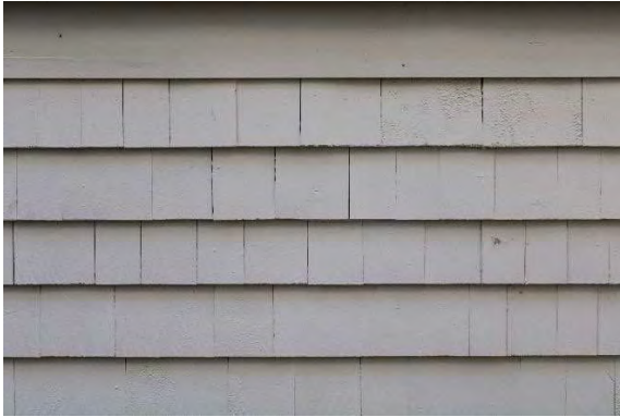
Photo 7: Wooden shingling exterior
