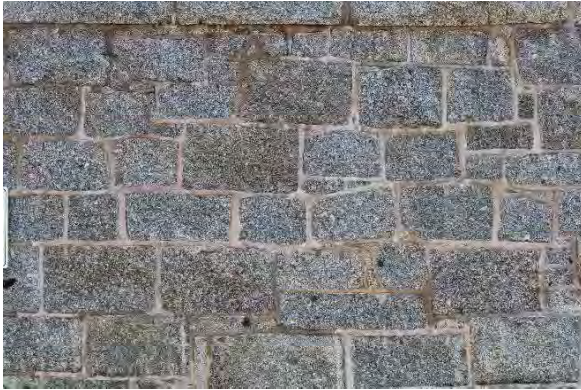
Photo 29: Cut stone foundation from the structure's addition, looking northeast
