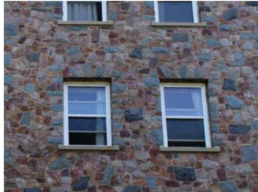
Photo 10: Rectangular window openings on 1967 addition, looking east
