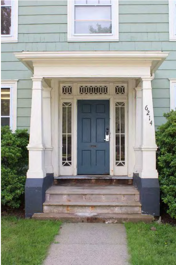
Photo 7: Partial width porch and main entrance, looking south
