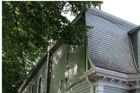
Photo 3: Side view of mansard roof, looking southwest
