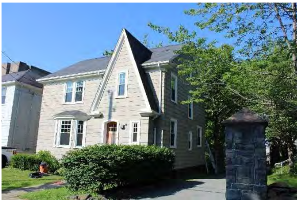
Photo 15: General view showing height and roof pitch, looking west
