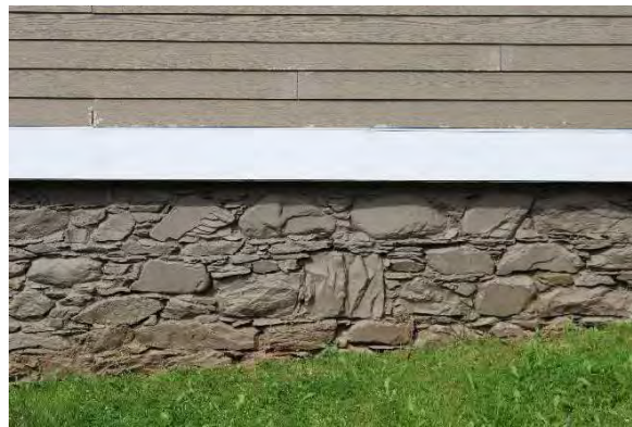
Photo 10: Stone foundation, looking west
