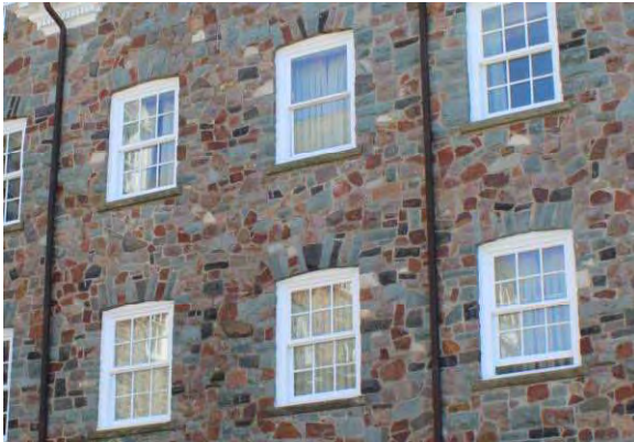
Photo 9: Segmental arch window openings, looking east
