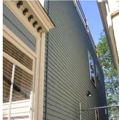
Photo 14: Roof pitch, looking west
