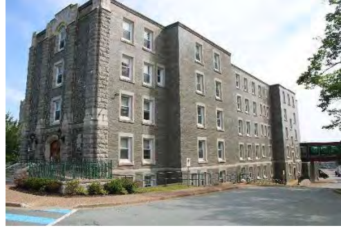
Photo 19: Glazed brick section of south wing, looking northeast
