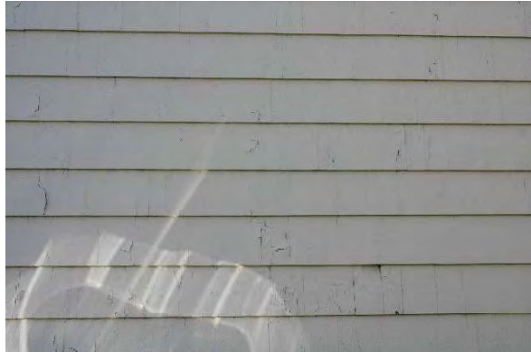
Photo 2: Wood cladding details, looking south
