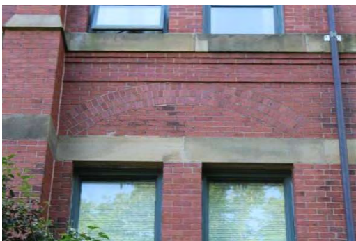
Photo 5: Brick exterior and decorative brick arch, looking west
