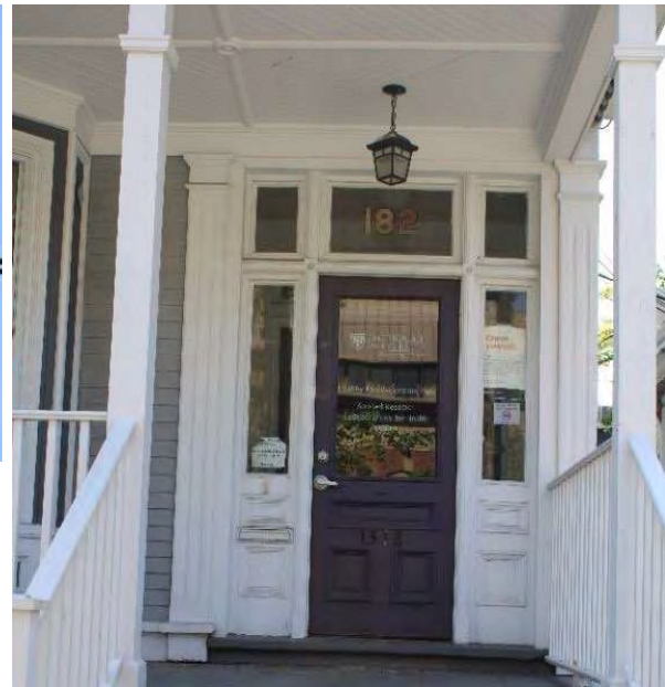
Photo 10: Entrance with wood door, transoms and sidelights
