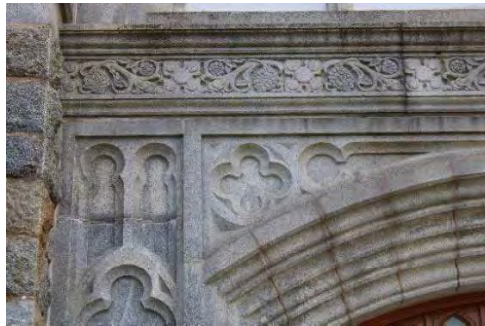
Photo 9: Representative tracery details, looking east
