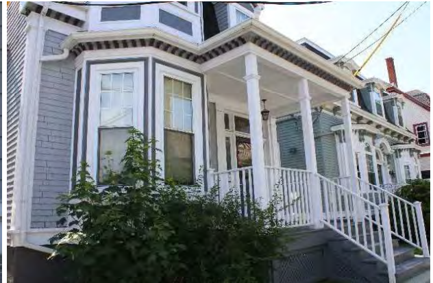
Photo 8: Partial width porch and first storey bay window
