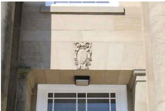
Photo 11: Escutcheon, looking west
