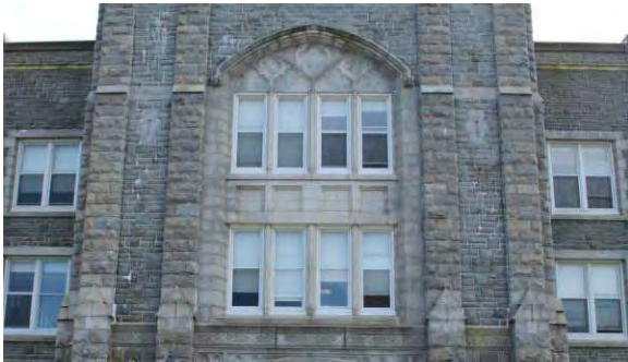
Photo 8: Arched stonework, looking east
