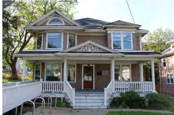
Photo 6: Asymmetrical front façade, looking south
