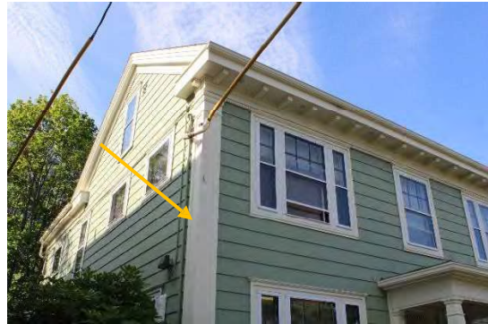
Photo 4: Pilaster, denoted by arrow, looking south
