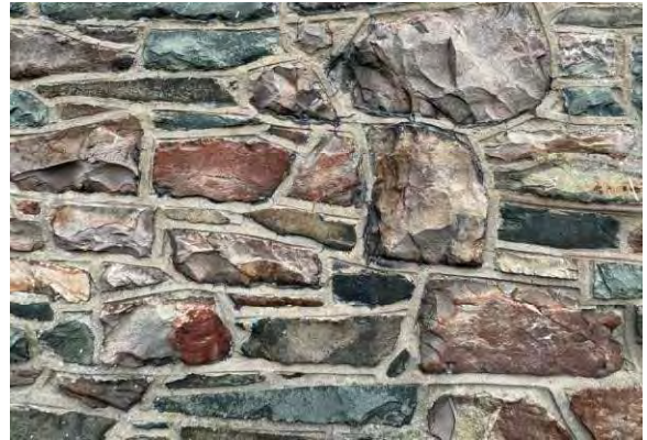
Photo 18: Stone exterior, looking east
