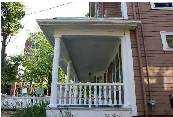
Photo 9: Porch columns, pilasters, and railing, looking east
