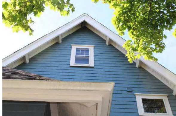
Photo 2: Gable roof, looking south
