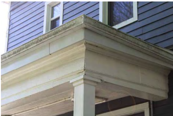
Photo 7: Plain wooden cornice and supports on porch, looking northeast
