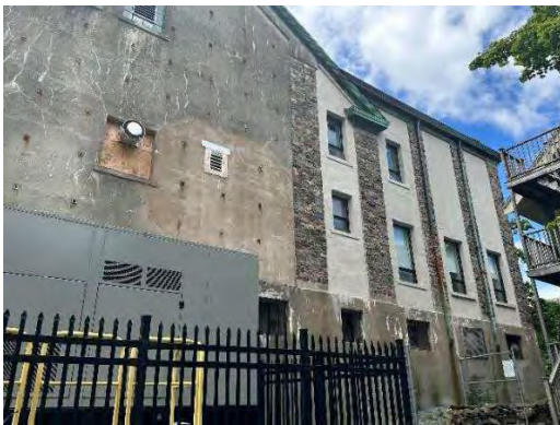
Photo 5: Representative cladding, looking west
