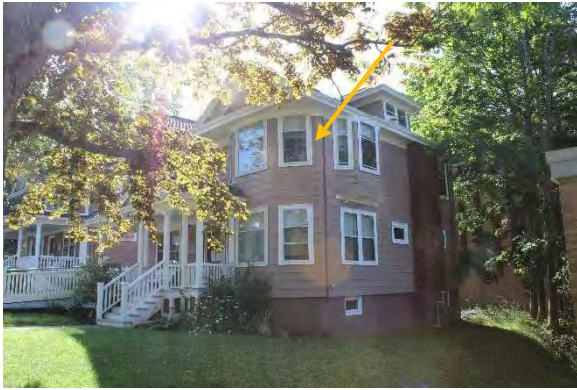
Photo 19: Full length gable bay, denoted by arrow, looking southeast
