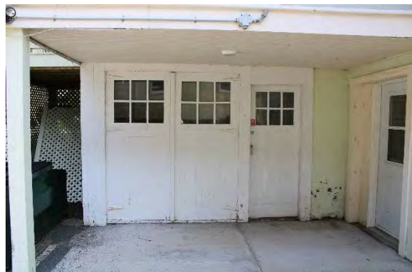
Photo 14: Garage doors, looking north
