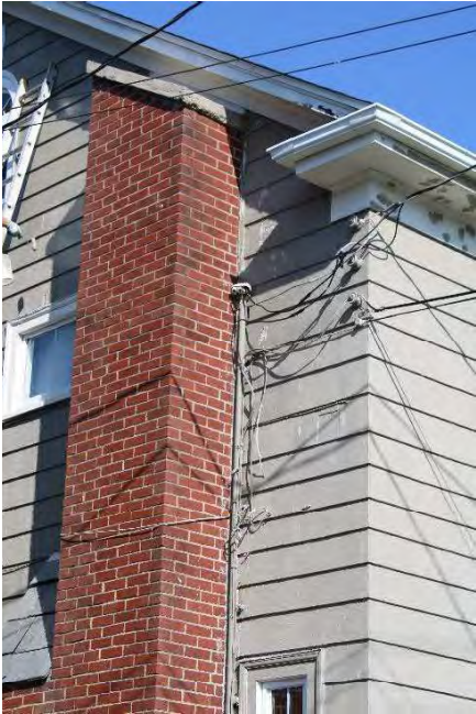
Photo 23: Capped red brick chimney, looking north
