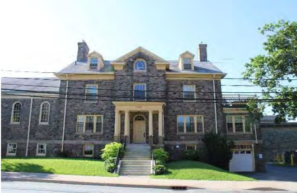
Photo 15: General view of President’s Lodge, looking south (HRM 2023b)
