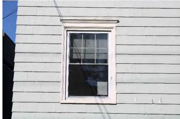
Photo 10: Representative window opening, looking west
