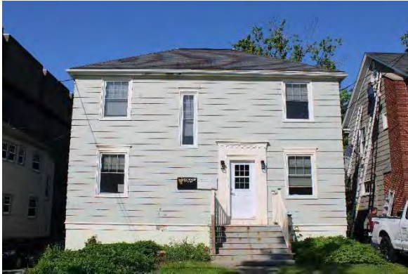
Photo 9: Asymmetrical front façade, looking west
