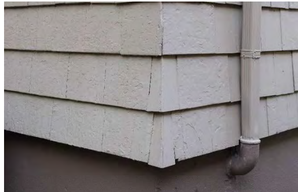
Photo 16: Representative shingle cladding, looking northwest
