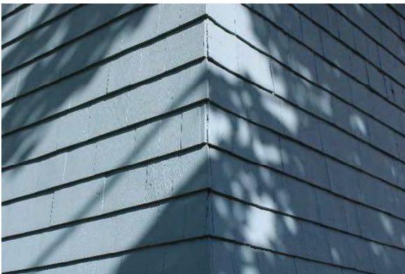
Photo 5: Representative wood shingle details, looking west
