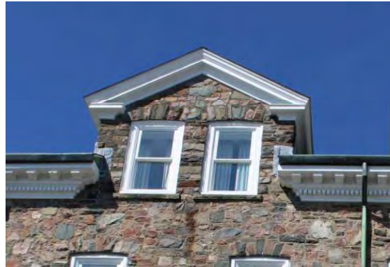
Photo 4: Gable dormer, looking west
