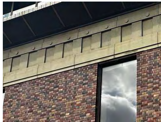
Photo 2: Frieze, looking west
