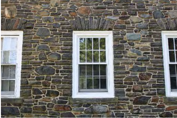
Photo 16: Window opening, looking north
