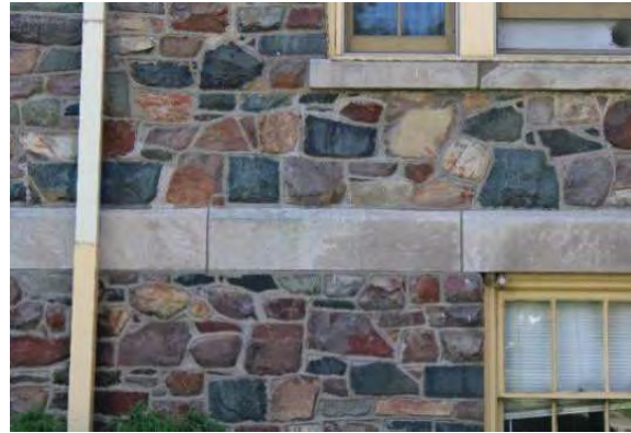
Photo 22: Belt course, looking south
