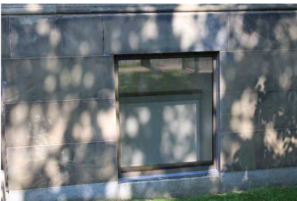
Photo 11: Stone cladding, looking north
