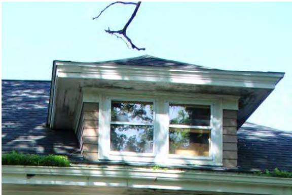
Photo 3: Representative hip dormer, looking west
