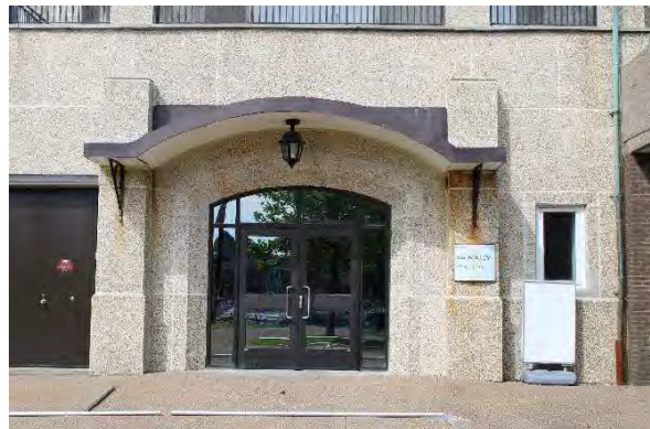
Photo 29: Main entrance, looking west
