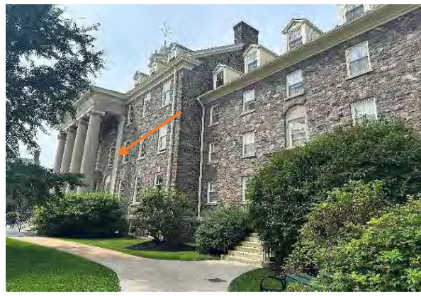
Photo 10: Pillaster, denoted by arrow, looking south (HRM 2023b)
