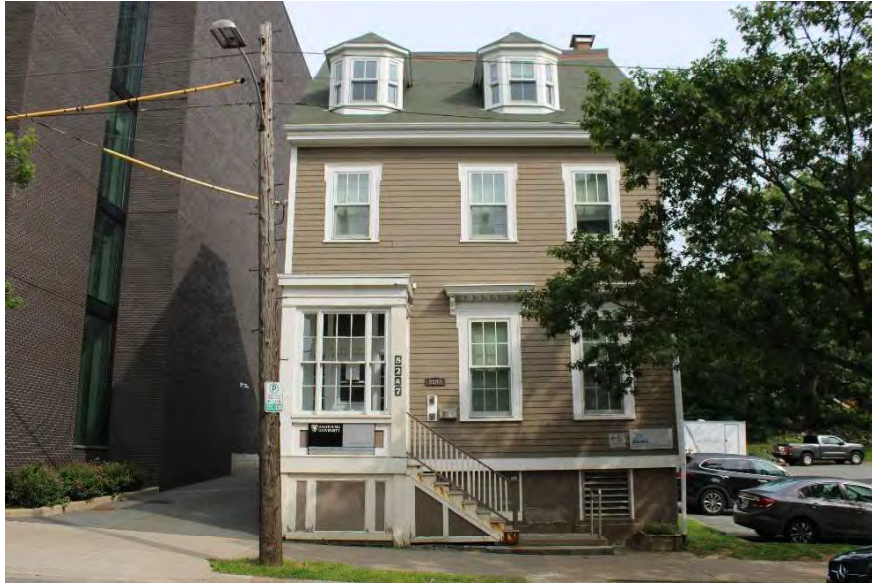
Photo 1: Simple, 3-bay design and proportions inspired by Georgian architecture, looking north
