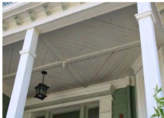
Photo 17: Wood details under roof of porch
