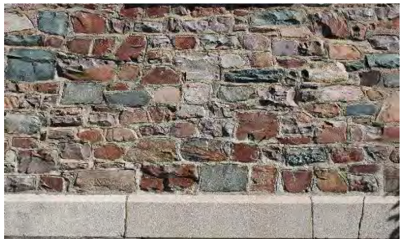
Photo 28: Stone cladding, looking north
