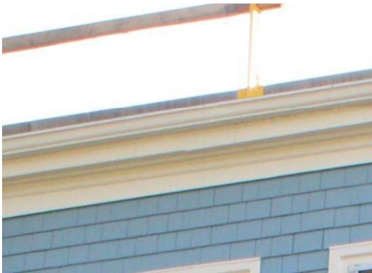
Photo 15: Wood fascia and soffits, looking east
