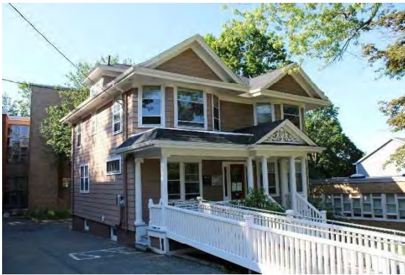
Photo 13: General view showing height, looking south
