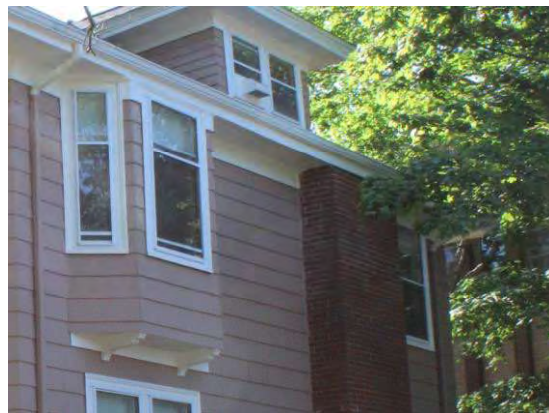
Photo 23: Bay window and former chimney, looking south
