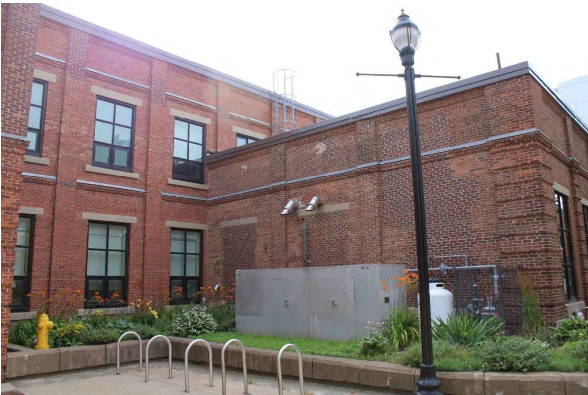
Photo 16: Bricked in window openings and repairs evidenced by different brick and mortar colours, looking southeast
