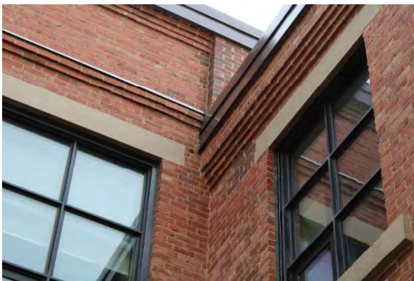
Photo 7: Corbelling, looking southeast
