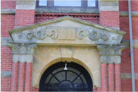
Photo 21: Decorative brick columns and stone pediment above main entrance on the front façade, looking southwest
