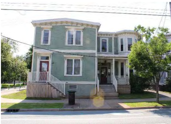
Photo 3: Two storey structure looking east
