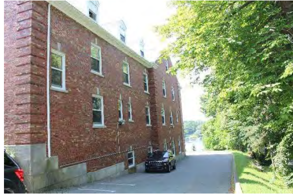
Photo 3: View of the side (northwest) façade showing the transition to three and one half storeys at the rear with additional gable roof dormers, looking southwest
