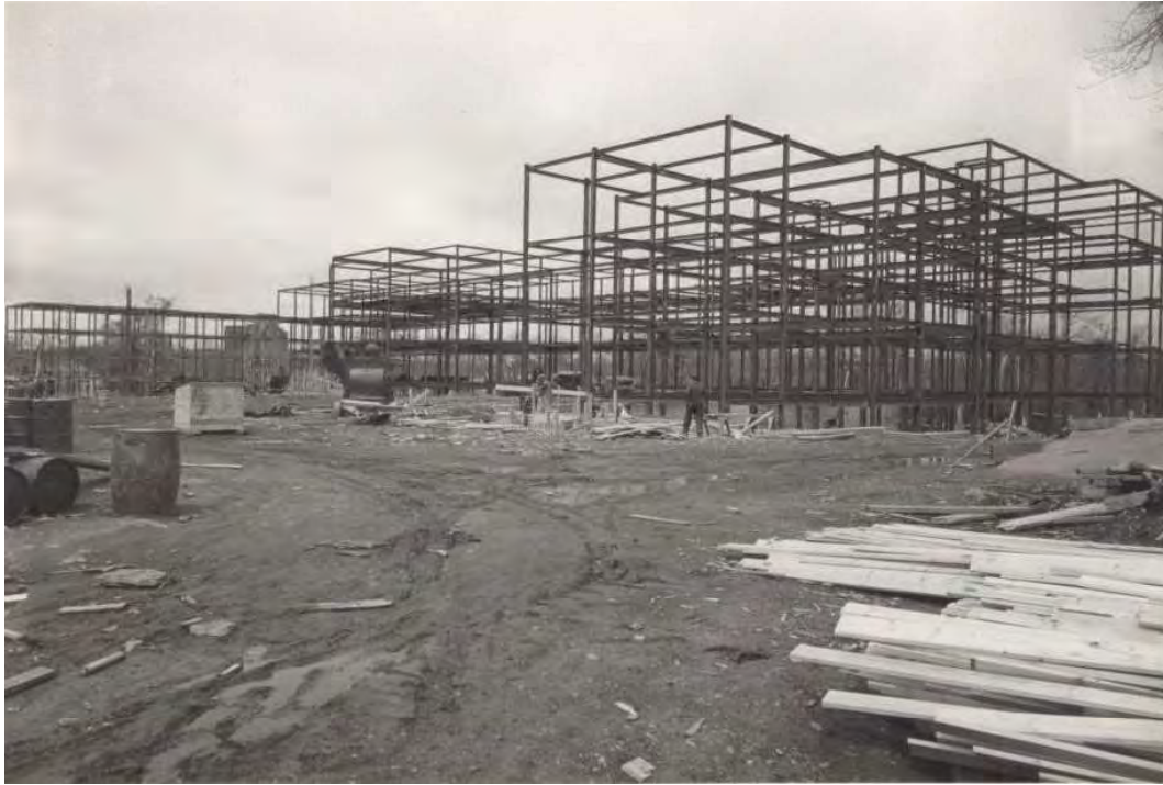
Plate 1: Steel frame of McNally Building, 1950 (SMU Archives 1950a)
