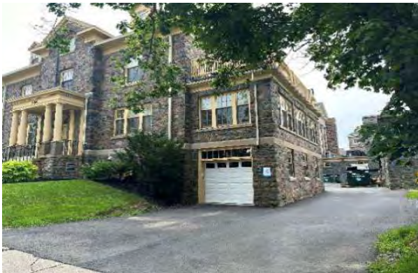
Photo 23: Garage, looking south (HRM 2023b)
