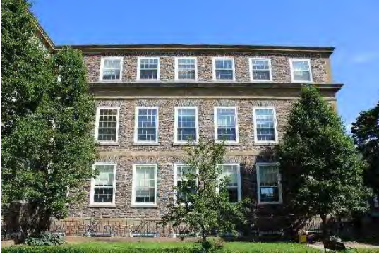
Photo 7: Representative window openings and fenestration, looking north
