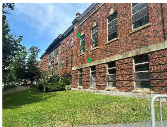
Photo 4: Belt courses (denoted by arrow), looking west
