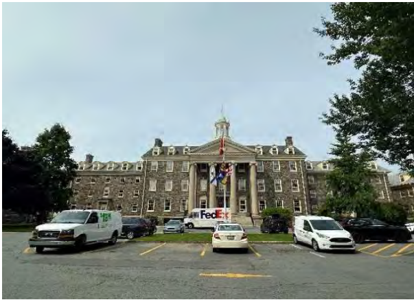
Photo 1: Arts and Administration Building, general plan, looking west (HRM 2023b)
