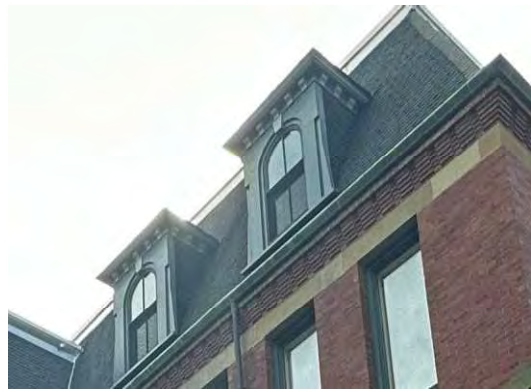
Photo 4: Flat roof dormers, looking north
