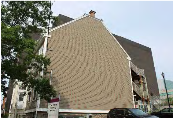
Photo 2: Truncated gable roof, looking northwest
