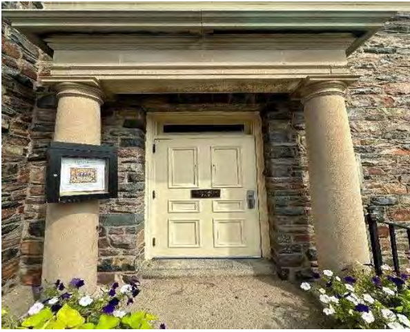
Photo 31: Frontispiece and main entrance, looking north
