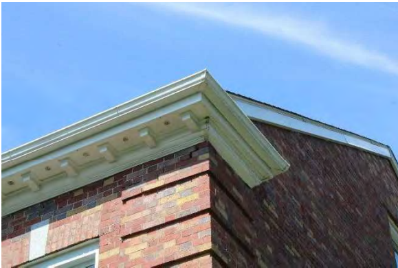
Photo 4: Return eaves, wide soffits and cornice with small brackets, looking west
