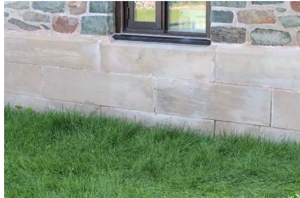
Photo 13: Cut stone foundation cladding, looking west
