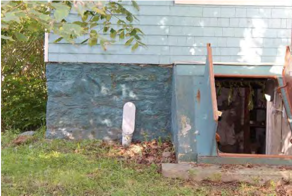
Photo 11: Basement cellar access
