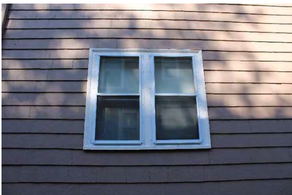
Photo 17: Representative window opening, looking west
