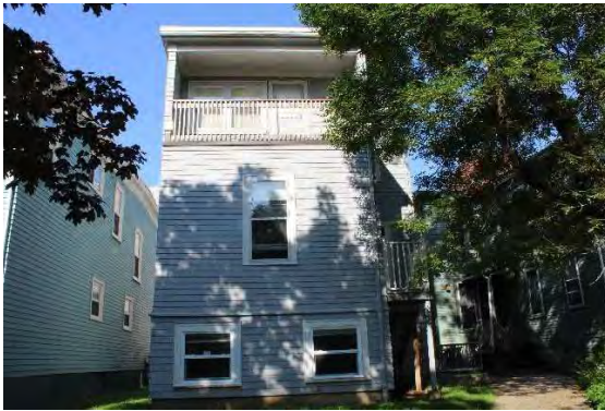
Photo 9: Second storey porch on rear (east) façade
