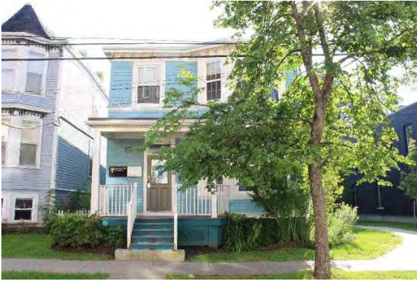
Photo 1: 1435 Seymour Street, looking east
