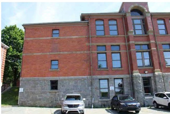
Photo 27: View of the addition (left) and original building (right) on the structure's rear (southwest) façade, looking northeast
