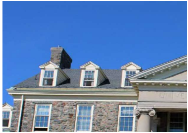
Photo 2: Representative view of roof, chimney, and dormers, looking west
