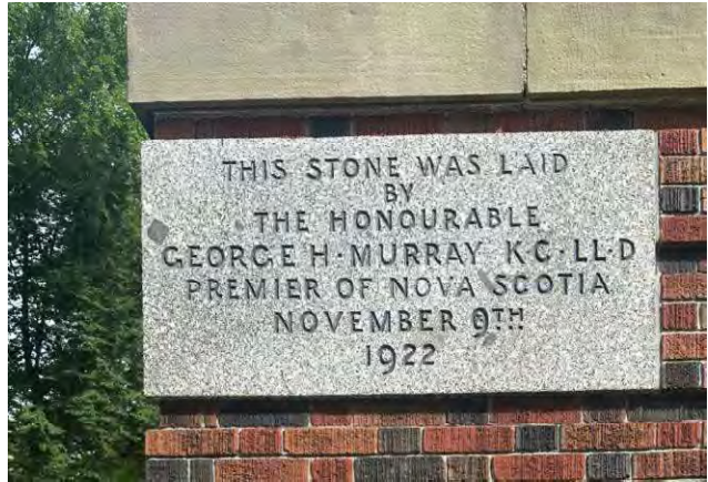
Photo 11: Cornerstone, looking north
