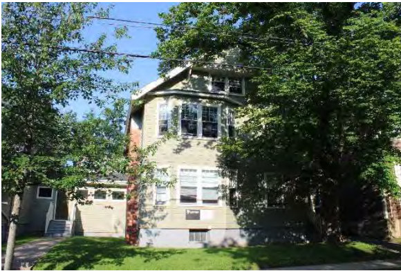
Photo 9: General view of residence, looking west
