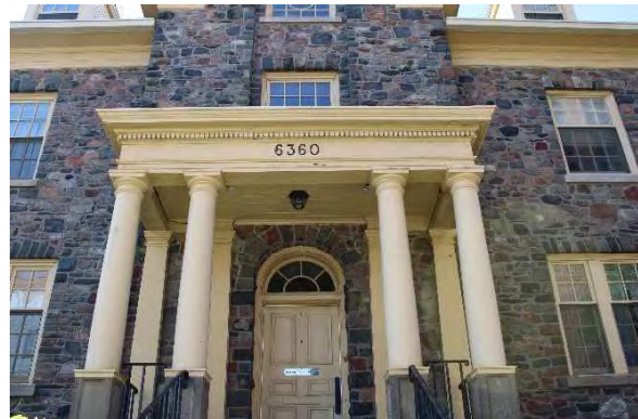
Photo 20: Portico, looking south (HRM 2023b)
