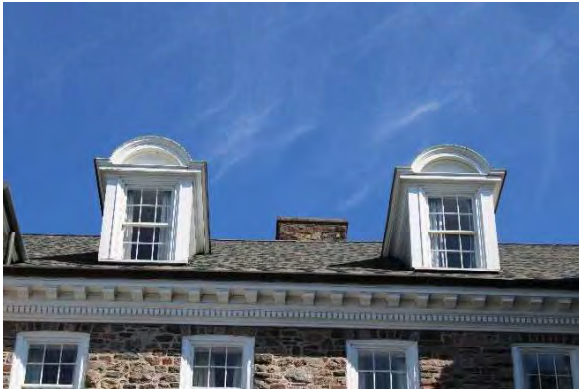
Photo 3: Arched dormers, looking north
