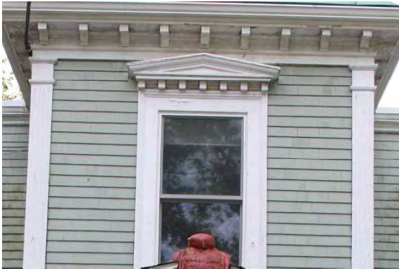
Photo 8: Classically inspired window surround, looking south
