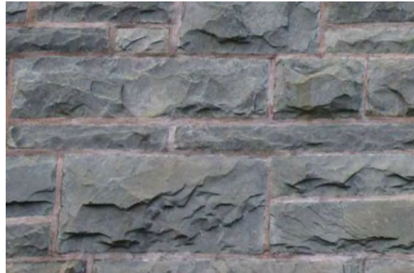
Photo 13: Dressed stone cladding, looking south
