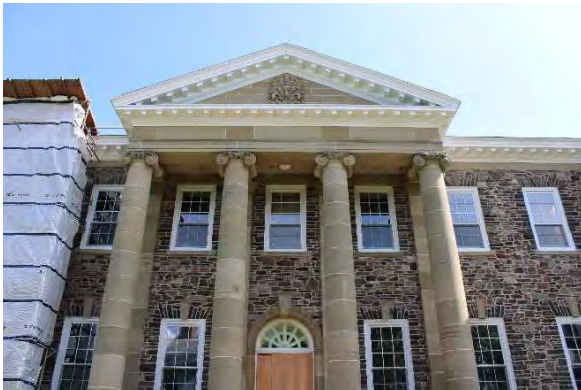
Photo 5: Projecting pediment over main entrance, looking south
