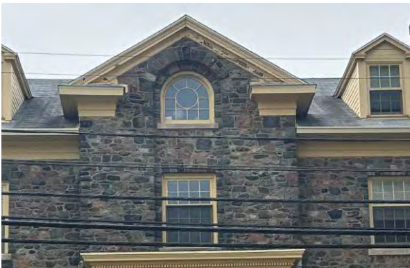
Photo 19: Centre bay, looking south (HRM 2023b)
