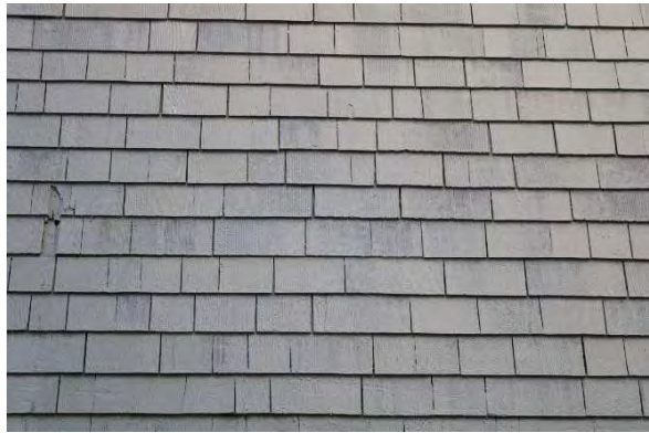
Photo 4: Wood shingle exterior, looking east
