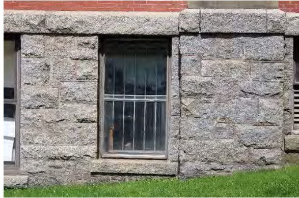
Photo 26: Cut stone foundation, looking northwest
