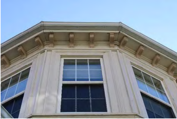
Photo 3: Bracket detailing on roofline
