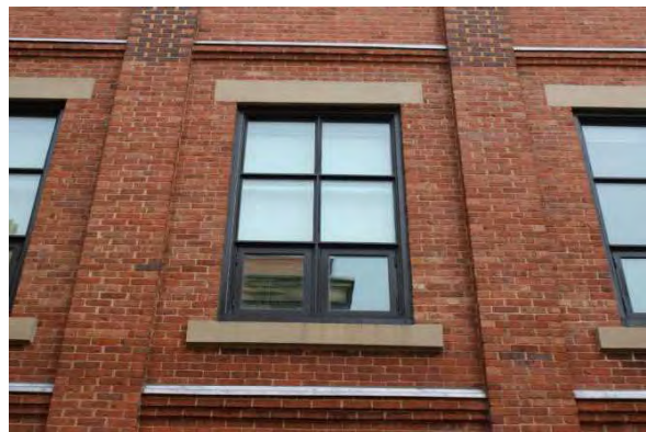
Photo 8: Pilasters, looking east
