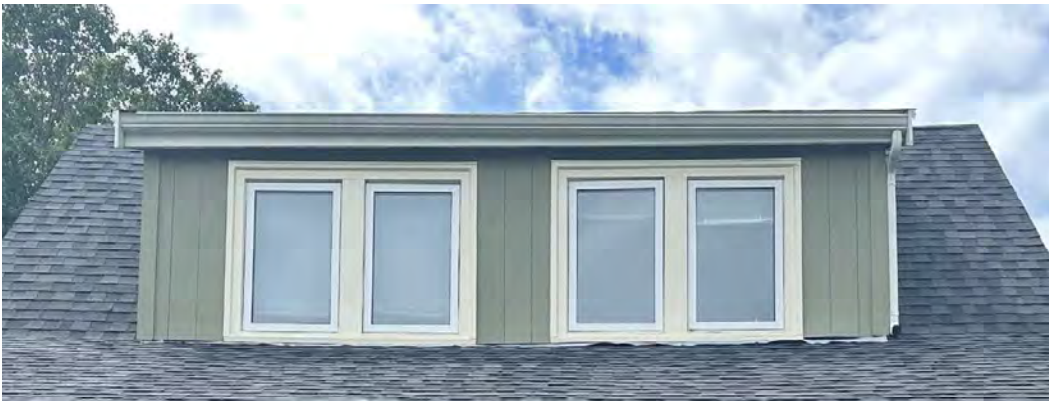
Photo 3: Shed roof dormer, looking west (HRM 2023b)
