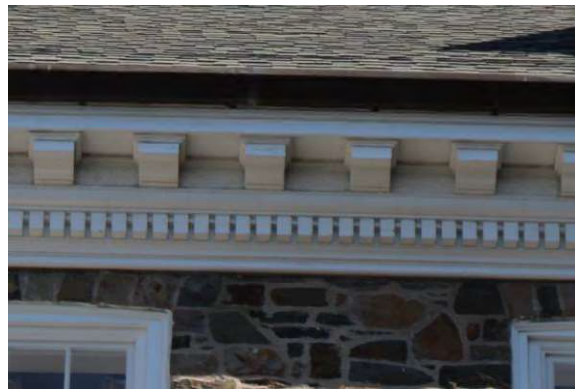
Photo 6: Cornice, looking north
