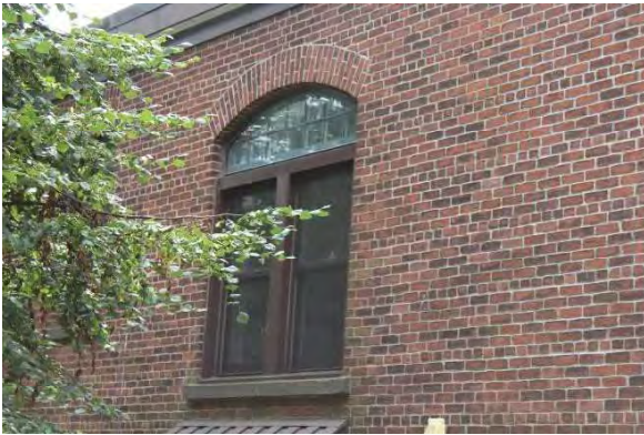
Photo 16: Arched window with wooden mullions, looking southeast
