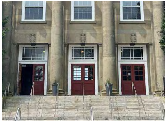
Photo 10: Entrance doors, looking west
