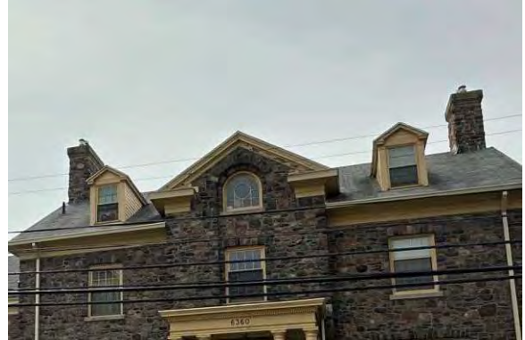
Photo 16: Side gable roof, dormers, and chimneys, looking south (HRM 2023b)
