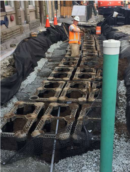
Soil cell installation along Argyle street.
