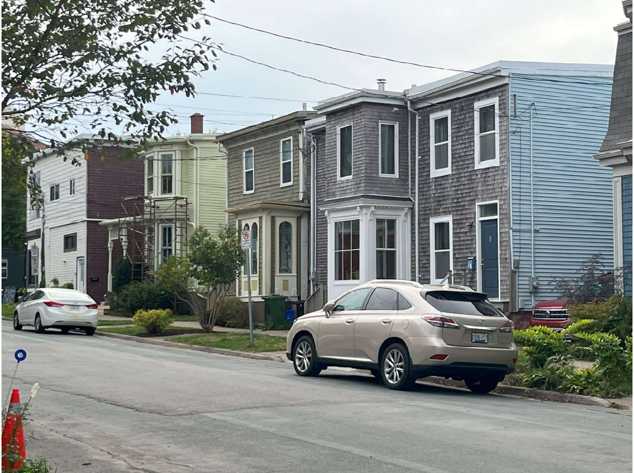
Figure 22: Photograph looking west up Harris Street from Maynard, showing similar two-storey Halifax Box styles with covered porche entryways (Staff visit, September 19 th , 2024)
