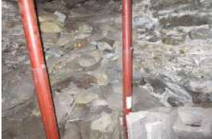
Figure 14: Image of house foundation from interior (Provided by applicant)
