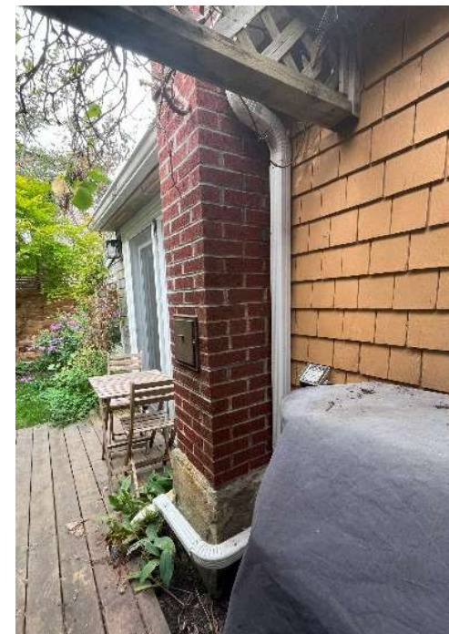
Rear addition with chimney
