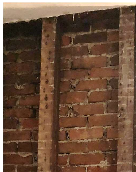
Ballon-like construction evident in spacing of studs with nail marks
