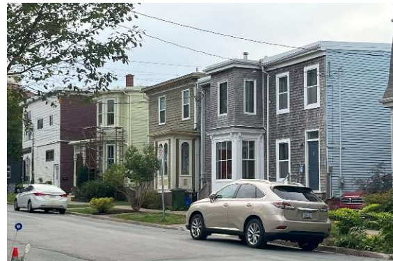
East side of Maynard Street, north of the subject property
