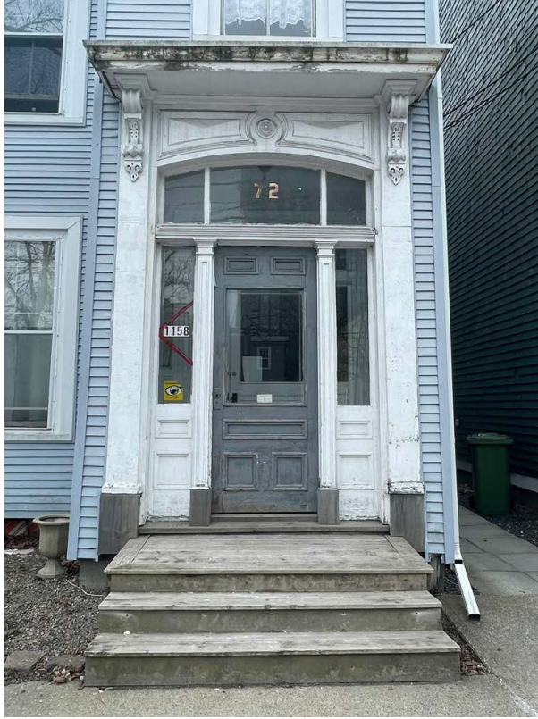
Figure 15: Entry door with transom, side lights, corbels and decorative panels, July 2025
