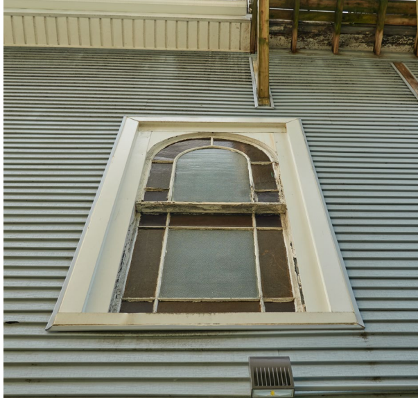
Figure 17: Arched-top window with stained glass on the north elevation, July 2025
