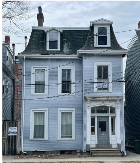
Figure 1: 1158 South Park Street, July 2025
