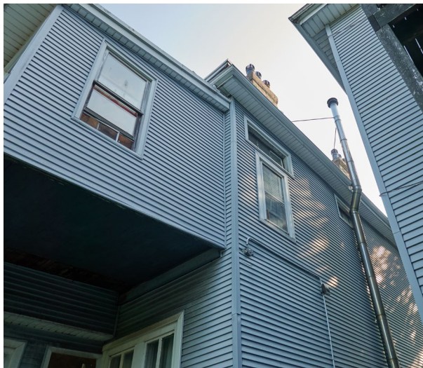
Figure 22: Rear addition and new window opening, July 2025
