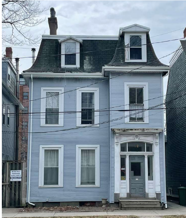
Figure 1: 1158 South Park Street, July 2025
