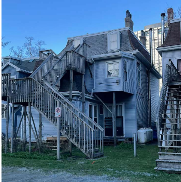
Figure 13: Southwest corner, July 2025
