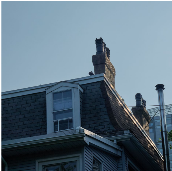
Figure 16: Brick chimneys and a dormer on the mansard roof, July 2025
