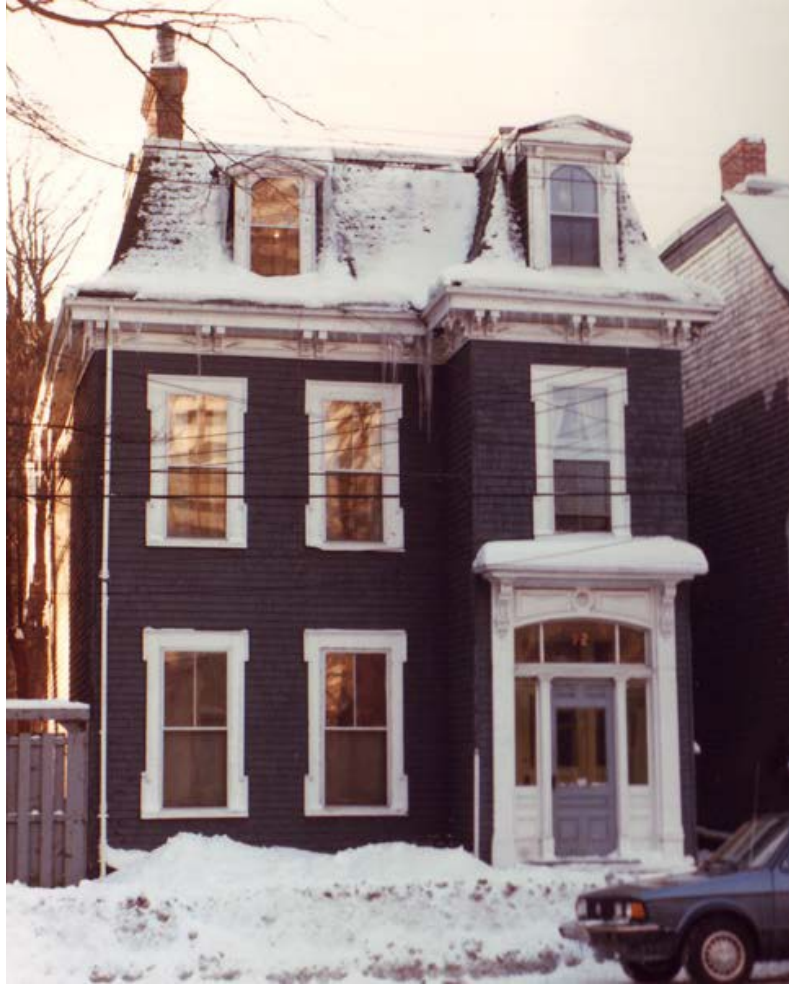
Figure 20: Historical photo (c. 1985) indicates the absence of the moulded window trims, eave brackets, wood siding and dormer details
