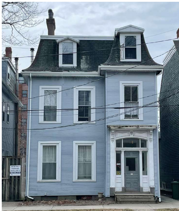
Figure 12: East elevation, July 2025
