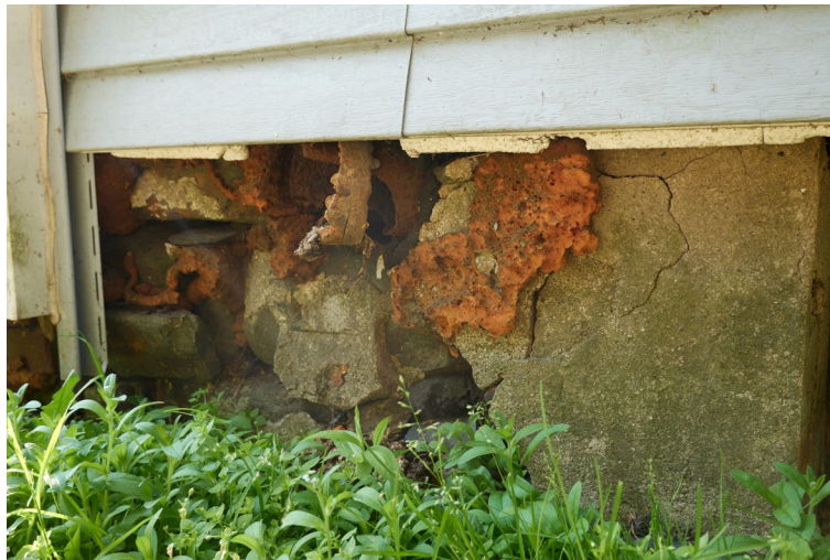
Figure 11: Stone foundation of the subject property, July 2025
