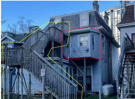
Rear Addition, Stairs & Decks
