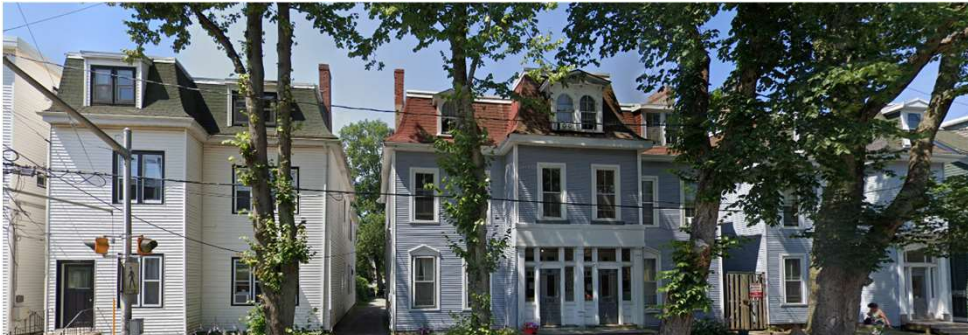
Second Empire Homes at 1146, 1150-1152, and 1158 South Park St (subject property); Constructed by McNab
