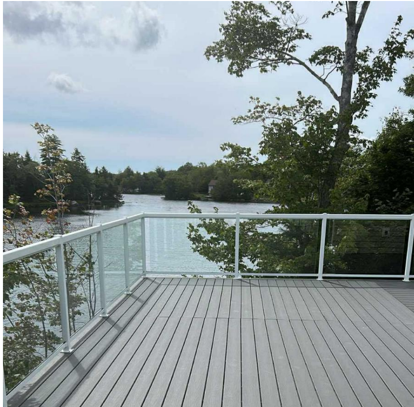
Figure 1: Banquet hall balcony, facing South.
