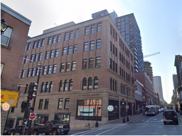
Figure 9: T. Eaton Maritime Store, Halifax, NS, designed by Sydney Perry Dumaresq
