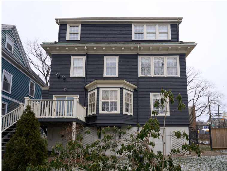
Figure 14: West elevation (March 2025)
