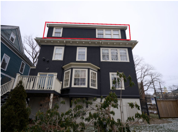
Figure 20: Shed dormer on west elevation (highlighted in red box), added in the 1990s with matching windows and cladding (March 2025)
