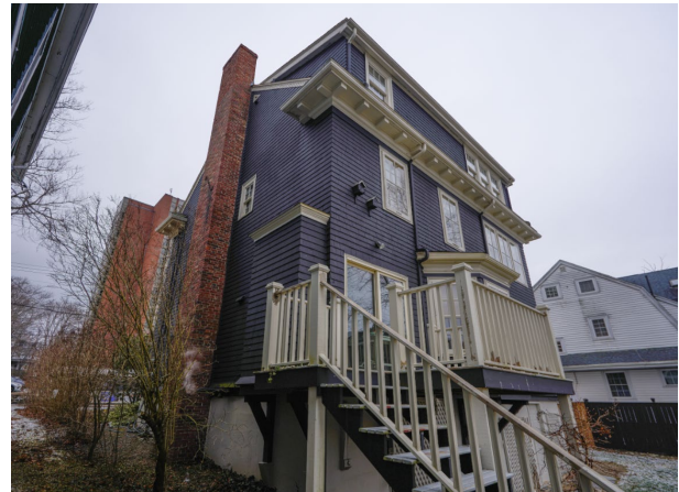
Figure 21: The utility projection, back entrance, and deck were added recently (March 2025)
