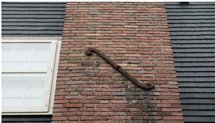
Figure 18: Anchor plate on the brick chimney (March 2025)
