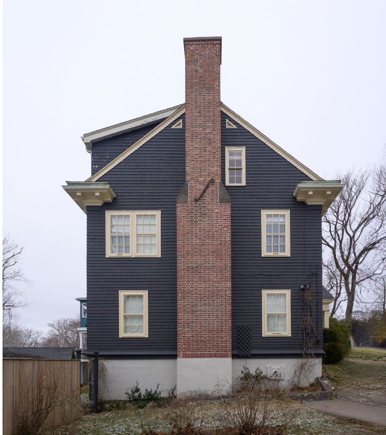
Figure 15: South elevation (March 2025)
