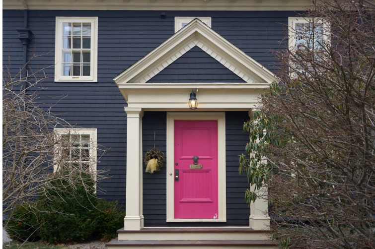
Figure 17: Central entry porch with pediment, classical pilasters and trims (March 2025)
