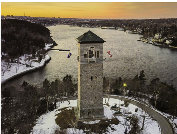
Figure 7: Dingle Tower, Halifax, NS, designed by Sydney Perry Dumaresq and Andrew R. Cobb
