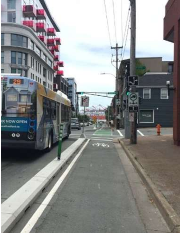
Tactical Protected Bike Lane Typical Cost: ~$1,100/m
