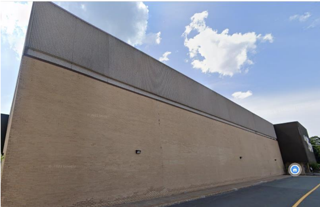
Existing blank walls at the Mic Mac Mall
