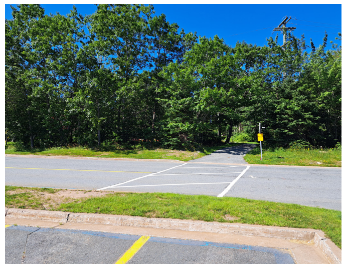
On-site crosswalk ends at inaccessible curb (HRM Planned Growth)
