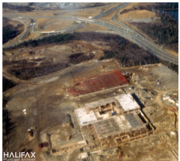
Mic Mac Mall Construction, 1972 (Halifax Municipal Archives)
