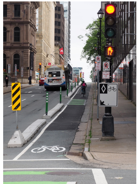
Hollis Street Protected Bike Lane
