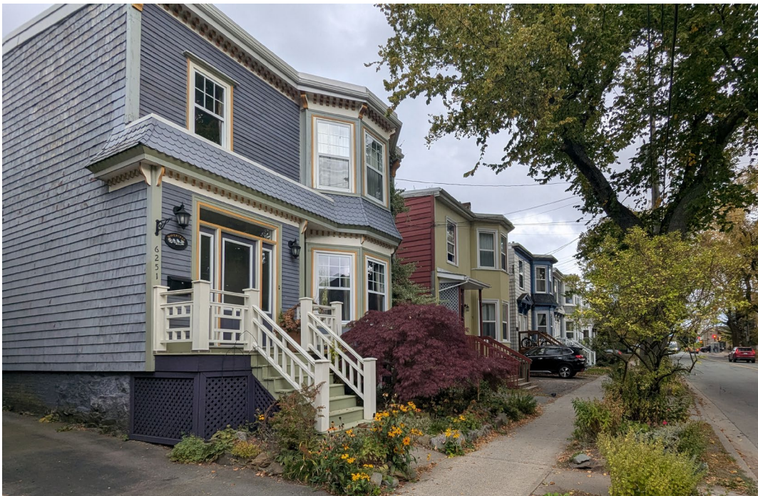
Figure 32: Photograph of the north side of North Street between Windsor and Almon Streets, originally built and sold by Rosborough & Thomas (Staff photo, October 16th, 2025).
