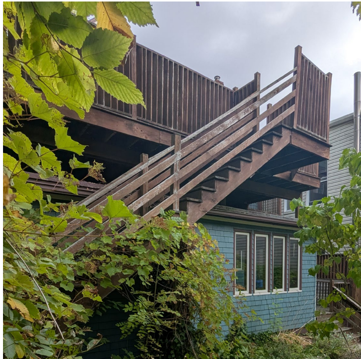
Figure 21: Photograph of the rear of the subject property showing rear deck and addition (Staff photo, October 16th, 2025).
