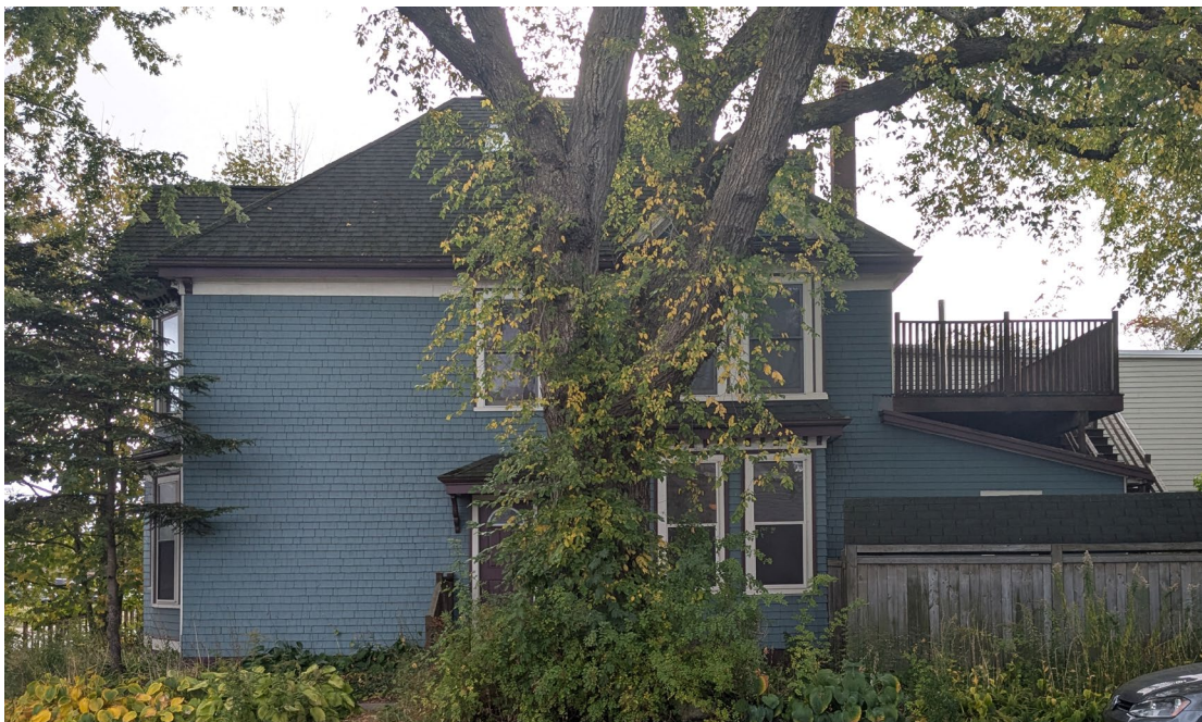
Figure 19: Subject property from Seaforth Street, showing north facing facade (Staff photo, October 16th, 2025).
