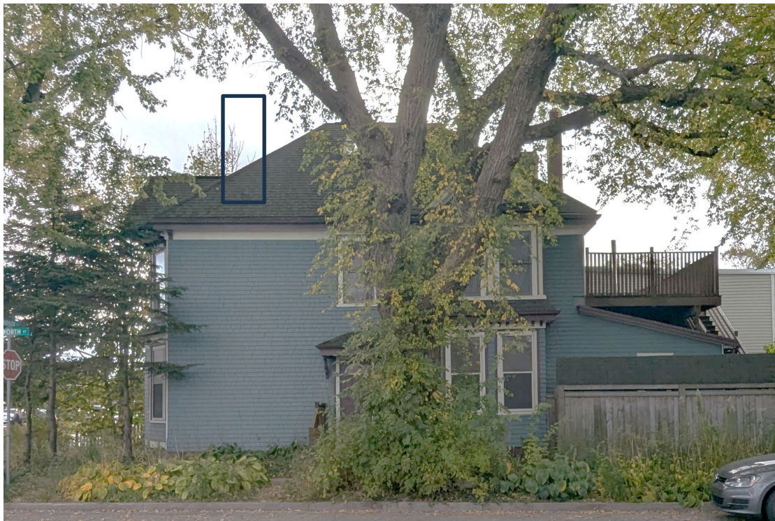
Figure 26: Photograph of subject property's north facing elevation from Seaforth Street, with area where former north east chimney stood highlighted (Staff photo, October 16th, 2025).
