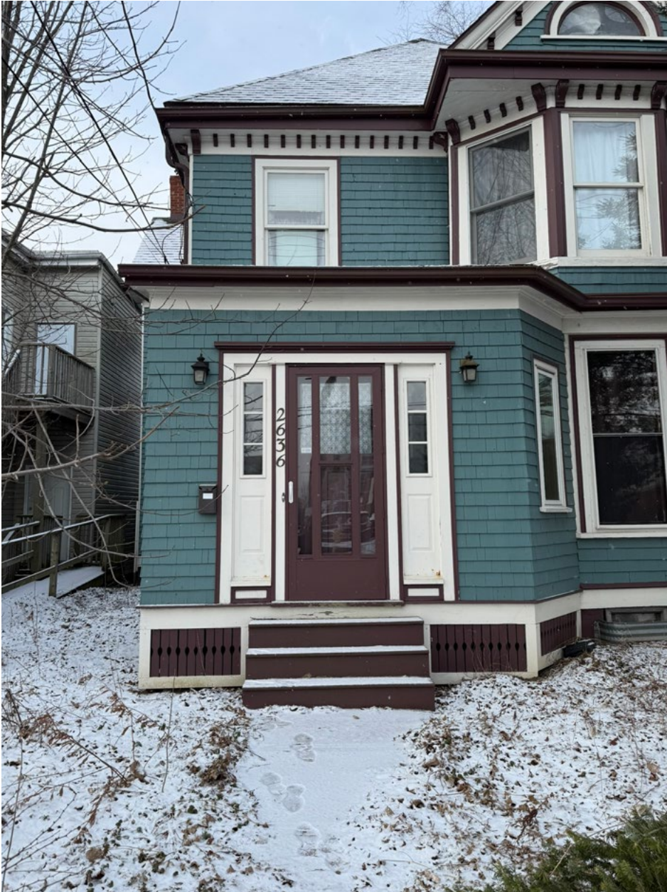
Front elevation of the enclosed front porch
