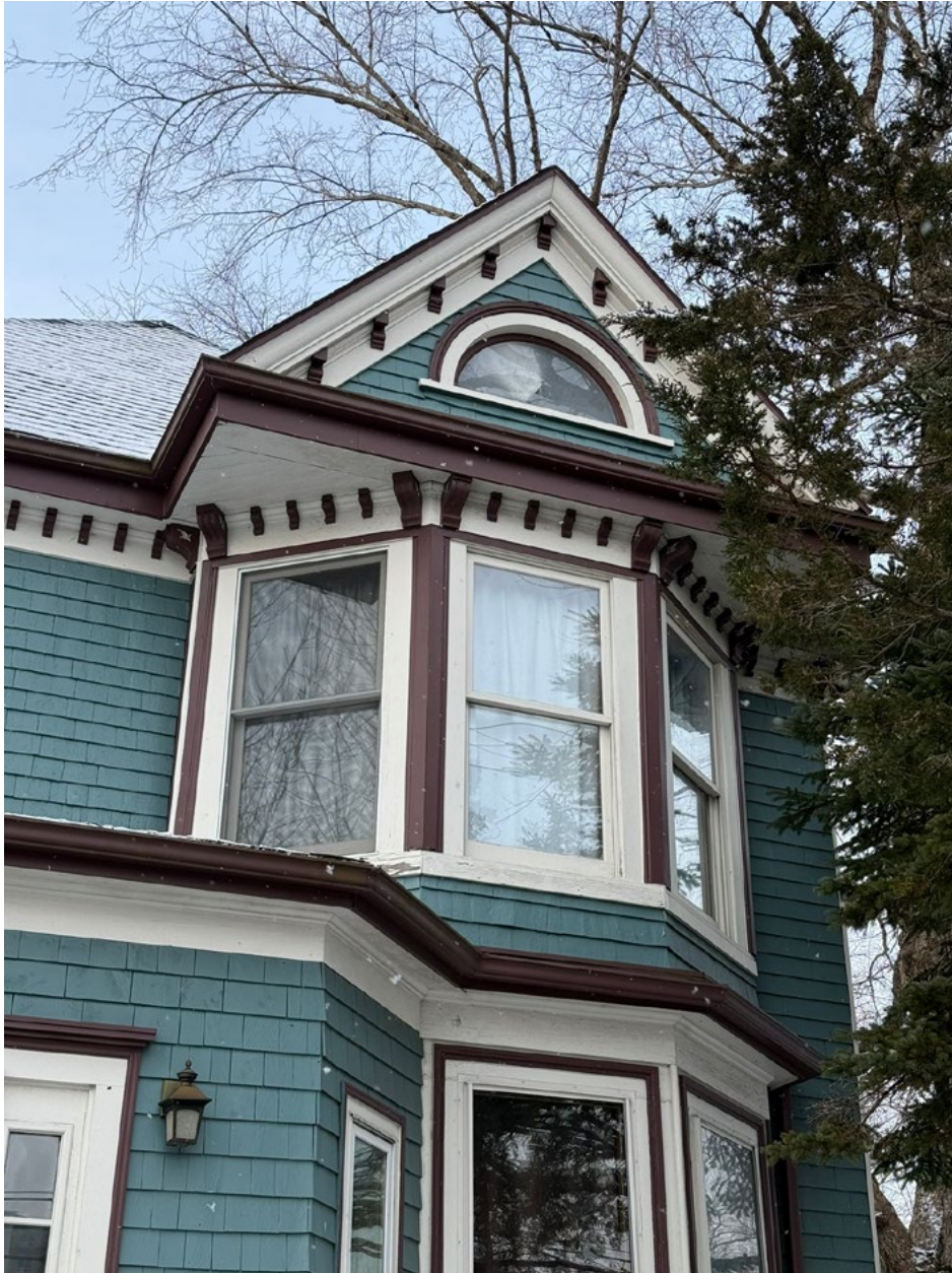
Bay window on front (North) facade
