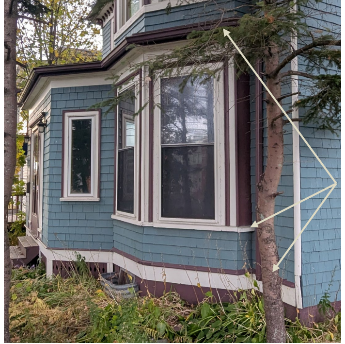
Figure 23: Photograph of first storey bay windows and enclosed porch, current day with wood trim highlighted (Staff photo, October 16th, 2025).
