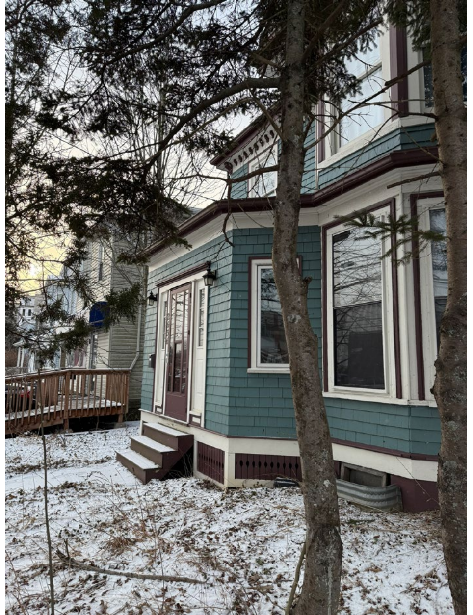
Side elevation of the enclosed front porch
