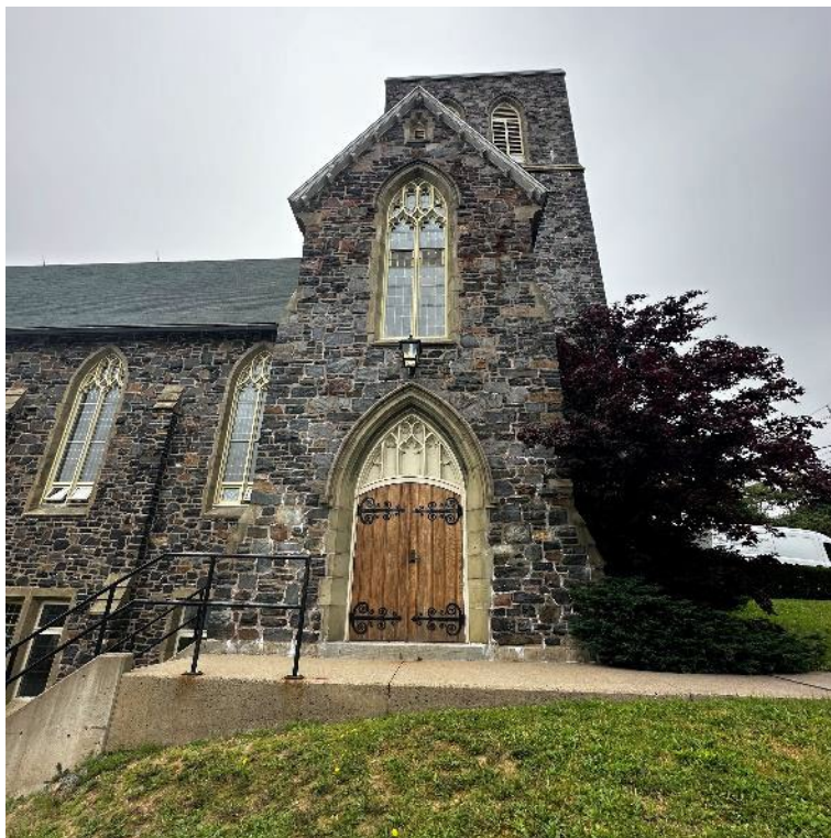
Figure 25: Gable with an entry door and Gothic window (July 17, 2024)
