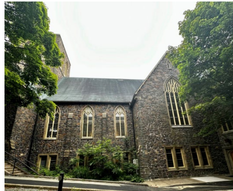
Figure 3: North elevation, July 2024
