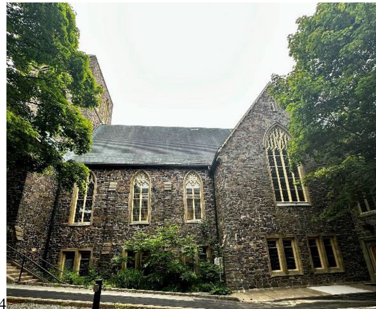
Figure 23: North elevation of original portion (July 17, 2024)
