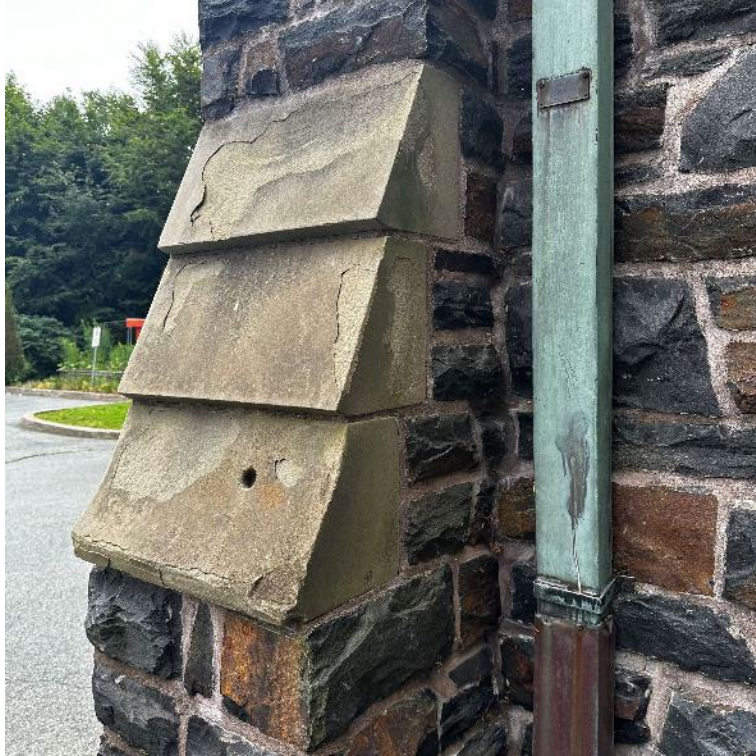
Figure 26: Detail of a stone buttress and copper downspouts (July 17, 2024)
