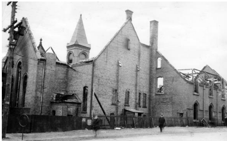
Figure 1: Former First Baptist Church on Queen Street, Halifax, depicting fire aftermath 2
