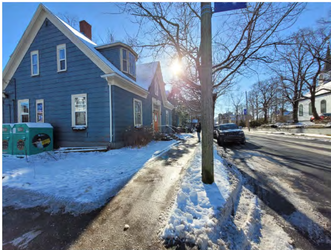
Figure 21b: Context of 86 Ochterloney Street (front, looking southwest along Ochterloney Street) – neighbouring Christ Church on the far right
