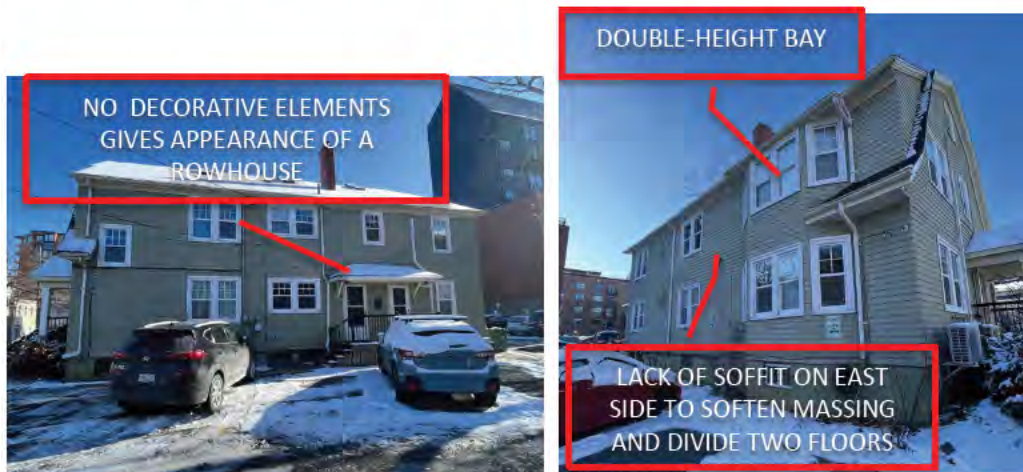
Figure 36b: Side components of 43-45 Dundas Street that detract from the style and overall design of a Dutch Colonial Revival house.
