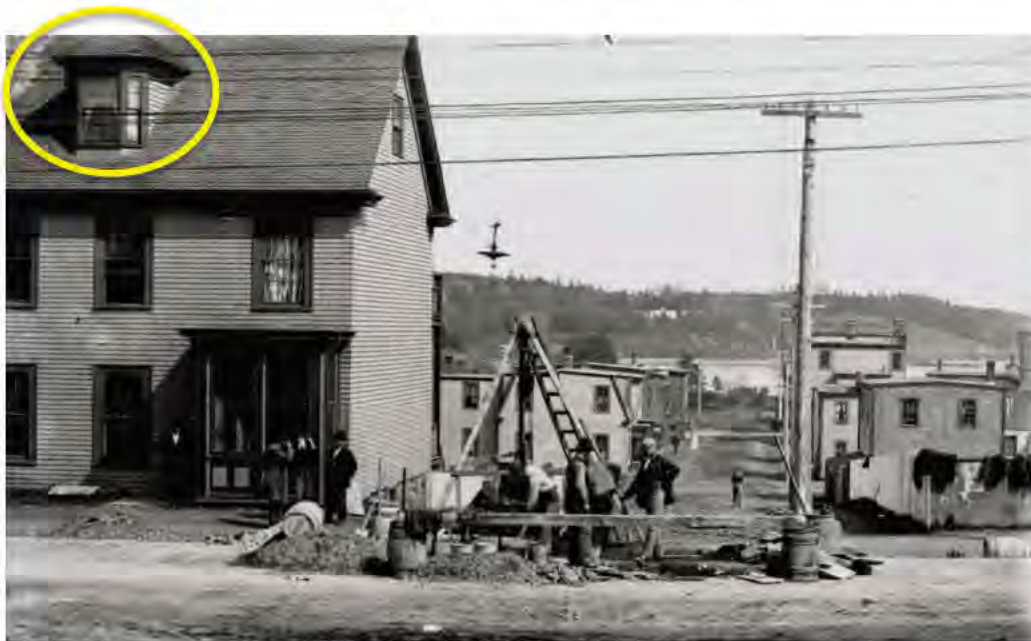
Figure 10: Victoria at Ochterloney – a house featuring the same Scottish dormers as the George and Mary Shiels Residence
