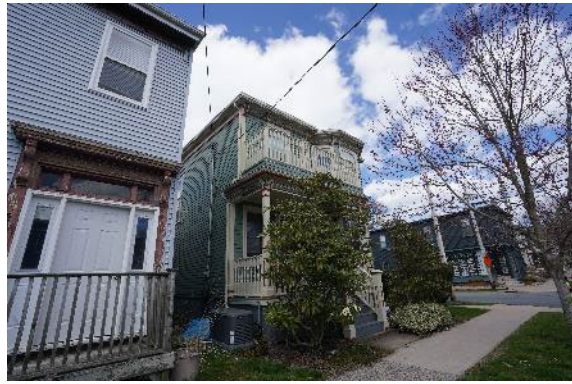
Figure 10: West Elevation (April 26, 2024)
