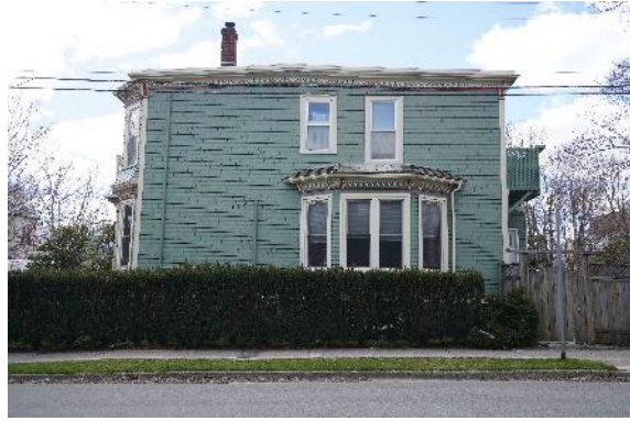
Figure 8: East Elevation (April 26, 2024)
