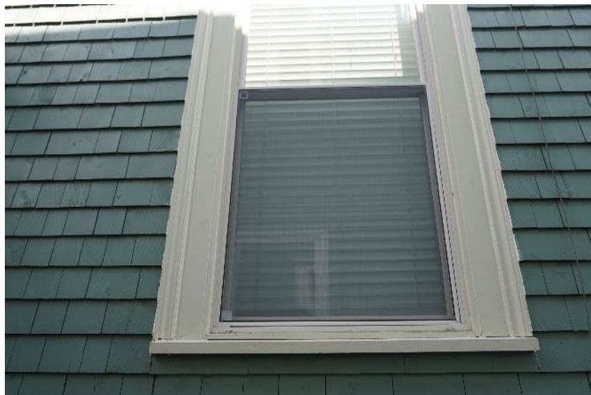
Figure 17: The sashes have been replaced with vinyl, while the frame retains its original wooden structure (April 26, 2024)
