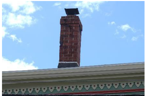
Figure 16: Brick Chimney (April 26, 2024)
