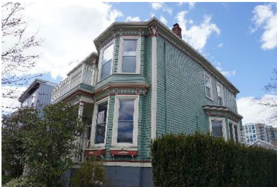
Figure 11: Two-storey bay window on the south elevation, composed of two sets of three, one-over-one wood-framed windows with piers, running trims and corbel detailing (April 26, 2024)
