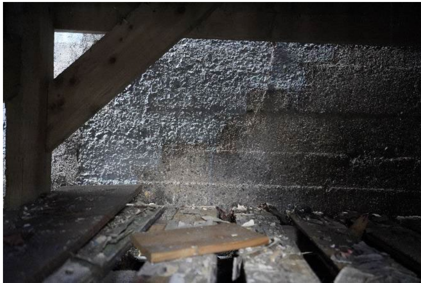
Figure 5: Poured concrete basement of the subject property (April 26, 2024)
