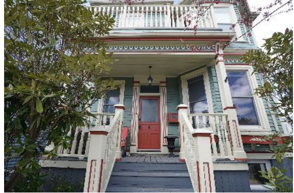
Figure 14: Porch with railings on the first floor and second floor, square columns, running trims, and corbels (April 26, 2024)
