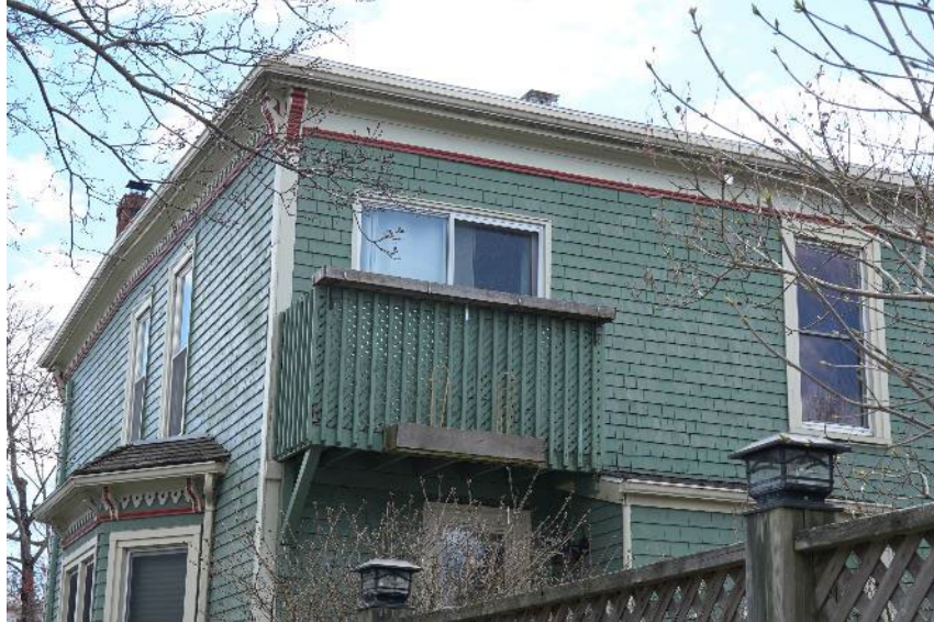
Figure 20: Added Balcony At The Rear (April 26, 2024)
