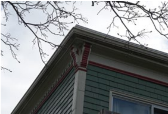
Figure 15: Detailings of the corner boards, corbels, and fleur running trims (April 26, 2024)
