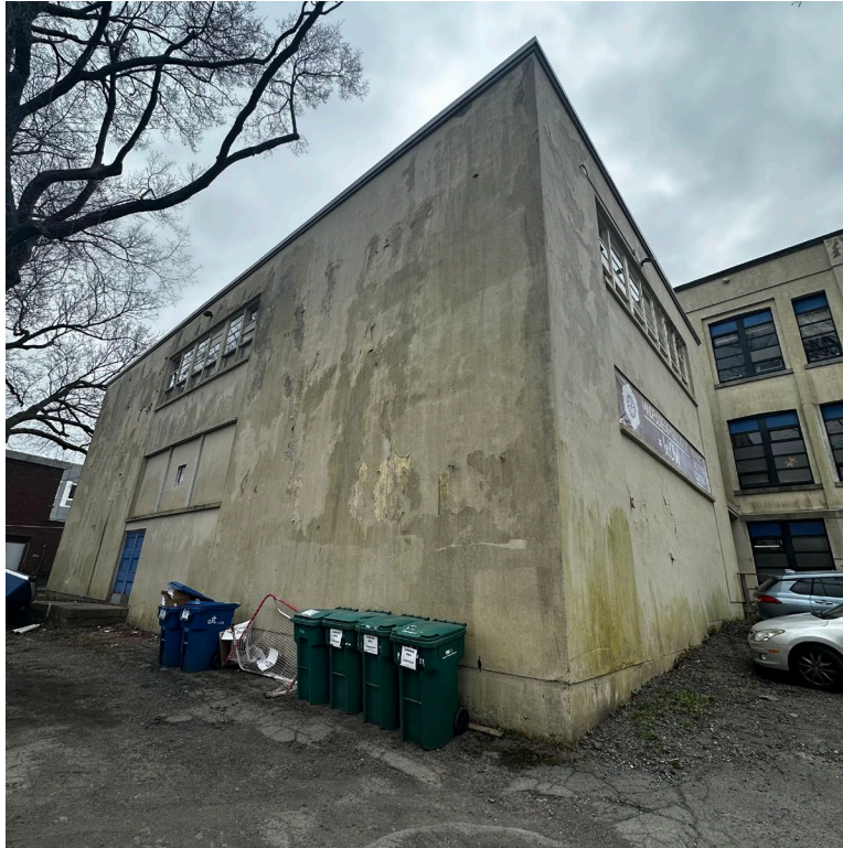
Figure 17: North and east elevation of the rear addition (May 1, 2024)
