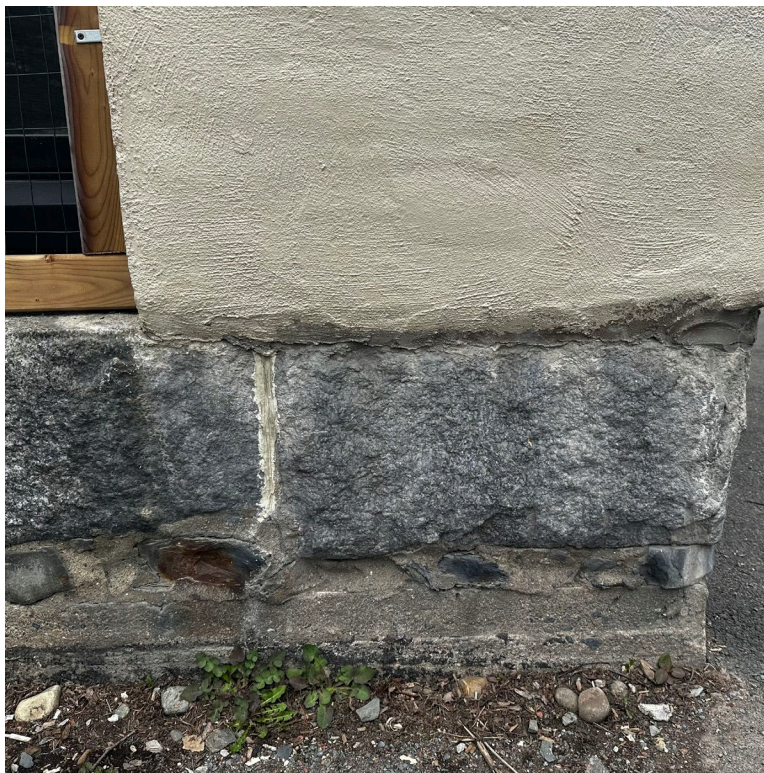
Figure 18: Stucco cladding and granite and rubblestone foundation (May 1, 2024)
