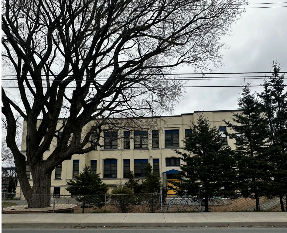
Figure 14: West elevation of the original portion of 5450 Russell Street (May 1, 2024)
