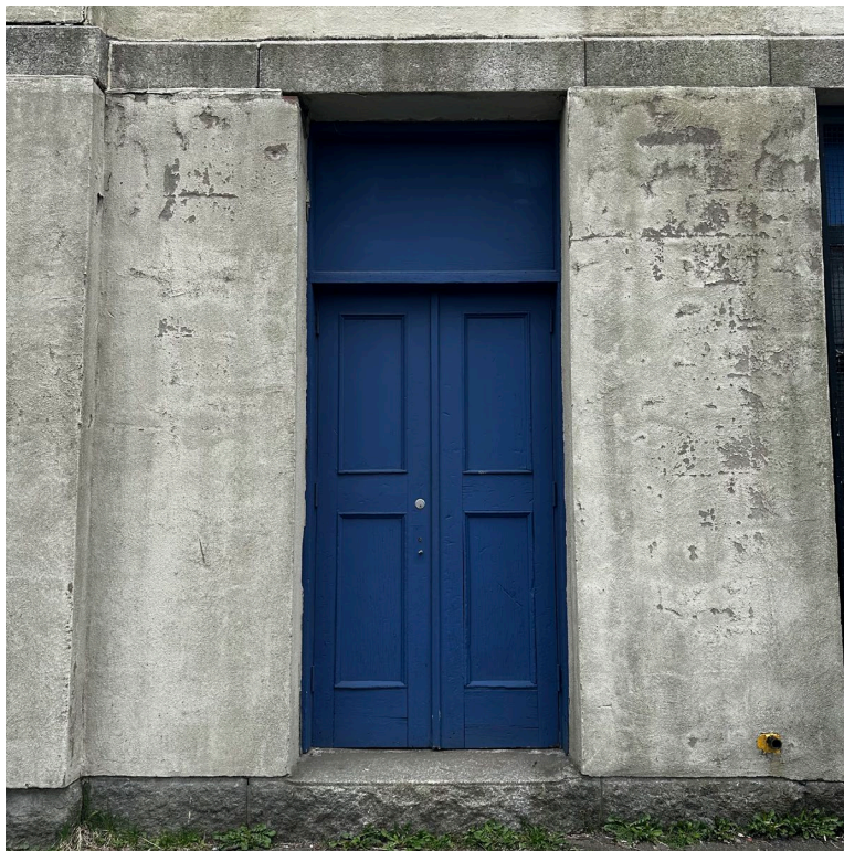
Figure 22: Double-leaf wood entrance with blinded transom on the east elevation (May 1, 2024)
