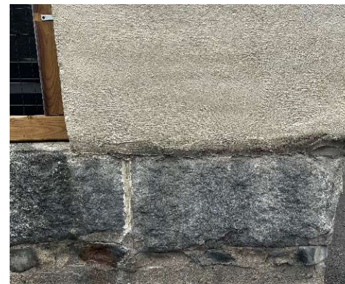
Stucco parging and granite block and stone foundation (May 2024)
