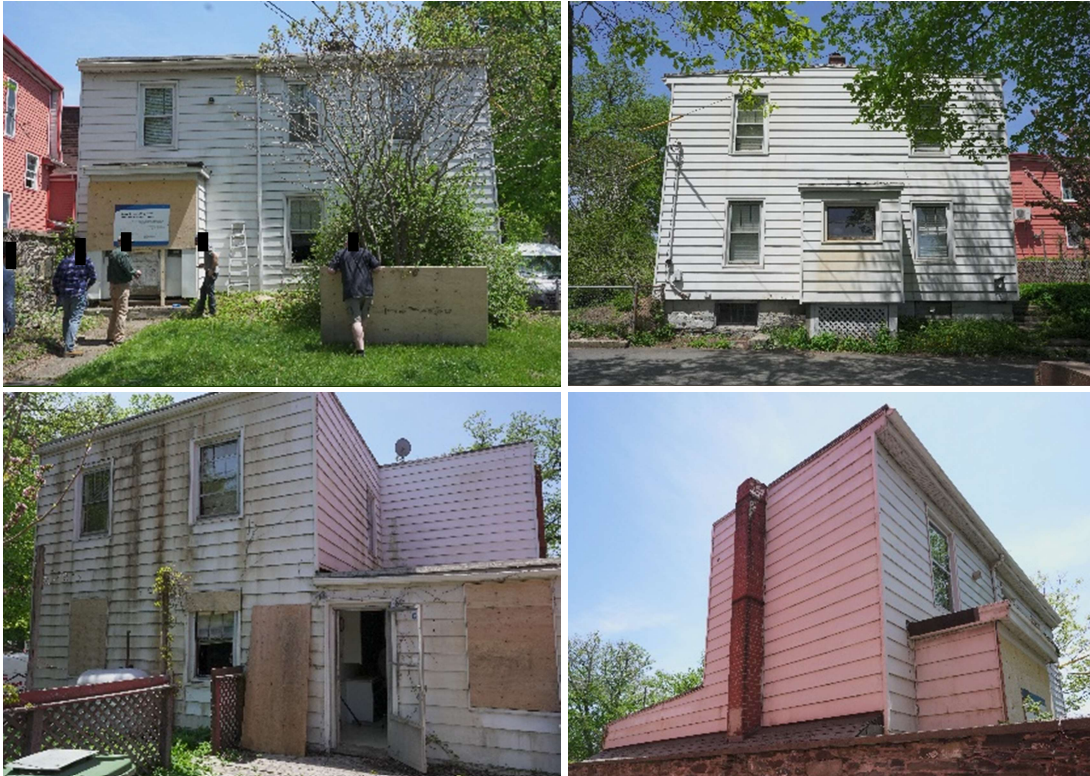
Elevation photos taken during site visit (May 31, 2023)
