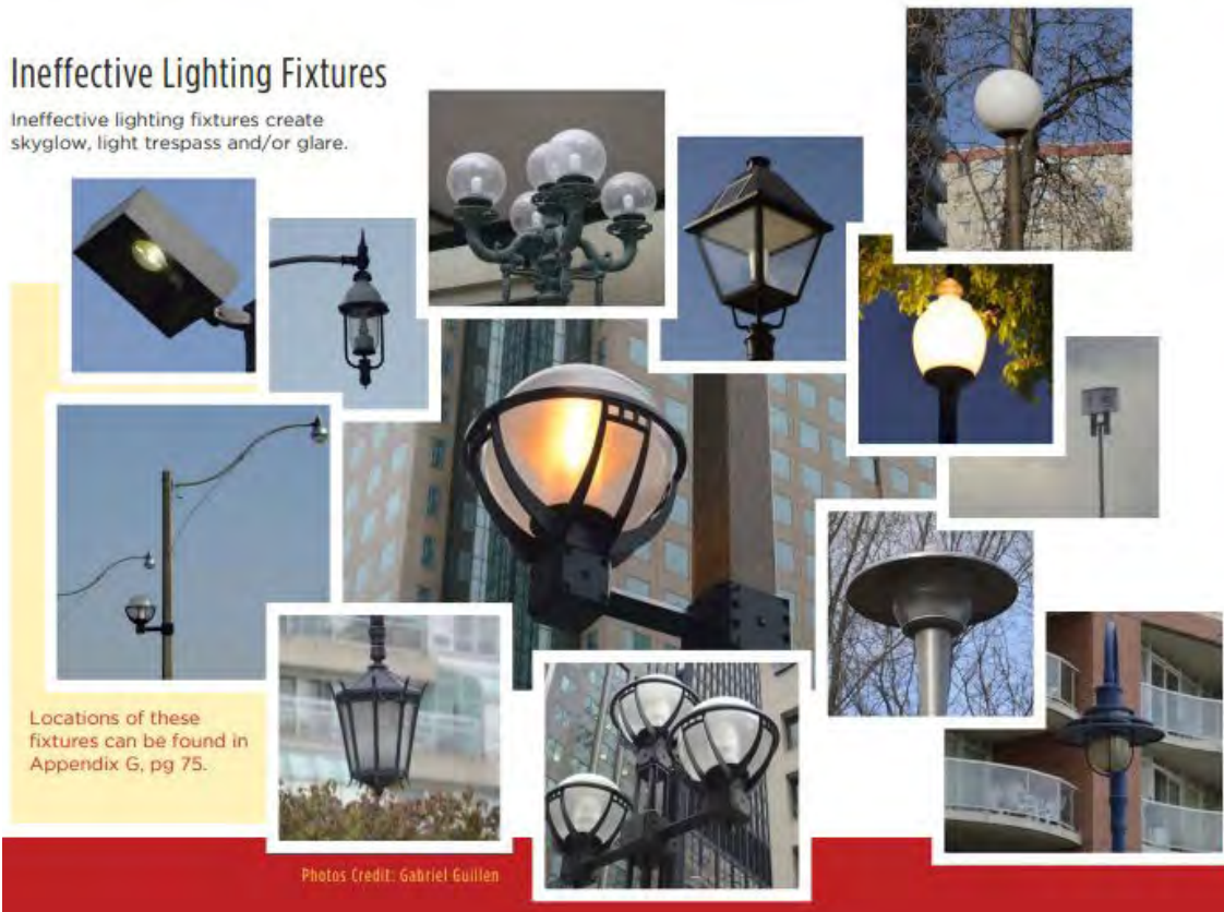
Figure B1: Ineffective Lighting Fixtures that create skyglow, light trespass, and glare (City of Toronto, 2017).
