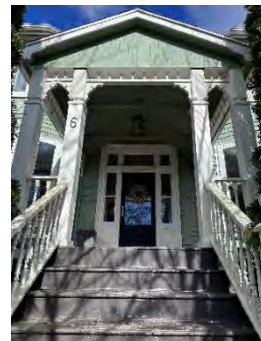
Figure 2: The porch and entry door of the subject building, July 2024
