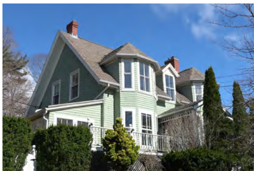
Figure 1: 6 First Avenue, April 2024
