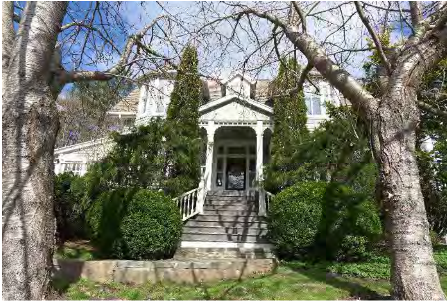
Figure 9: East elevation (Staff photo, April 18, 2024)
