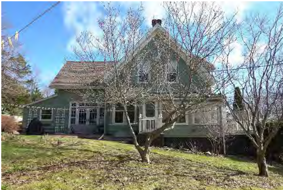
Figure 12: South elevation (Staff photo, April 18, 2024)
