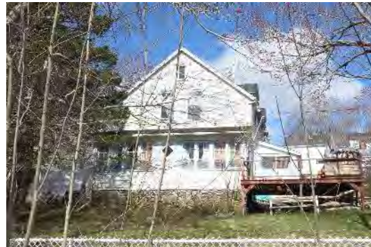
Figure 27: 9 Division Street (Staff photo, April 18, 2024)
