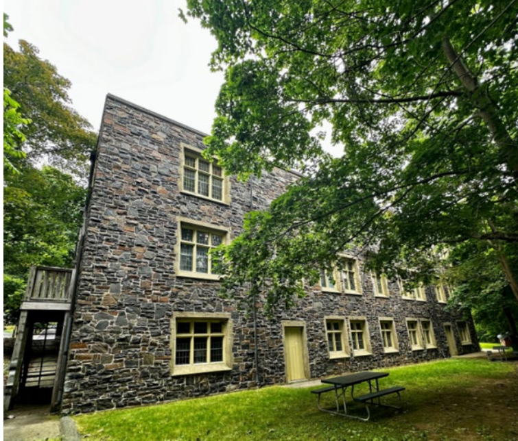
Figure 24: West elevation (Christian Education Wing addition. July 17, 2024)
