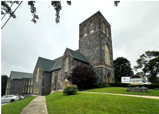
Figure 2: South and east elevations, July 2024
